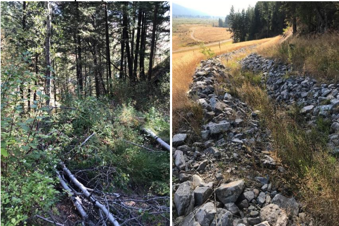
Left: Eroded area above Tunnel Pond Repository; Right: Vegetation in perimeter ditch as a result of eroded area above Tunnel Pond Repository
