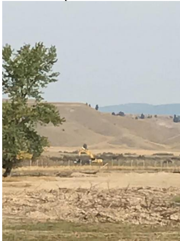
Figure H-12: Area with Remediation Underway
