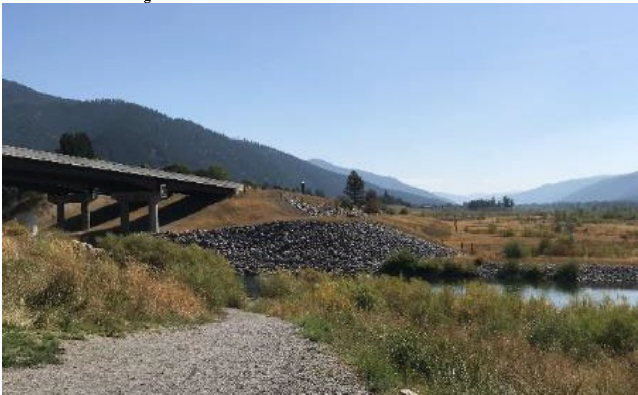
Figure H-4: Buttress Along Interstate 90
