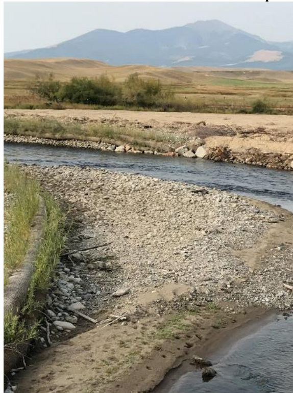
Figure H-15: Bank Stabilization on Clark Fork River with Sediment Deposition on Inside Curve
