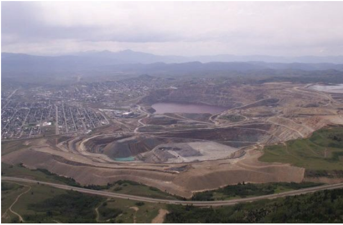
Picture of Butte and the Berkeley Pit in the mid-2000s (photo provided by Nikia Greene)
