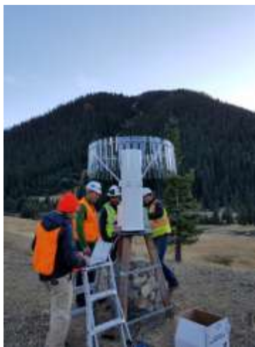
Photo 12: Gladstone ETI NOAH 2 precipitation gage installation.
