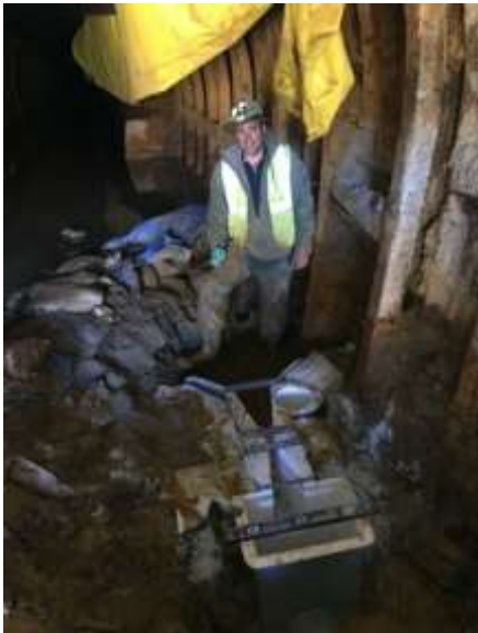
Photo 3: American Tunnel flume
