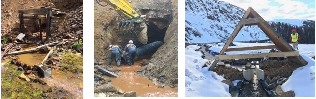
Photos 9-11: Blackhawk Mine portal stabilization and flume install with snow shed.
