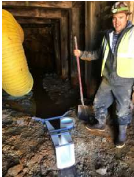
Photo 4: Mogul Mine flume installation
