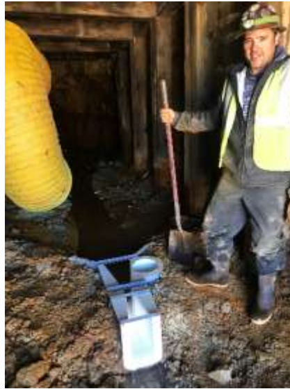
Installation of fiberglass Parshall flume at the Mogul mine portal, October 2018.
