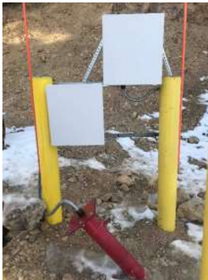
American Tunnel monitoring well (ATPZ_2) instrument installation, November 2019.
