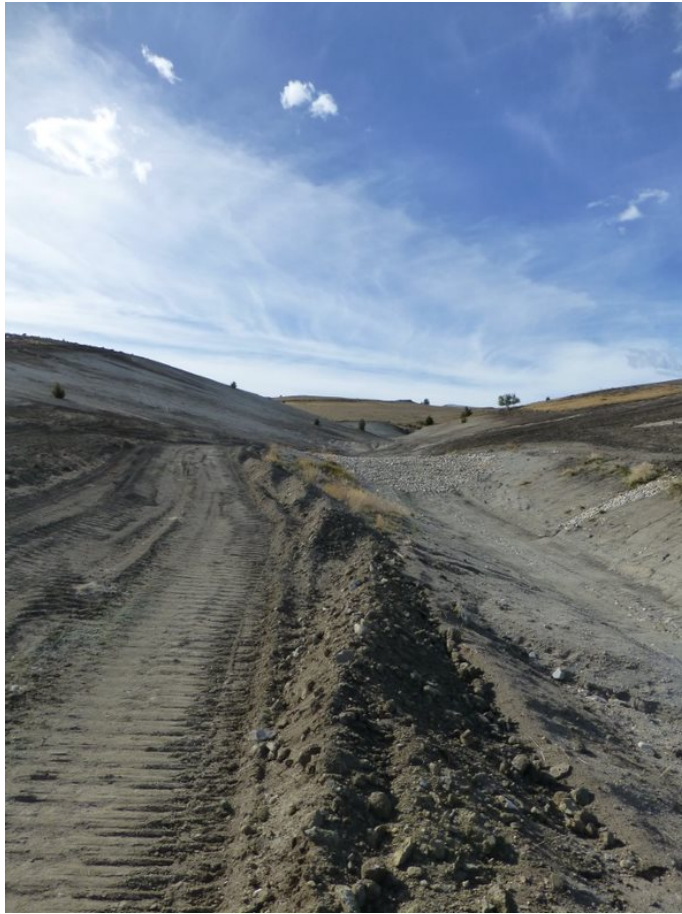
OU4: North Opportunity area showing check dam and stormwater channel
