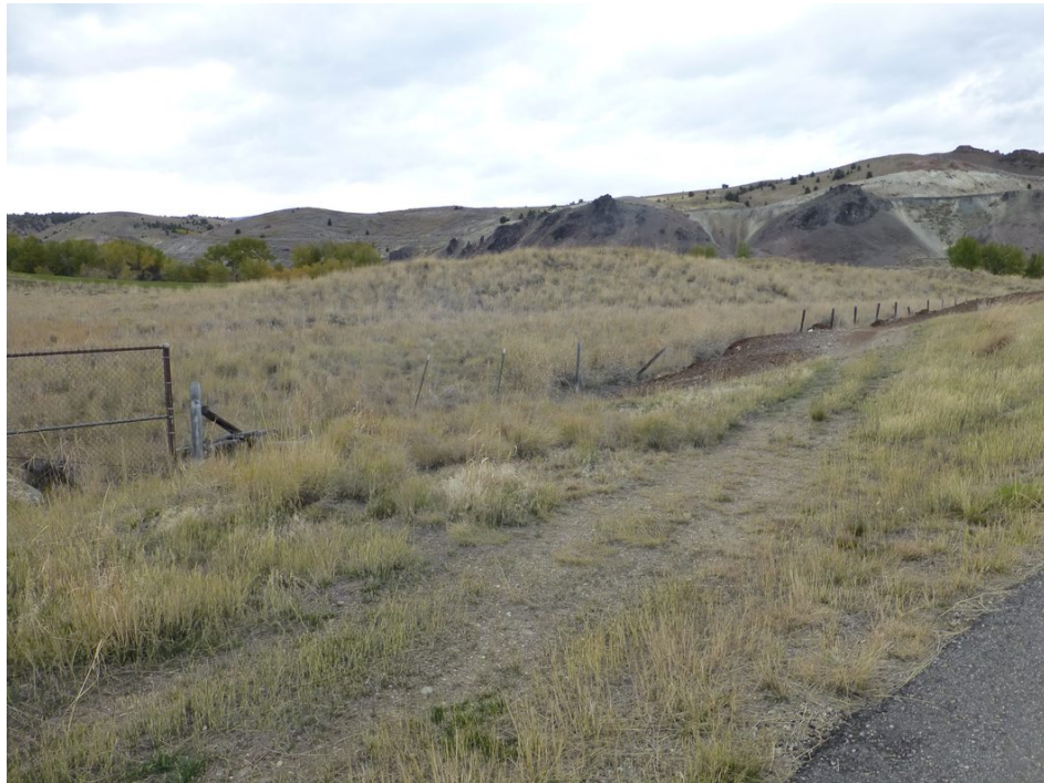
OU7: Damaged fence and vehicle/bike tracks between golf course and recreation trail
