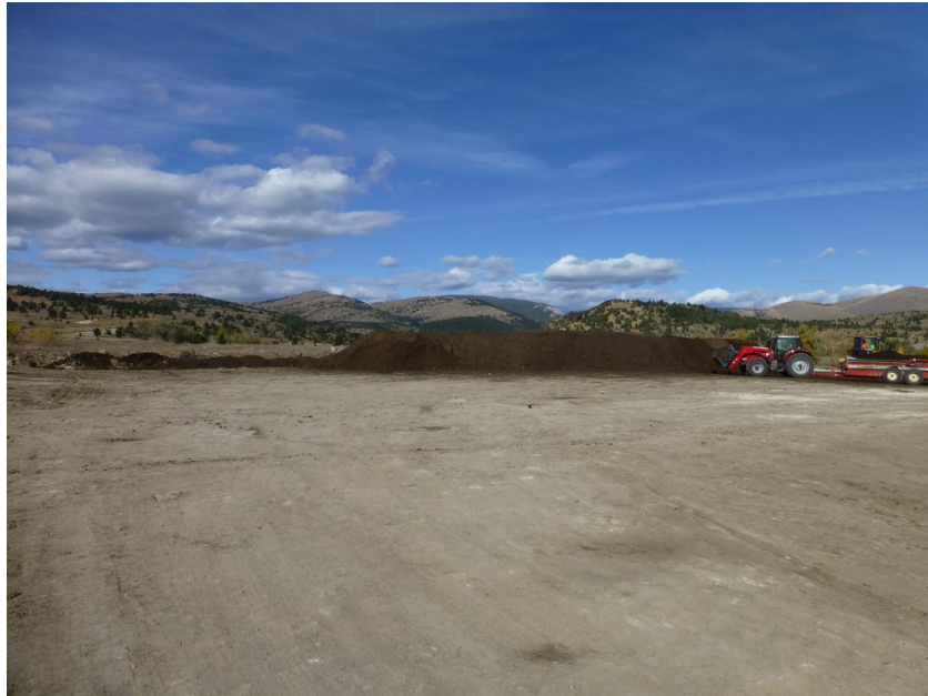
OU4: Organic soil amendments for reclamation of remediated areas
