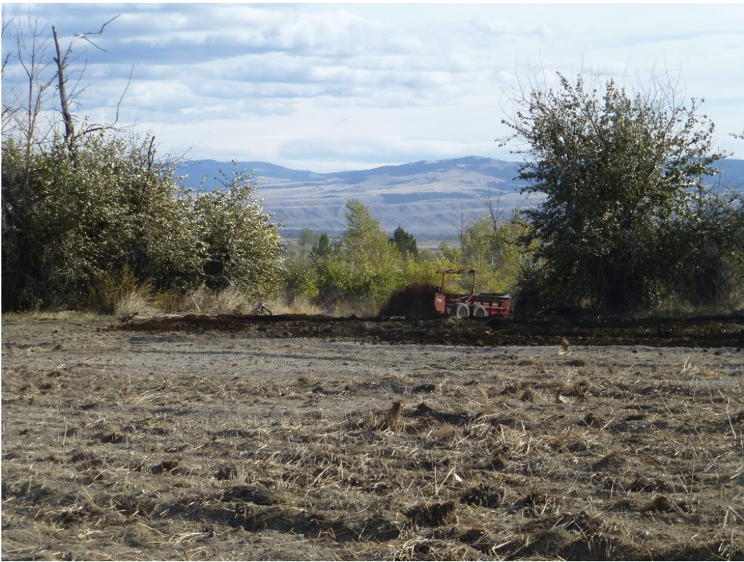
OU15: Stripped area ready for lime
