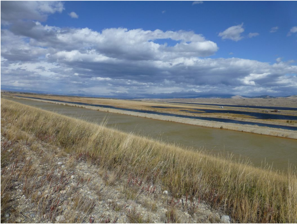
OU4: Groundwater and surface water management system
