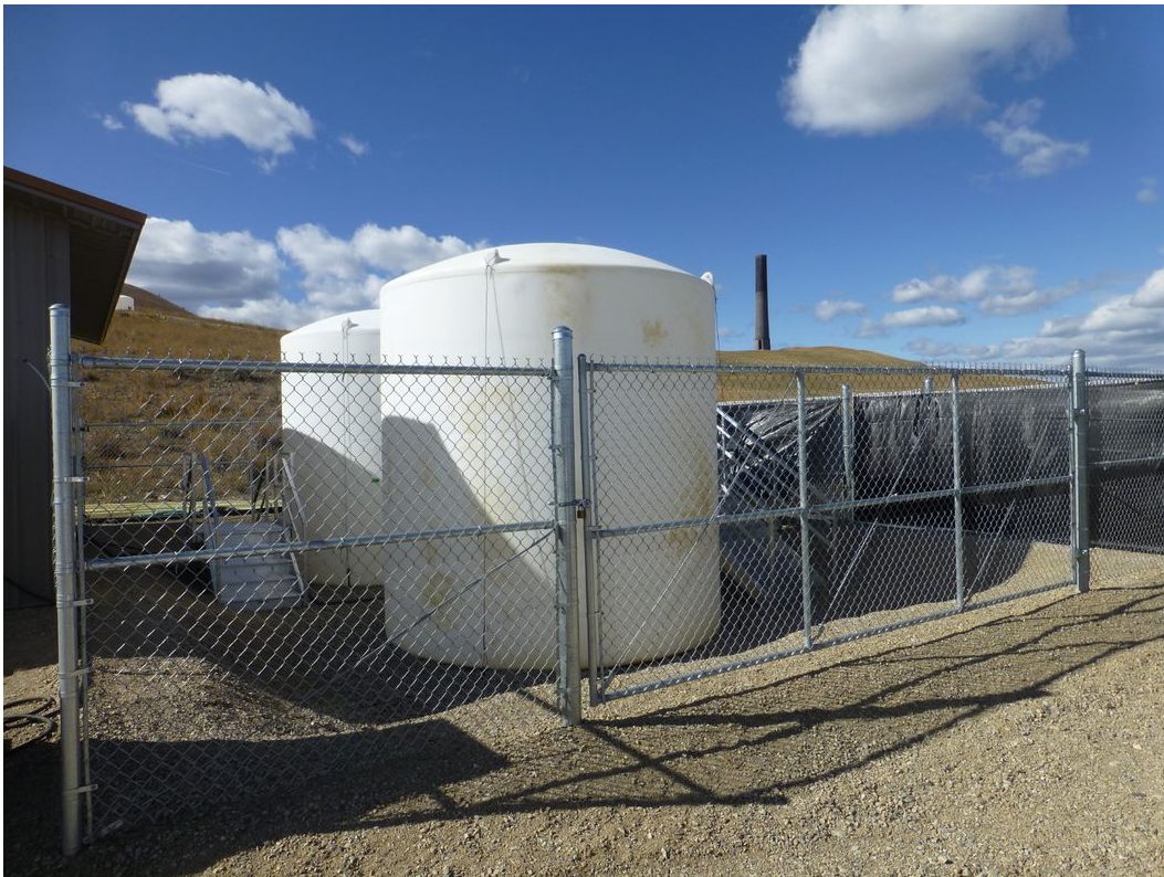
OU11: Flue Dust leachate collection and evaporation system located near smelter hill
