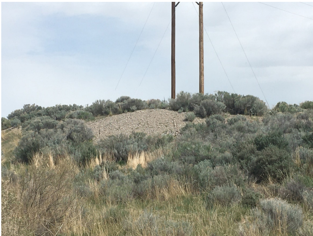
Photo 8: OU4 Established Vegetation and Intact Gravel Hill Covering Remaining Contamination
