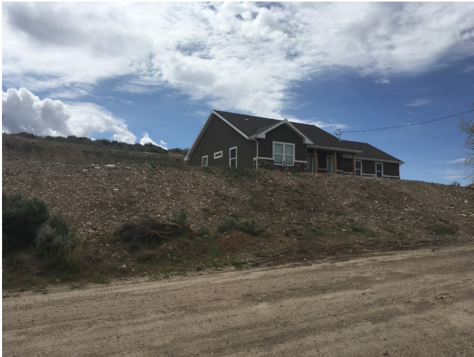
Photo 2: OU1 New Home Construction
