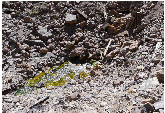
Figure 6. Mine discharge emerging from the collapsed Nelson Tunnel Portal
