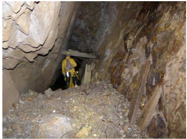
Figure 5. Large Roof Fall North of the Commodore Shaft
