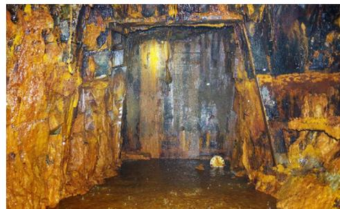
*This engineered, reinforced bulkhead (essentially a plug) controls the discharge of contaminated water from a mine.*
