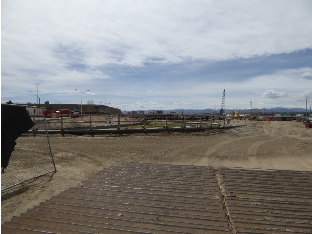
OU2 Globeville Landing Park renovation construction
