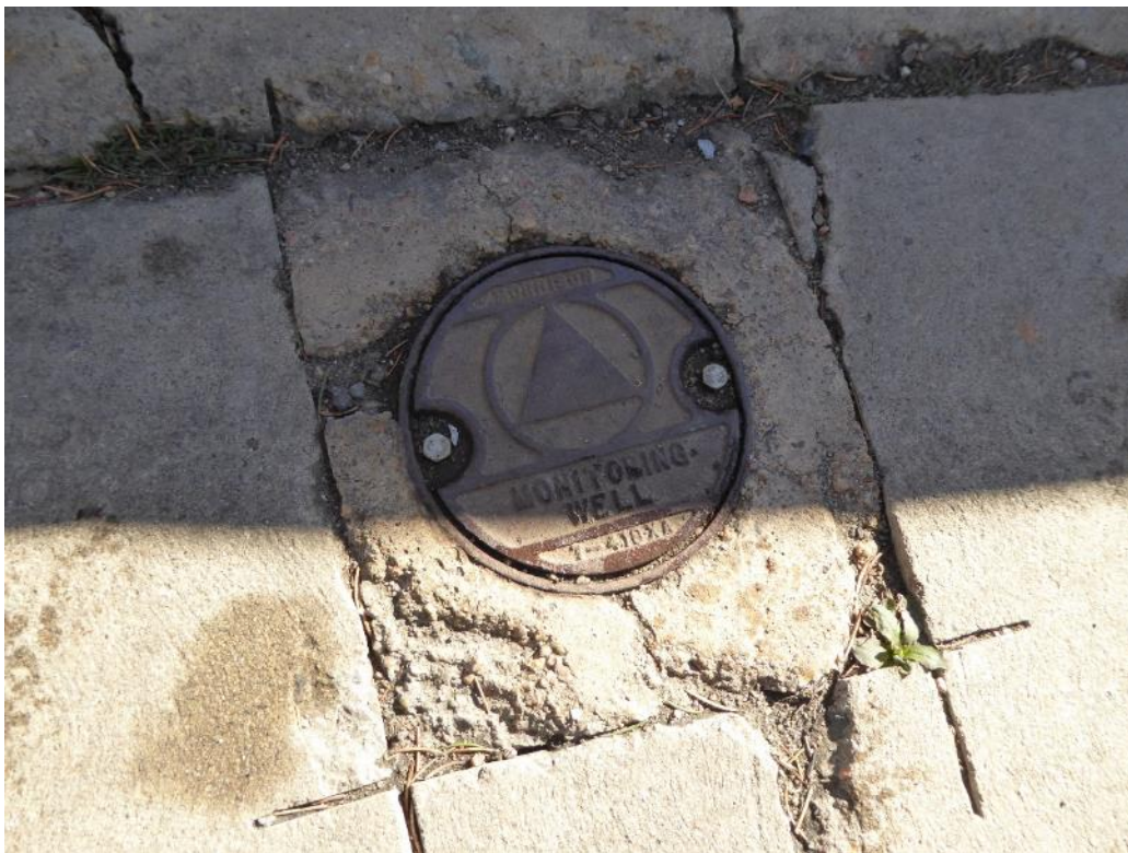
Flush-mounted monitoring well at OU3
