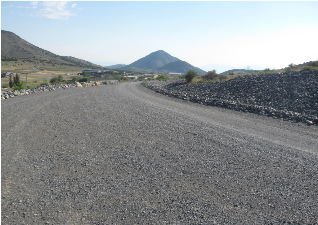
Looking east on Chief Mill Site No.1 access road
