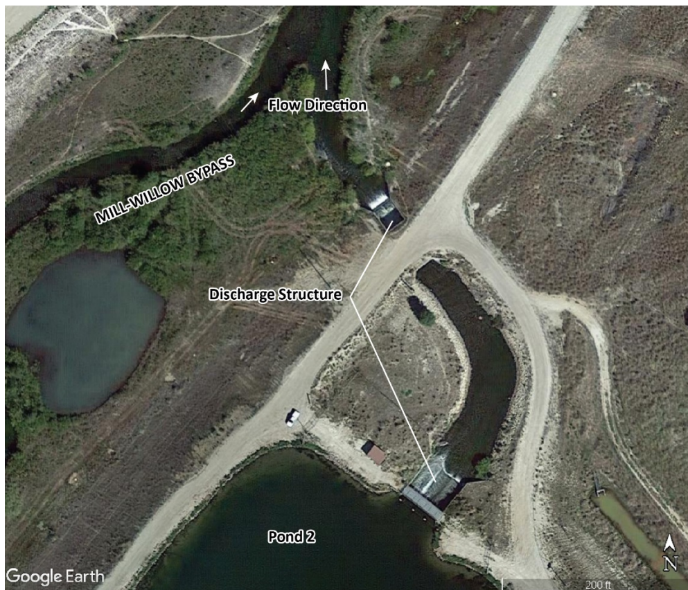
Photo 2-1. Pond 2 outfall structure and barrier to fish passage into the Ponds from the Mill Willow Bypass.
