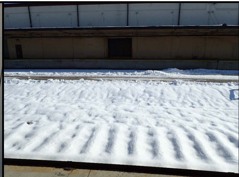
Building 16C Looking Toward Building 15C
