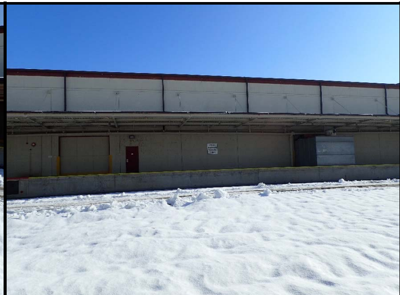
Former Trench Area between Buildings 15C and 16C
