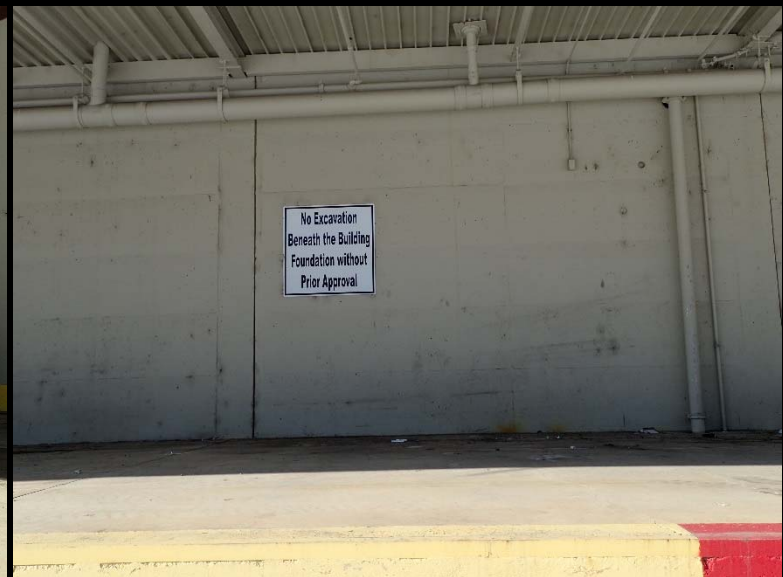
Warning Sign on Building 15C
