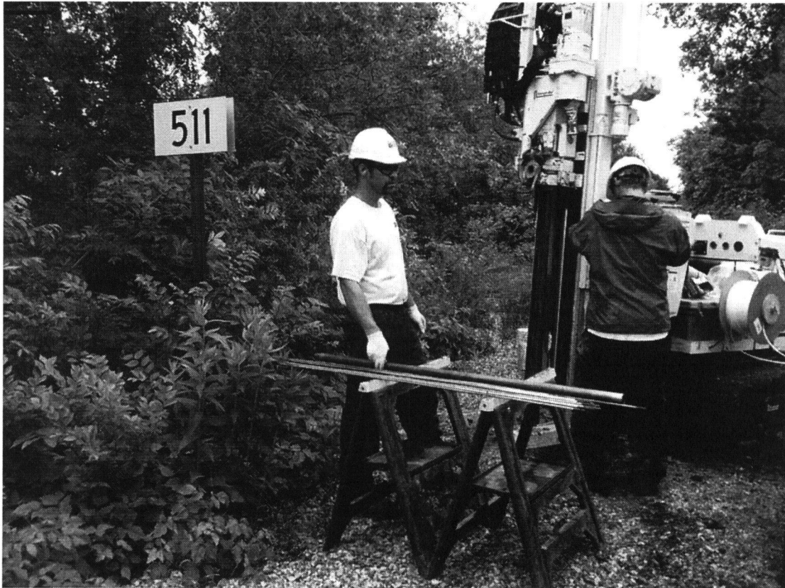
05/30/07. Facing east. Installing G-44, at north edge of former railroad track.
