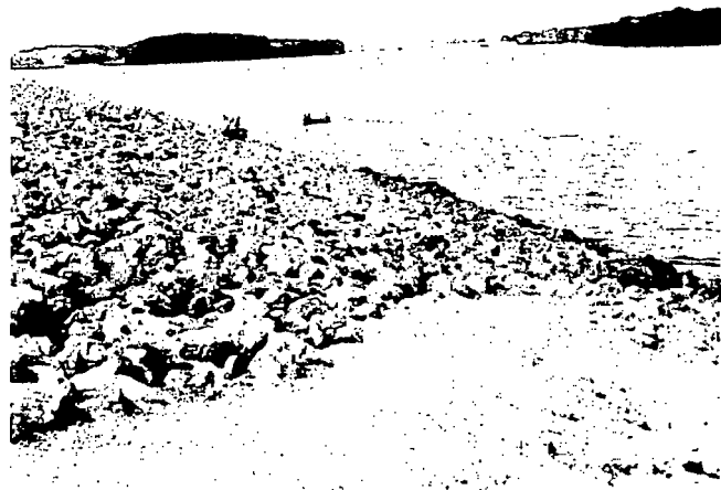
A riprapped section of shoreline on the Mississippi River. (Steve Brich photo)
