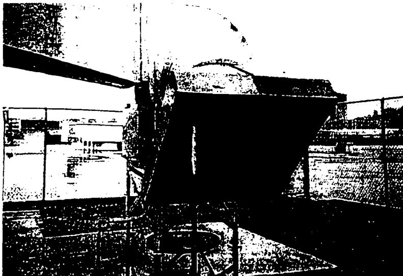
Frame 2, Air stripping tower air intake, facing N.
