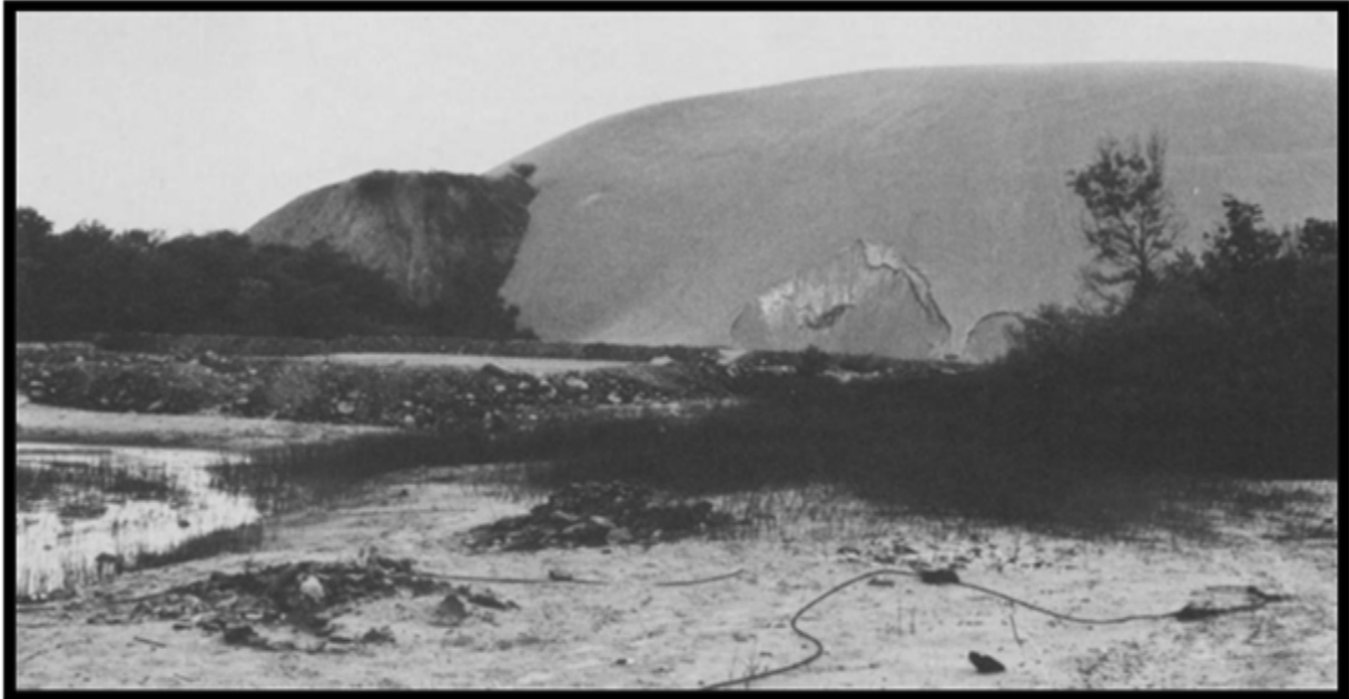
Figure 2: Historical photograph of the Elvins Mine Tailings Pile facing southeast (Whitton and Wixson, 1981). The photograph illustrates a partial pile collapse and drainage exiting the pile.
