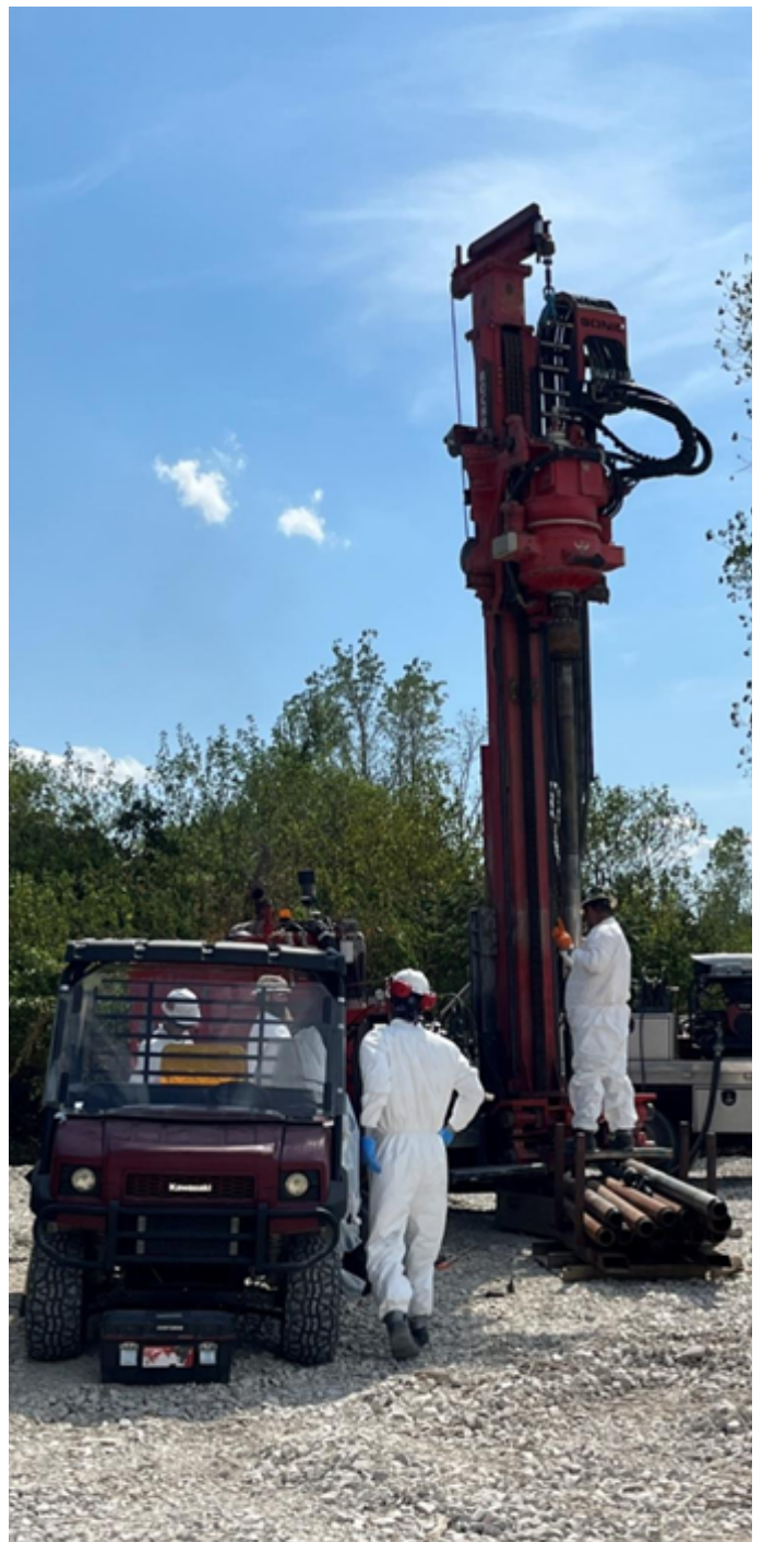
Drilling operations being conducted to collect samples in Area 1 of OU-1
