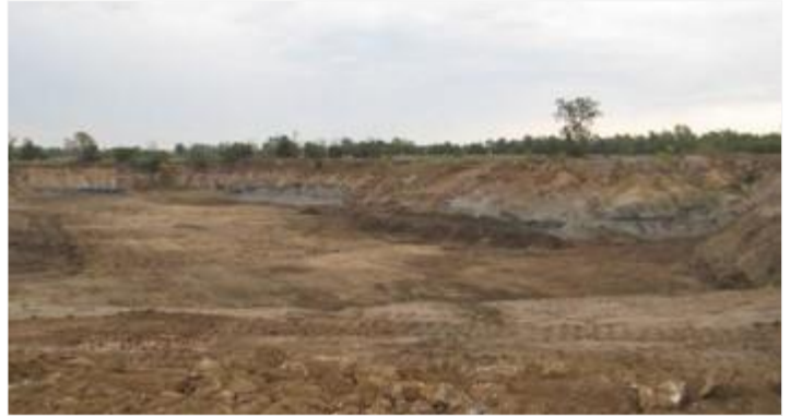
Figure 1: Ongoing cleanup at the Sunflower Pit. (U.S. EPA photo)
