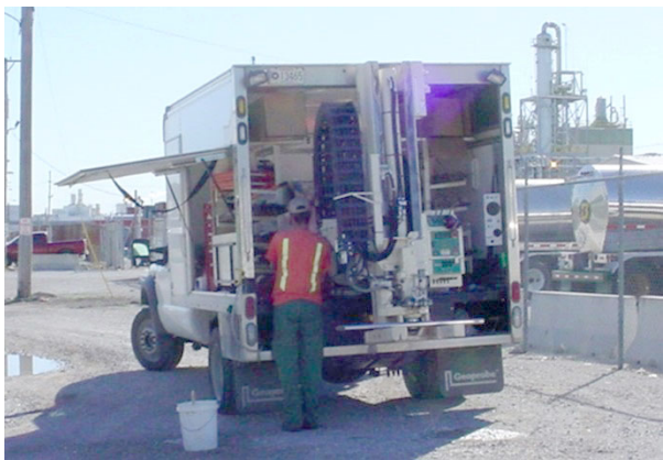
Photo of typical Geoprobe Systems DPT rig in use at a site in Region 7. Photo by EPA Region 7.
