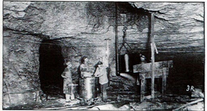
CAN OF ORE LEAVING FOR THE TOP, EAGLE-PICHER MINE, PICHER, OKLA.
