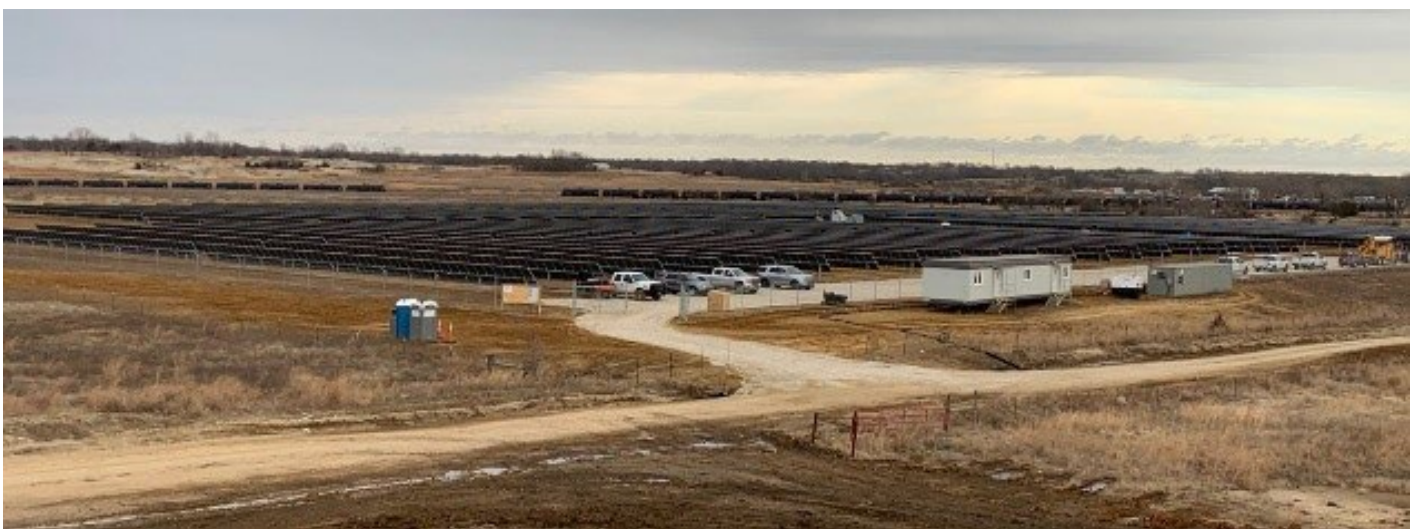
Figure 36: The Liberty Utilities community solar farm in Prosperity, Missouri.
