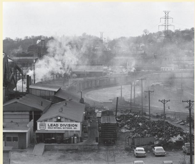
Historical images of ASARCO in 1937 (top) and Gould Electronics, Inc. in 1968 (bottom) show dense clouds of smokestack emissions that led to deposition of lead over 27 square miles of downtown Omaha. Image from the Omaha World-Herald/John Savage Photography Collection at The Durham Museum, used with permission.
