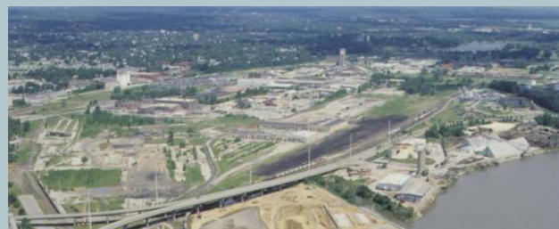
The former ASARCO facility property after demolition.
