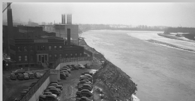
Installation of flood walls helped protect the ASARCO facility from flooding. Image from the Omaha World-Herald/John Savage Photography Collection at The Durham Museum, used with permission.
