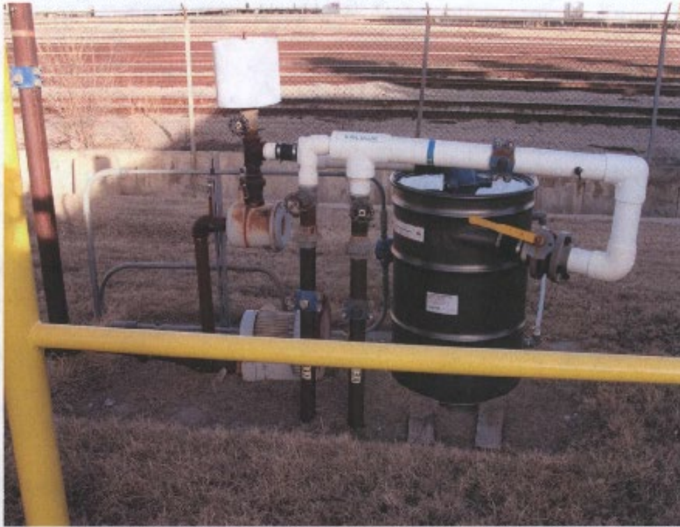
Photo 6. South Field Soil Vapor Extraction System (SVES)
