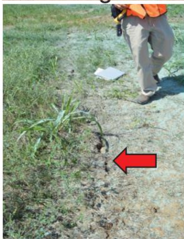
Figure 8 - Surface Cracks from Subsidence Settlement at Bridgeton Landfill, OU-2 (Ref 7)
