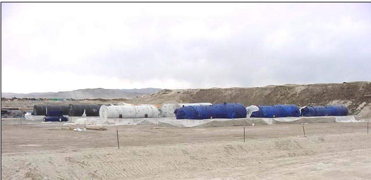
Figure 3-2. Large Component Disposal
