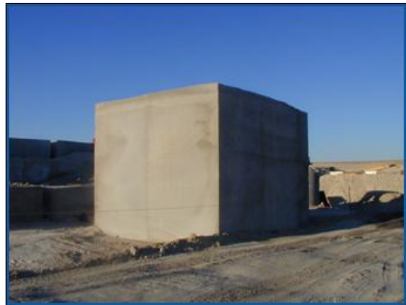
Figure 3-1. Macroencapsulation of Hazardous Debris
