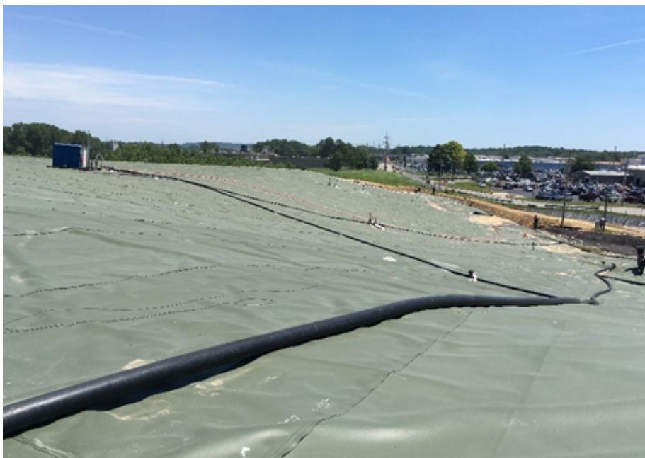
Newly installed EVOH cover in the North Quarry of the Bridgeton Landfill.
