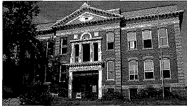
Robbins during renovation in 1999
