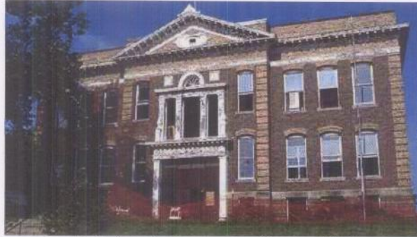
Robbins during renovation in 1999
