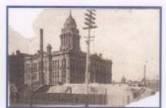
Douglas County Court House looking ne from 18th & Harney during Leveling Project
