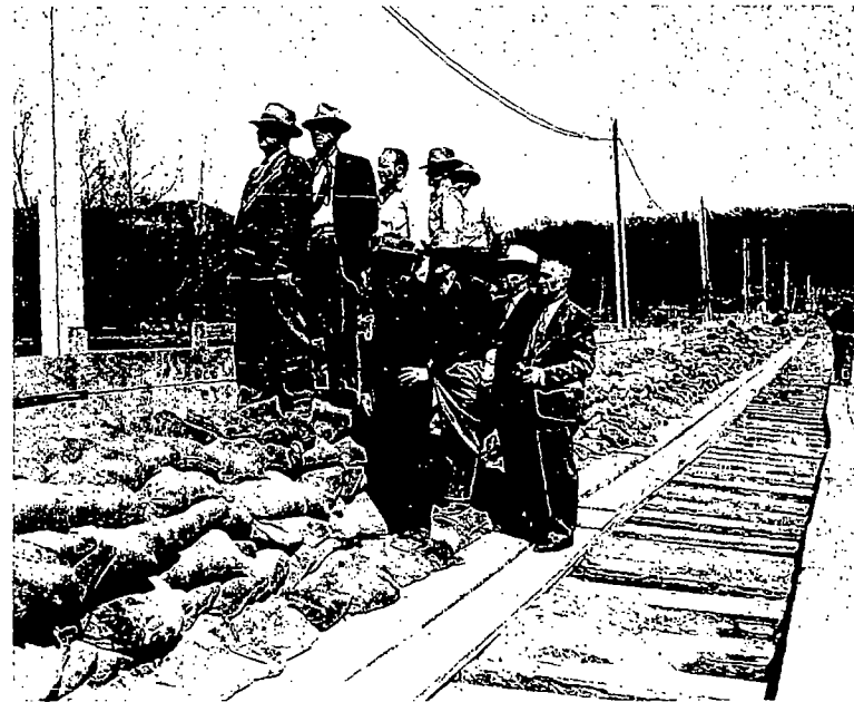
Watchful eyes look to the rising river levels atop countless sandbags filled by hundreds of volunteers working day and night to save Council Bluffs and Omaha.
