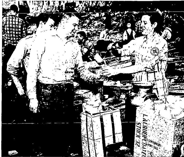
Lunch on the levee is necessary to keep hard-working men on the job day and night. Mrs. Charles Milner of Council Bluffs is serving coffee to Bill Guyer, an Omahan who came over to work on the local levee-building project. Sandwiches and hot meals were also served workers.
