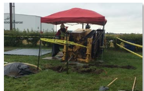
Figure 4. Construction of the SVE system. (Image source: SMC)
