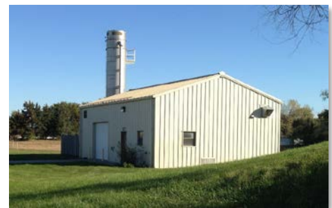
Figure 3. View of the on-site groundwater extraction and treatment system. (Image source: SMC)
