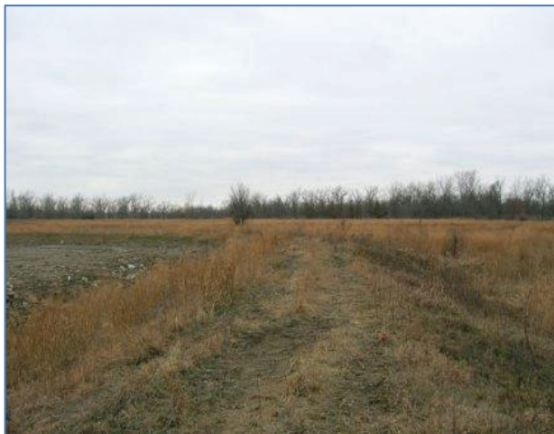
OU 1 - View of the Muncie site dike
