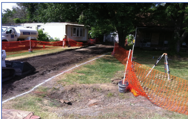
OU2 – Town of Afton Driveway Excavation
