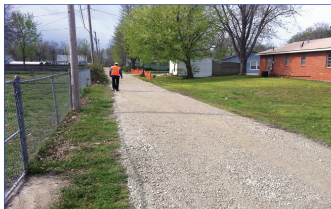
OU2 – City of Miami Restored Alleyway
