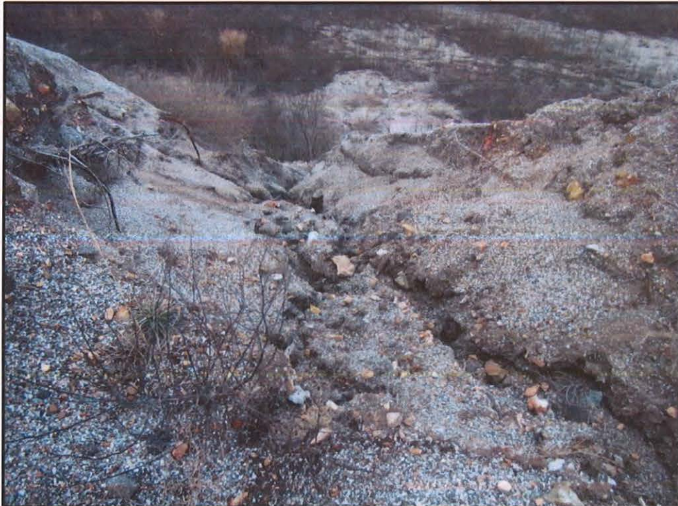
Photo 17: Erosion of Northeastern Side of Central Mill Repository
