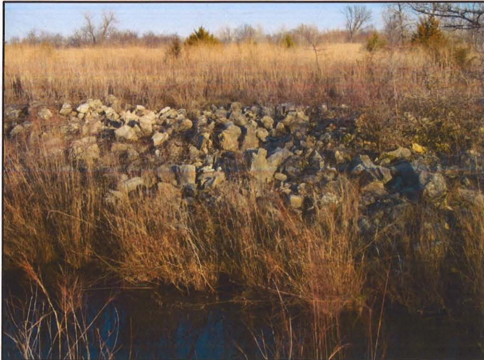
Photo 21: Rip-rap of Diversion Channel at Admiralty Mine Site
