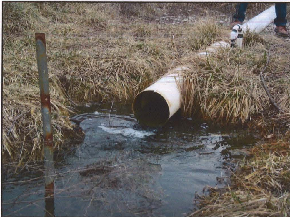
Photo 8: Outflow of Polishing Basin from MRPTS
