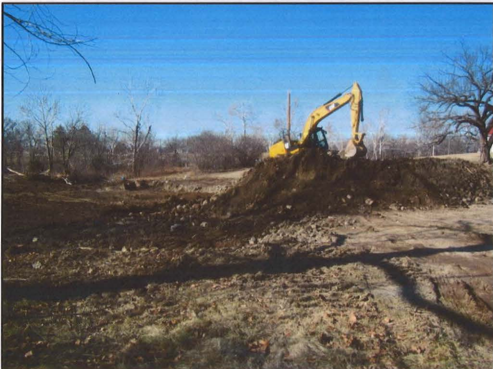
Photo 40: Excavation of Chat from Distal 6A
