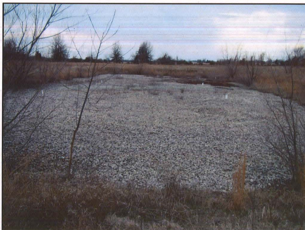
Photo 6: MRPTS Horizontal-flow Limestone Bed
