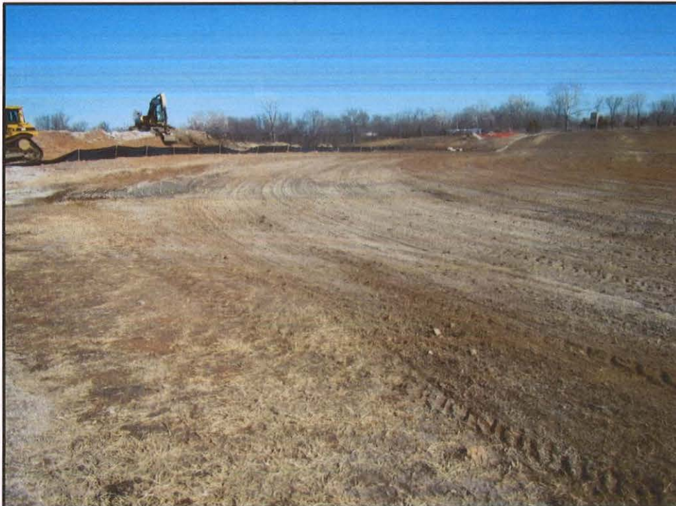
Photo 38: Soil Amendments Placed on Catholic 40 Site
