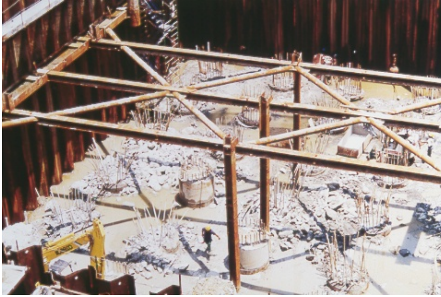
Figure 10 - Cofferdam for the Sidney Lanier Bridge, Oregon
