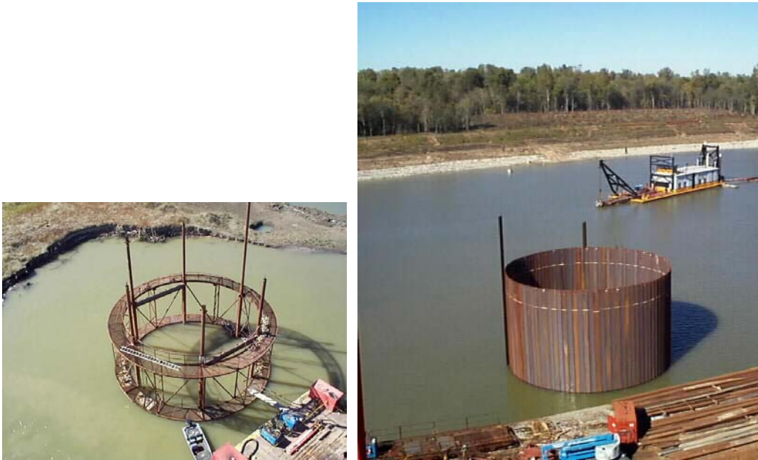
Figure 12 – Installation of wale and strut system and driving the sheet piles
