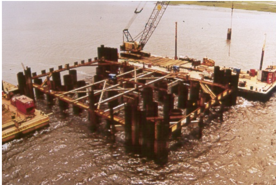
Figure 11 – Installation of wale and strut system
