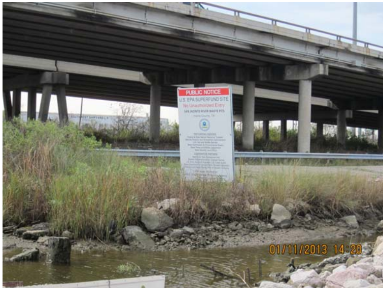
Photo 11: Public notice sign north of I-10 along southern berm (view southwest)
