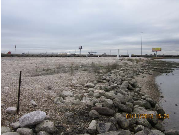
Photo 21: Western edge of the Western Cell (view south)
