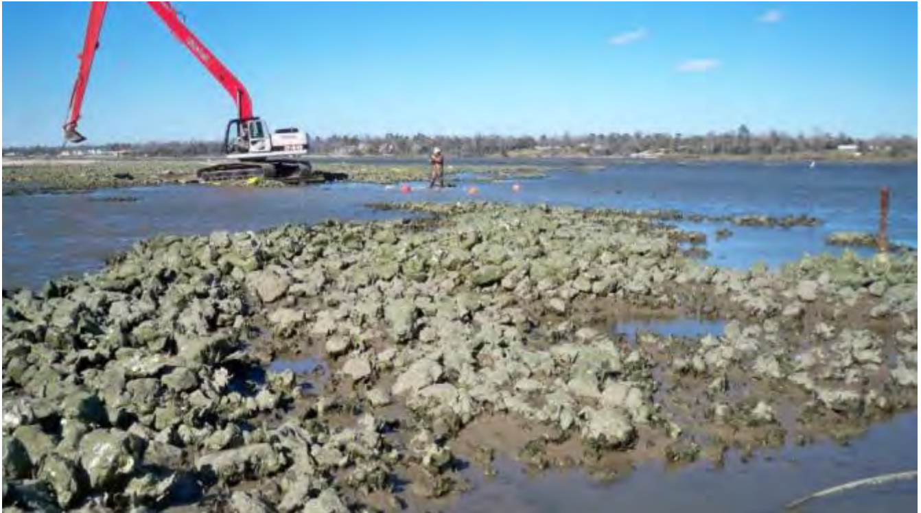
Photograph 4 – Surveyor checking MA 4 surface before demobilizing long reach excavator.
