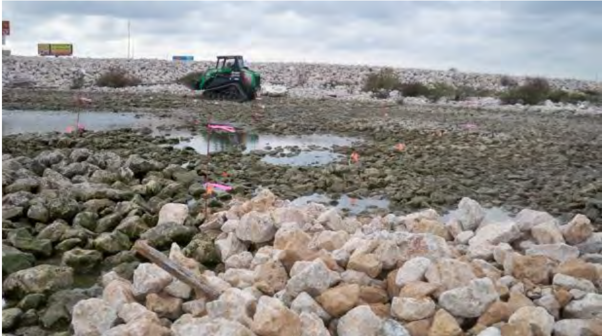
Photograph 2 – Skid Steer returning to temporary stockpile. Pin Flag marking MA 1.
