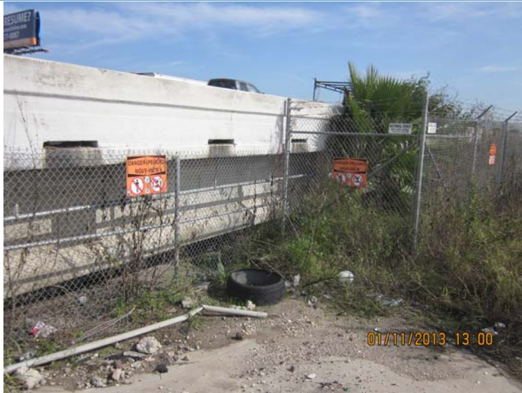
Photo 01: Warning sign and perimeter fence south of I-10 on west bank (view northeast)
