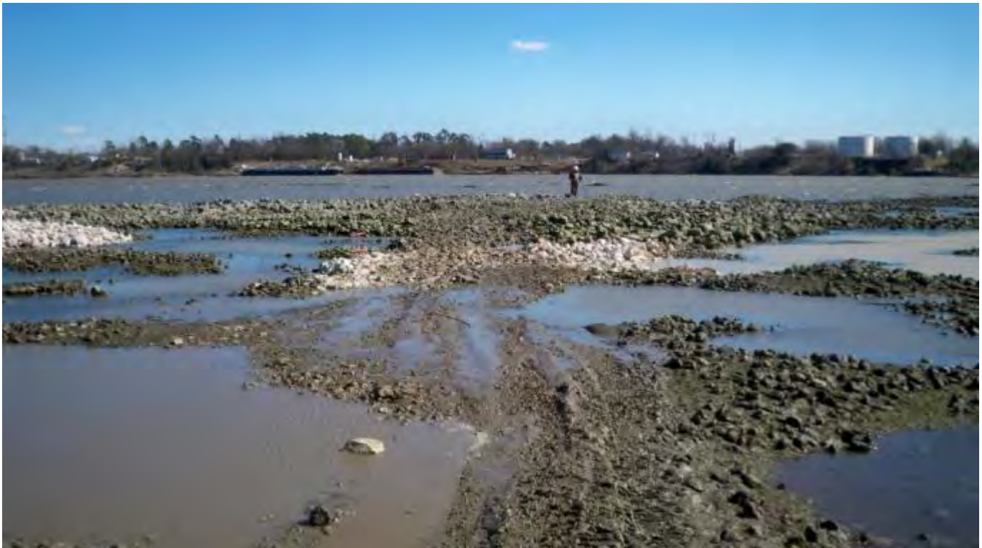
Photograph 1 - Completed MA 2 in foreground, surveyor marking MA 3 in background.
