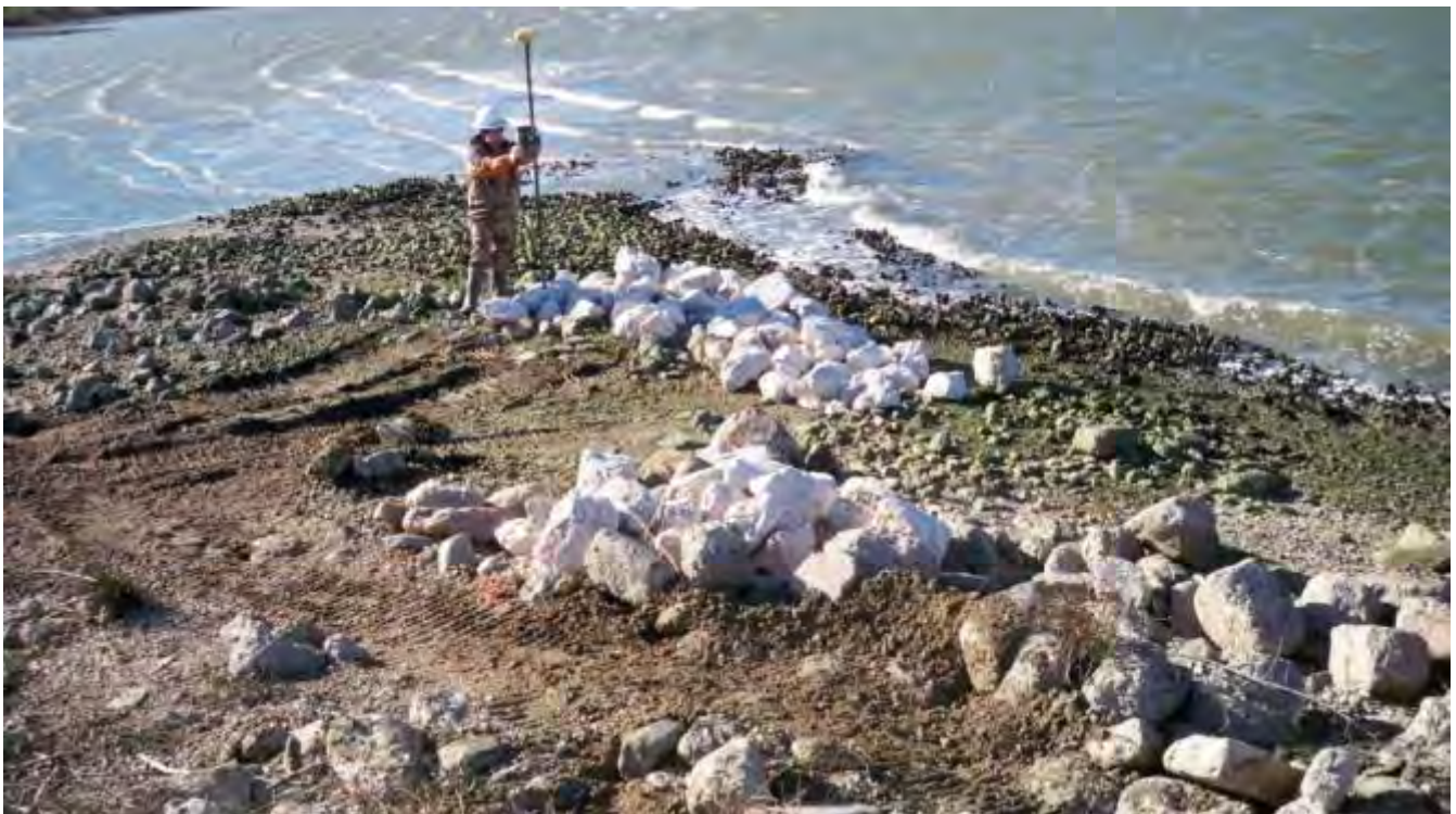
Photograph 5 – Surveyor checking lap joint maintenance, NW corner western flats. Photograph from atop western berm.
