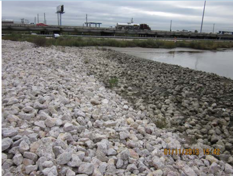
Photo 25: Southern end of the west berm; color variation in armor rocks indicates the submerged portions of the cap under normal tidal conditions (view southwest)
