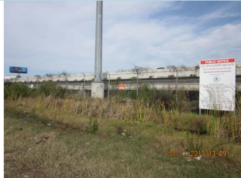
Photo 02: Public notice sign south of I-10 (view north)
