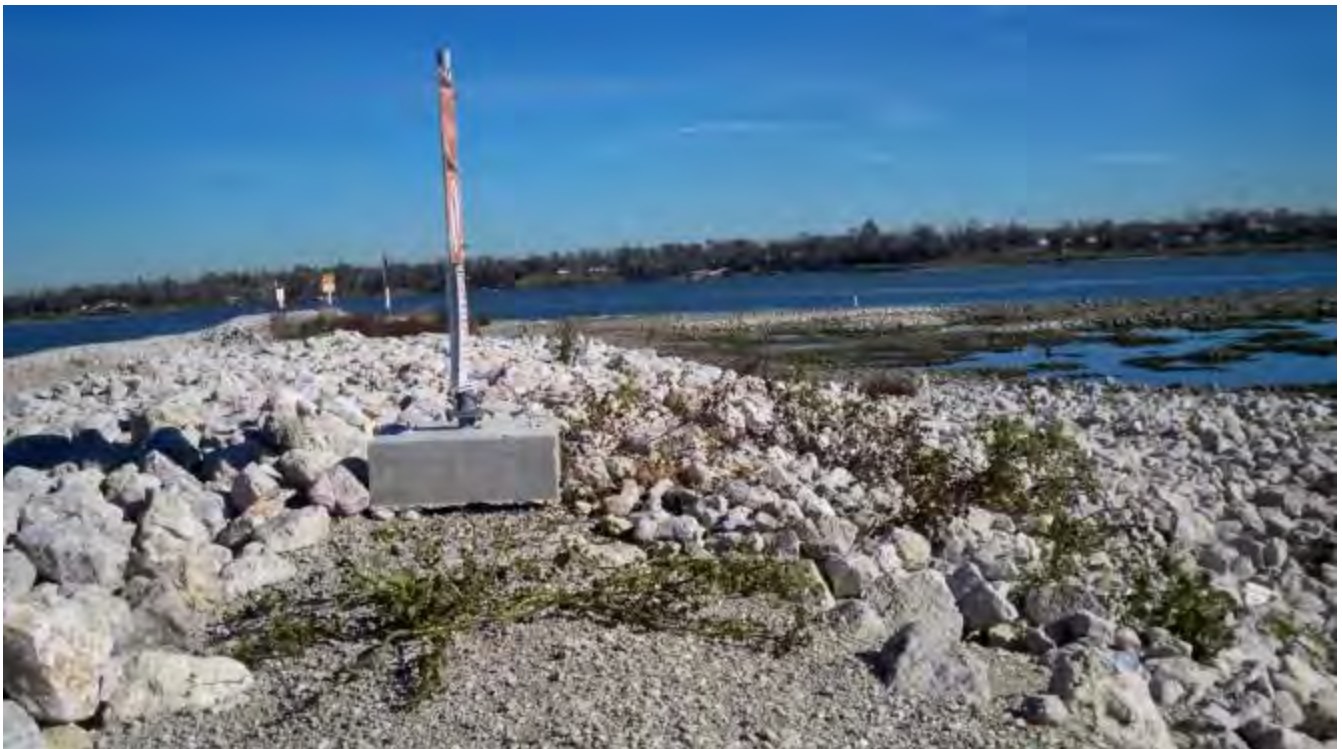
Photograph 3 – Woody stem vegetation cleared from signage on central berm.
