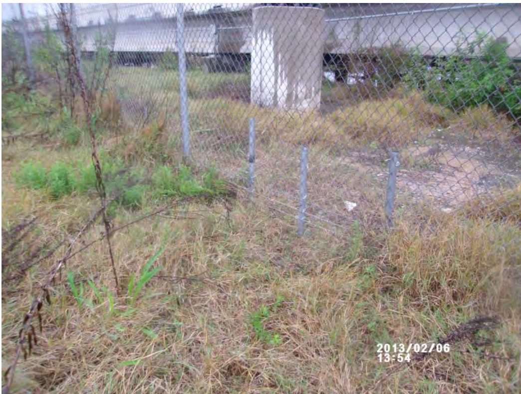
Photograph 3 – Added barb wire and fence supports to prevent access, south fence line, west bank.
