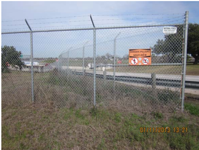
Photo 03: TCRA Site security fencing on the east bank (view north)
