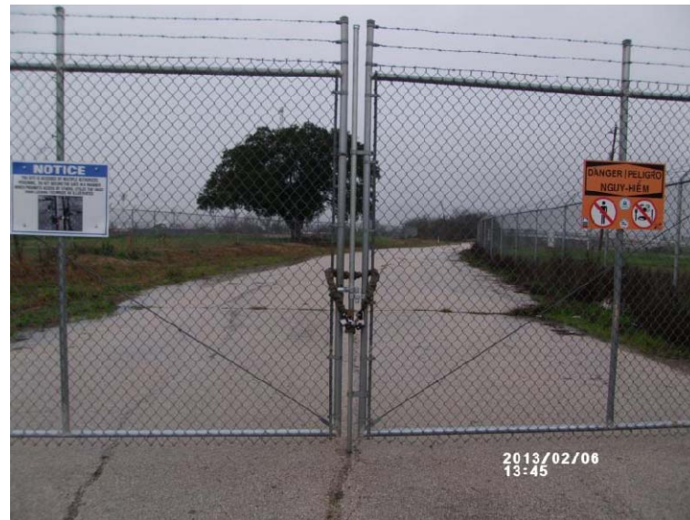
Photo 28: New gate center post installation, east bank (view north)
