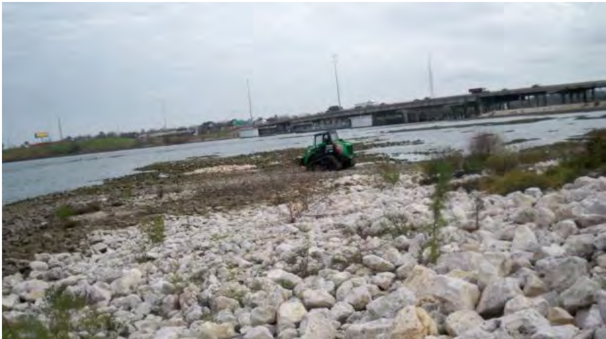
Photograph 1 – Skid Steer carrying Rock Type C to MA 1.
