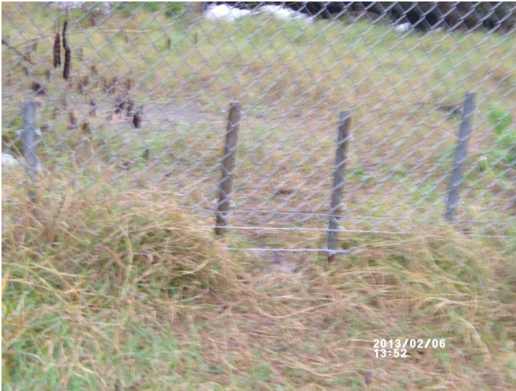
Photograph 2 – Added posts and barb wire closures, south fence alignment, west bank.
