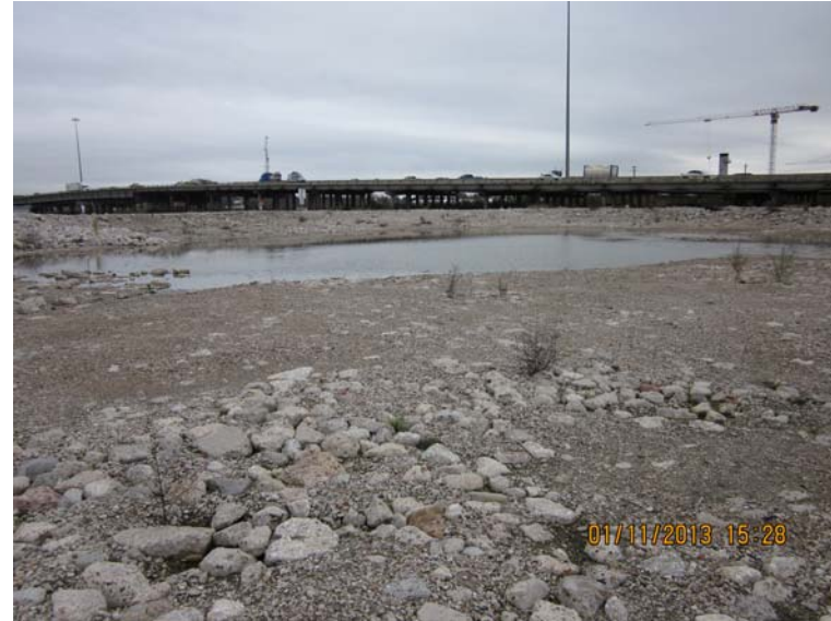
Photo 22: Interior view of the Western Cell with standing water in the background along the central berm (view southeast)
