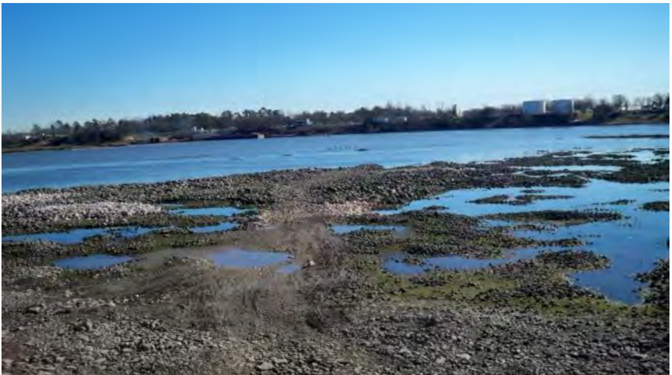
Photograph 7 – MA 1 and 2 and showing access lane to MA 2 and 3. MA 3 in the distance.
