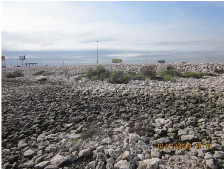
Photo 19: Northern portion of the Eastern Cell; color variation in armor rocks indicates the submerged portions of the cap under normal tidal conditions (view west)
