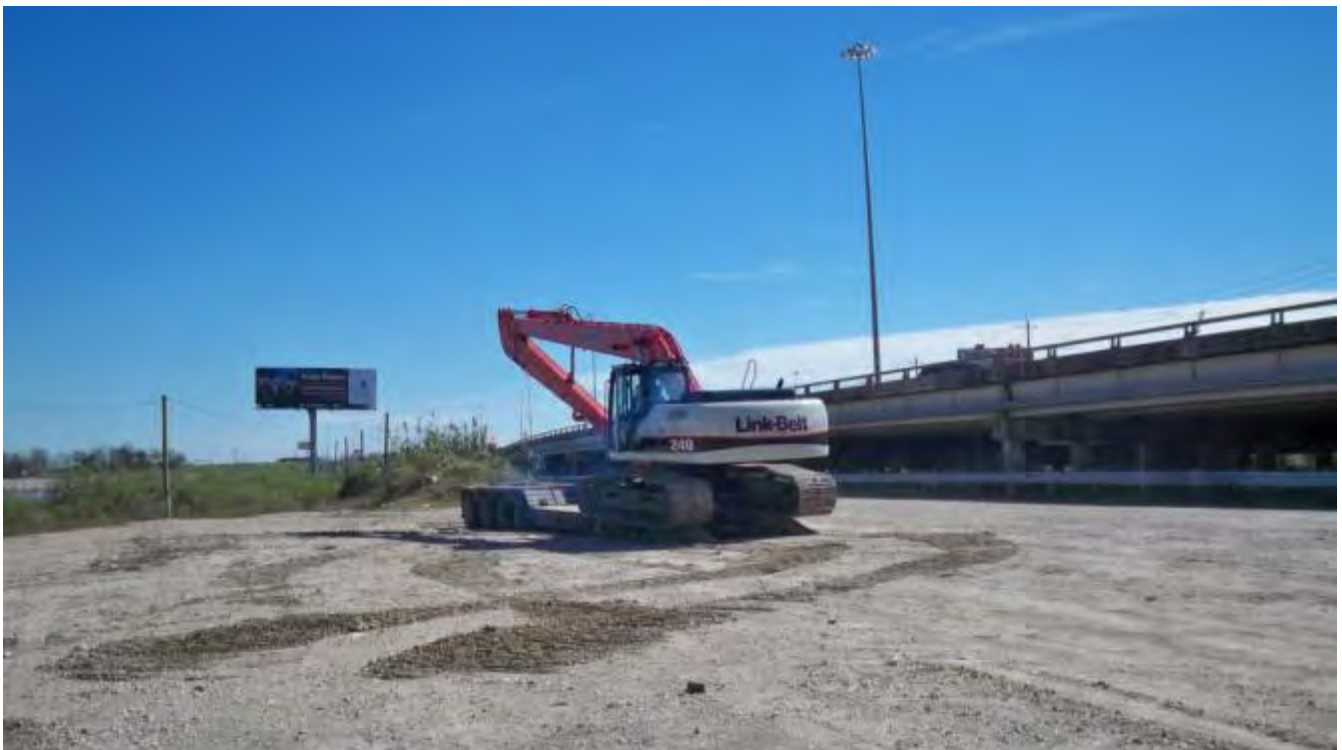
Photograph 5 – Linkbelt excavator demobilized from site.
