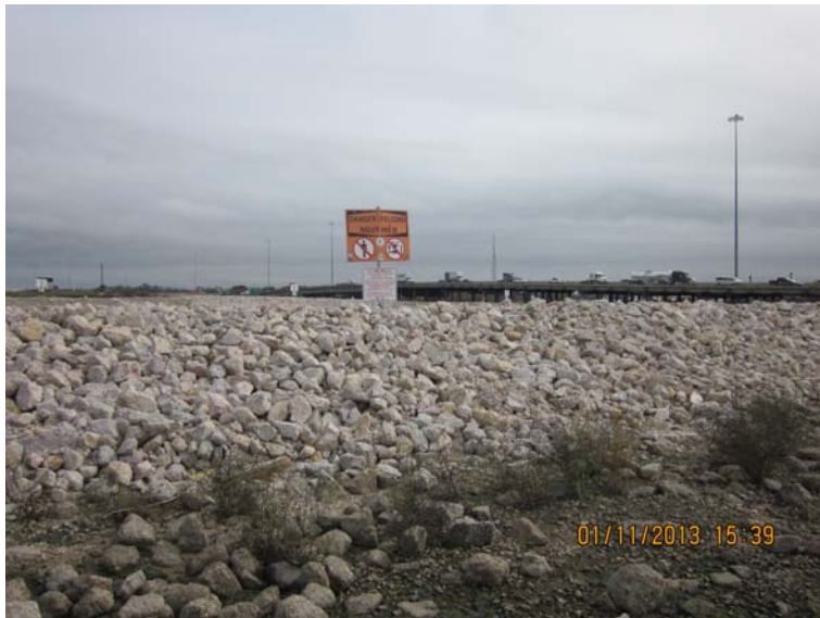
Photo 23: Warning sign on west berm (view east)
