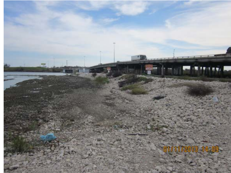
Photo 10: Northern face of southern berm and warning signs (view east)
