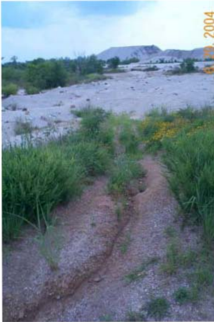
Photo 12: View along the south side of the diversion dike at the Admiralty Mine site.
