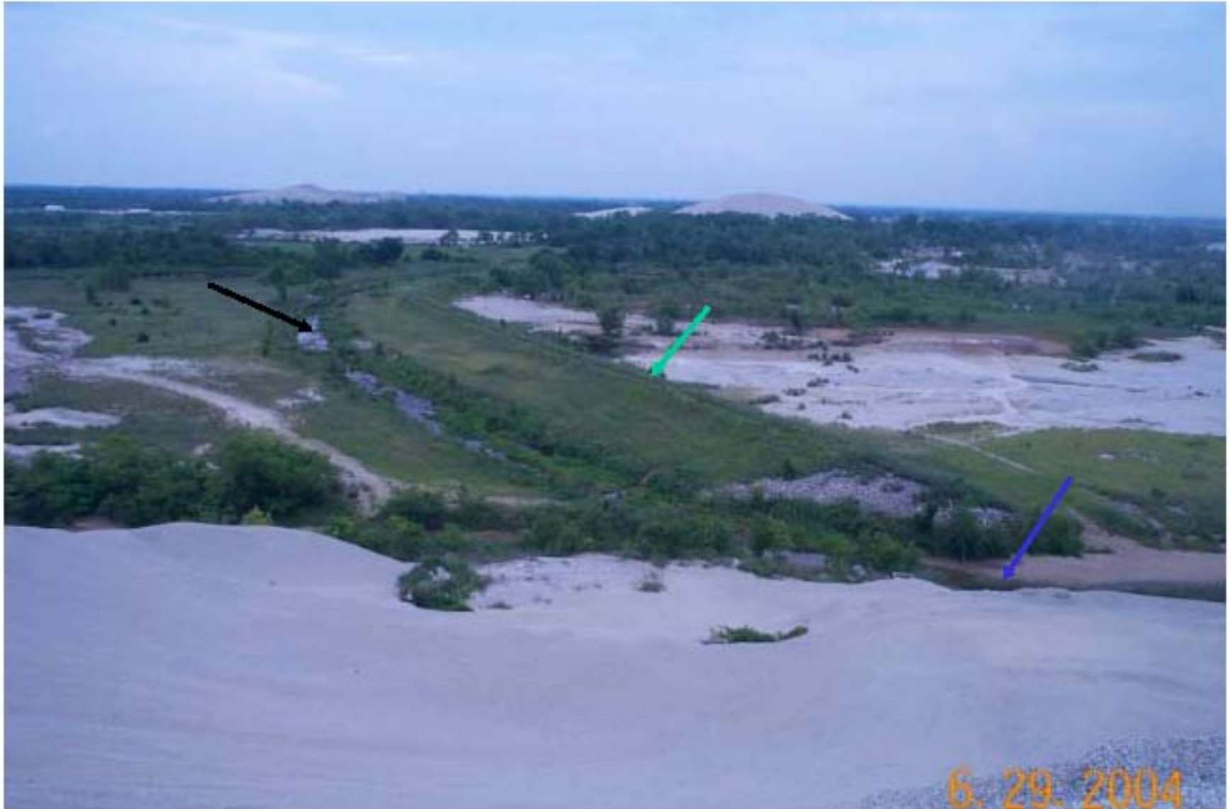
Photo 17: View of diversion dike (green arrow) at Admiralty Mine site from the top of a chat pile located west of Tar Creek. Tar Creek flows along the base of the chat pile (blue arrow). The diverted Lytle Creek channel is located at the black arrow.
