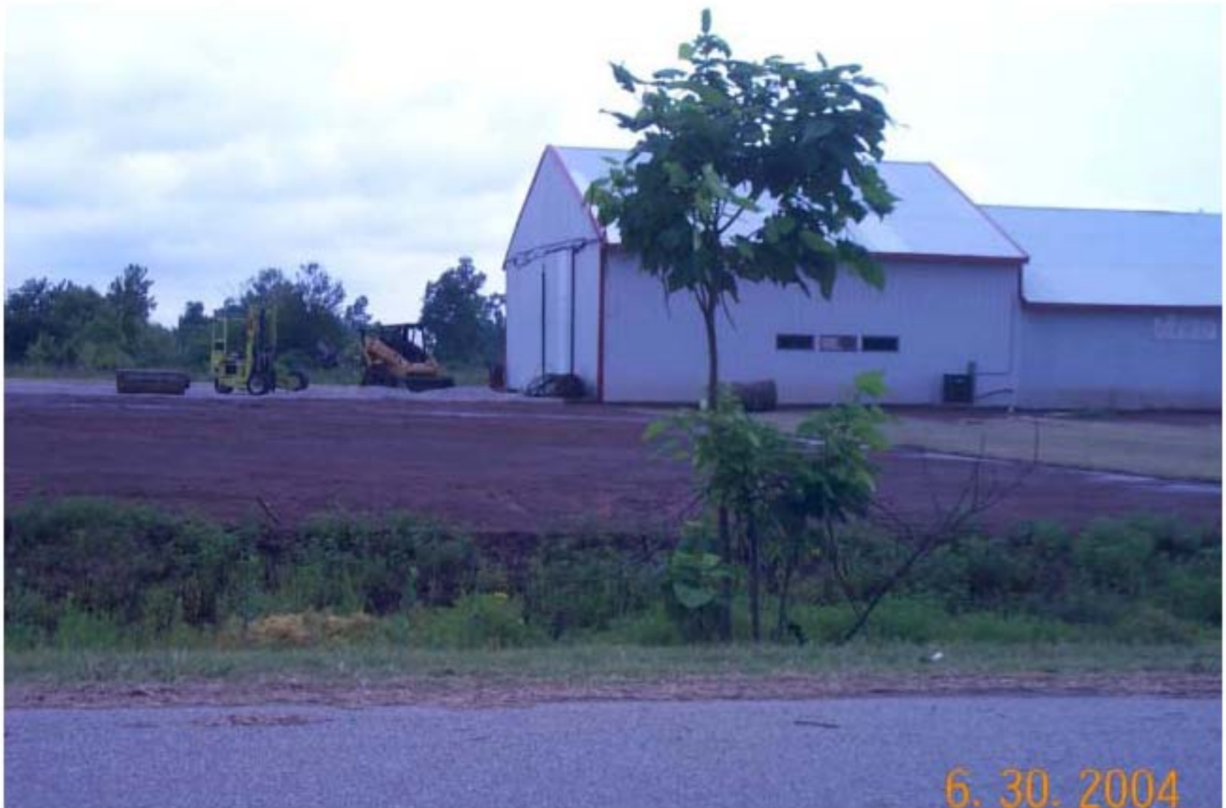
Photo 33: View of property in North Miami, Oklahoma. Construction was not complete at the time of the site inspection. Area in the foreground is where replacement sod has not yet been placed.
