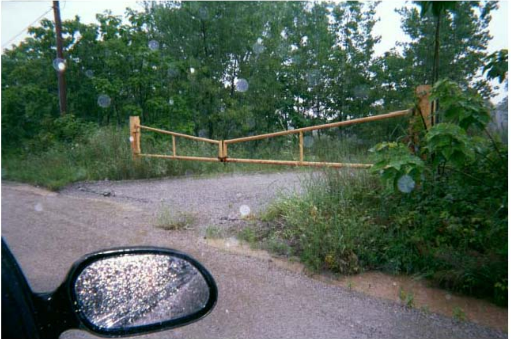
Photo 72: View of front gate at the north repository, located just west of US Highway 69 in Picher.
