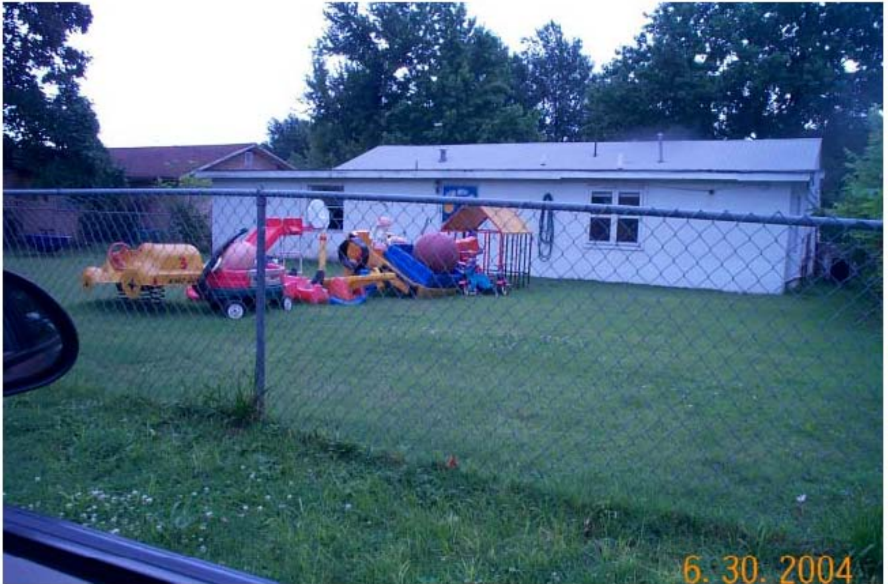
Photo 29: View of remediated area on play ground at a daycare facility, Miami, Oklahoma.
