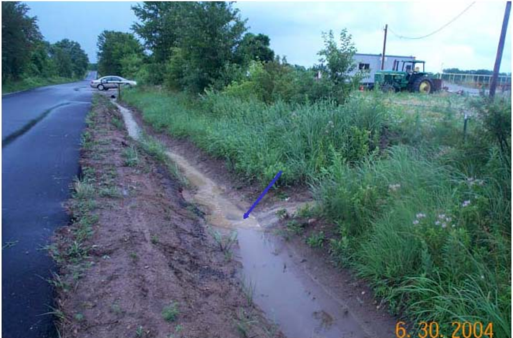
Photo 50: View of drainage ditch where runoff enters from the borrow source property. Discoloration of the runoff in the drainage ditch is apparent where the runoff enters the ditch (blue arrow).
