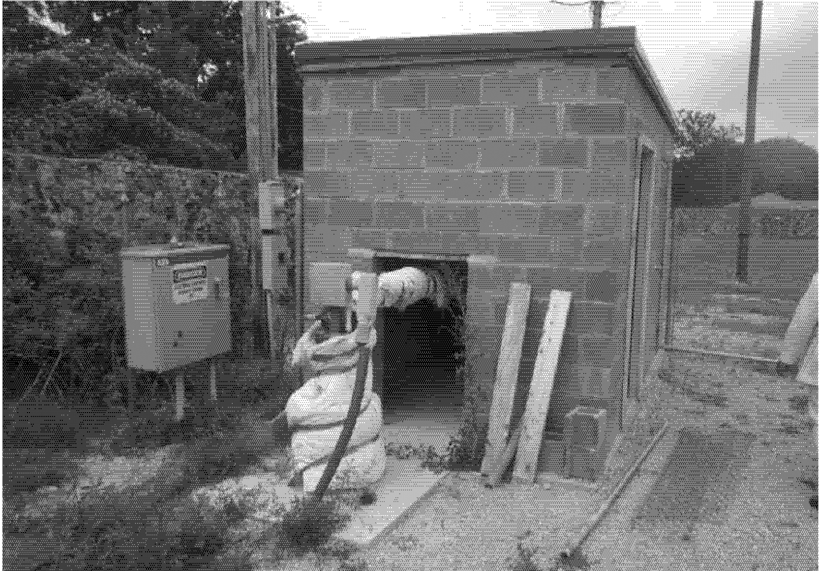
Photo 1: View of the Commerce #5 MW. The City of Commerce has erected a well house over the well-head in preparation for connecting the well to the public water supply.
