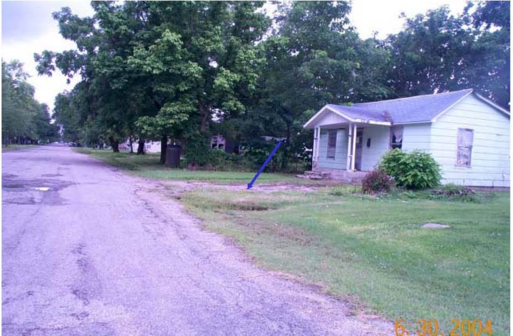
Photo 37: View of unremediated properties on Vine Street in Commerce, Oklahoma (view is to the south). Chat is present in the driveway in the center of the photo (blue arrow).
