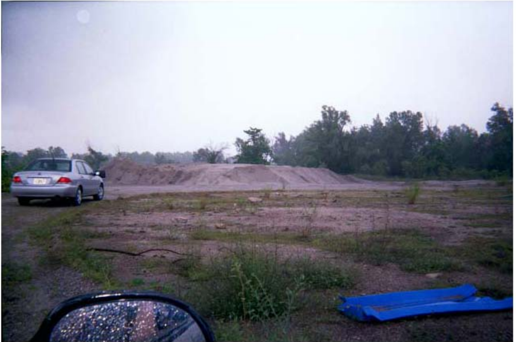
Photo 68: View of the north repository, located just west of US Highway 69 in Picher. Piled dirt in background is an old chat pile.
