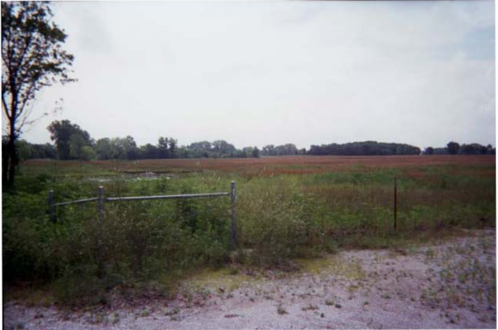
Photo 56: View of pilot project location. This project was executed by the State of Oklahoma and involved the removal of chat at the surface, placing the chat within subsidences and abandoned mine shafts, and the filling in of a mill pond. This photo shows the surface after the project was completed.
