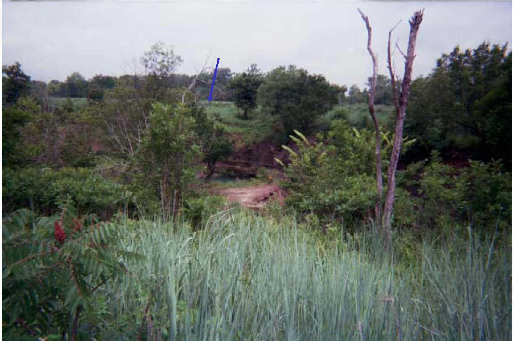
Photo 59: View of subsidence at the Big John Mine site, located in Kansas, facing northwest. This subsidence feature is surrounded by a diversion dike to prevent inflow of water into the mines. Tar Creek was diverted around the subsidence to the west (behind dike in background at blue arrow).
