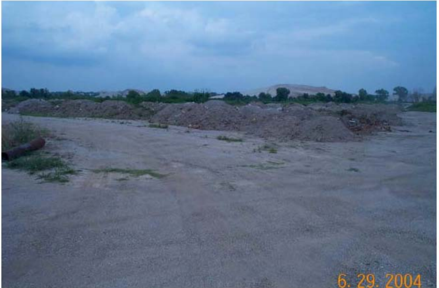
Photo 26: View of recently deposited soil at the repository on E40 Road. Lead contaminated soil from residential yards is used at the repository to fill in an old mill pond.
