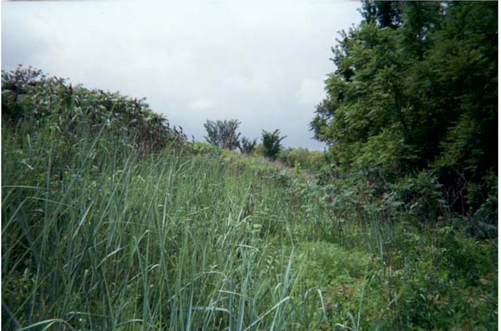
Photo 61: View of vegetation on the diversion dike at the Big John Mine site, located in Kansas.
