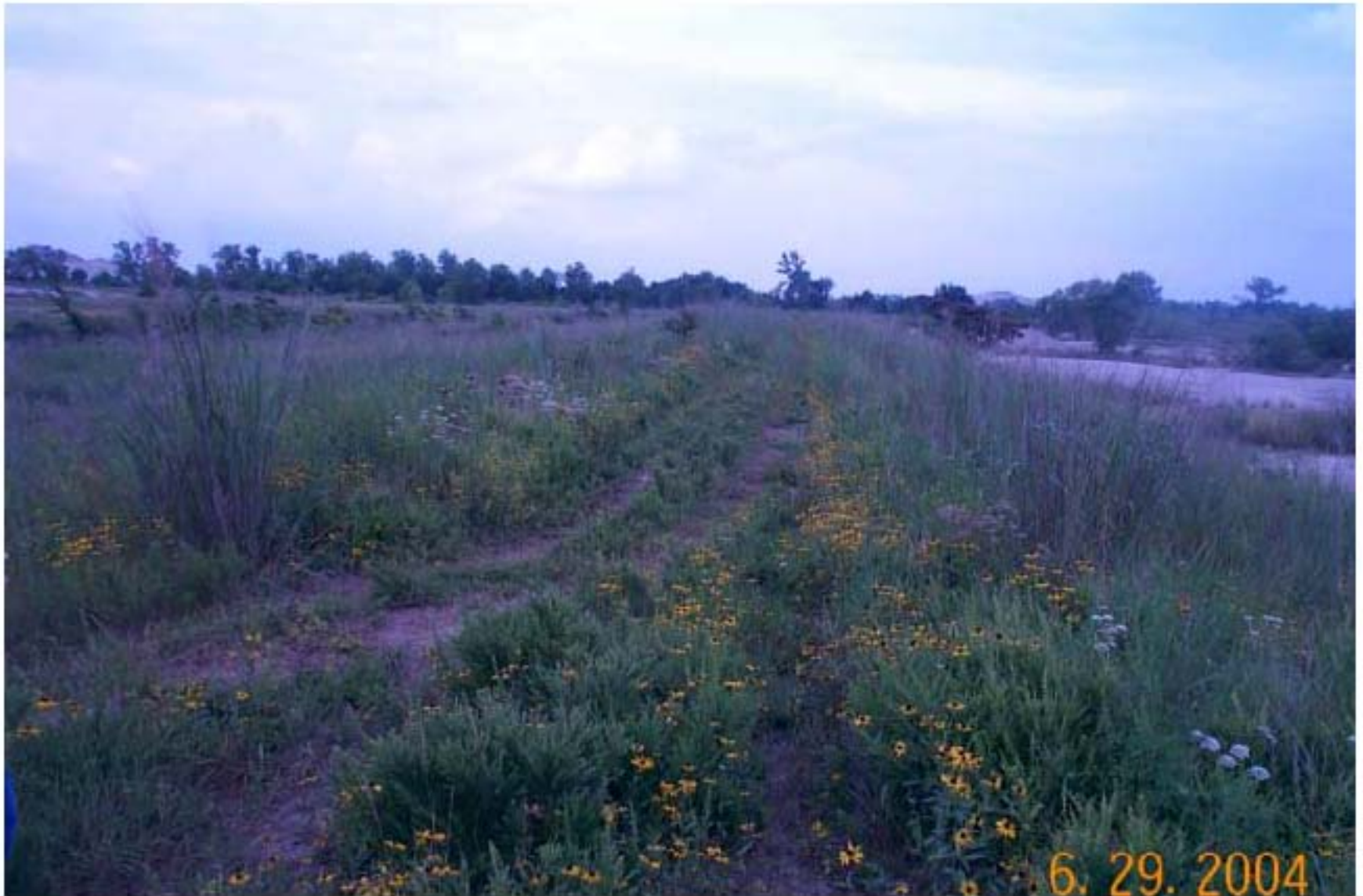
Photo 16: View of diversion dike looking east from Tar Creek.
