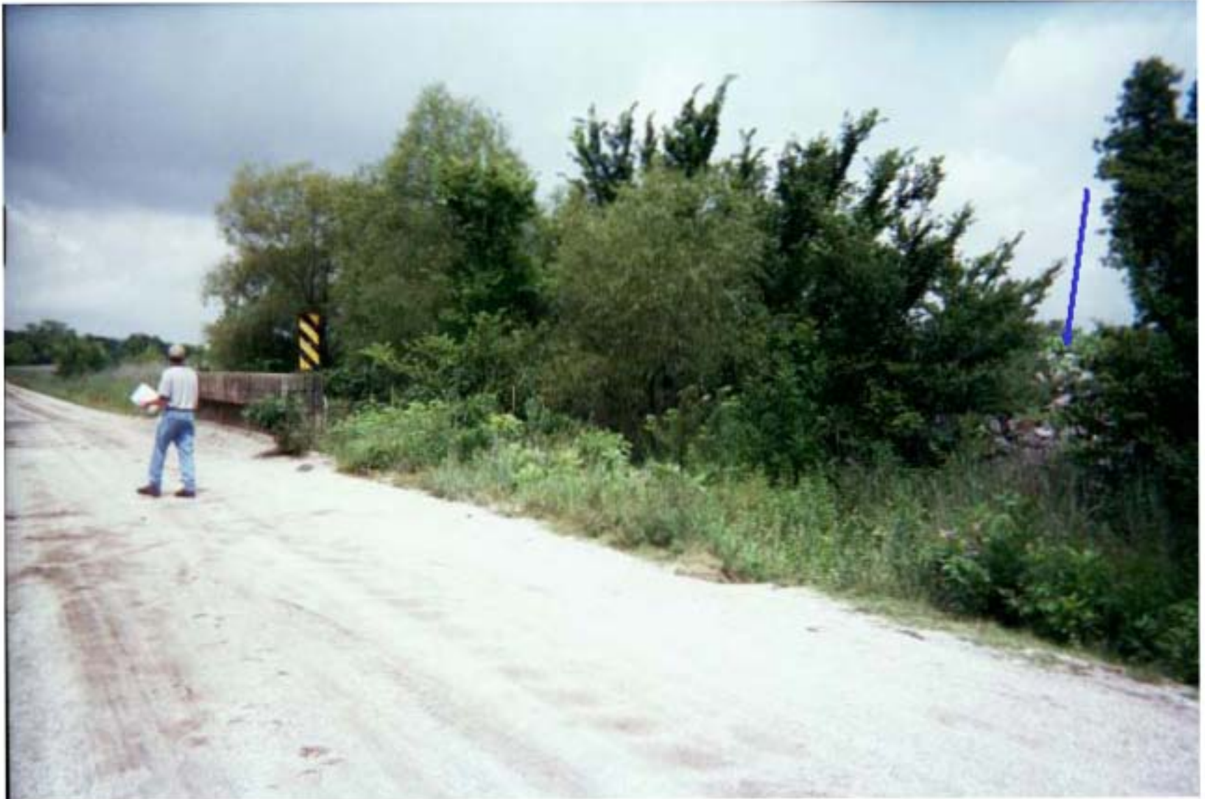
Photo 66: View of road on south side of diversion dike at Big John Mine site, located in Kansas. The backside of the diversion dike is barely visible through the trees (at blue arrow). The bridge is where the old Tar Creek channel used to flow.
