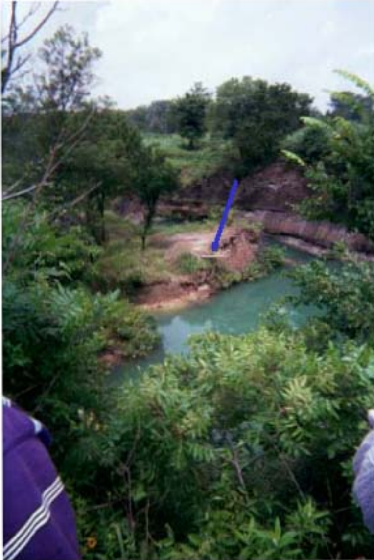
Photo 60: View inside subsidence at the Big John Mine site, located in Kansas. A diving board is visible in the center of the picture (at blue arrow). ODEQ noted that this location is frequented by swimmers.
