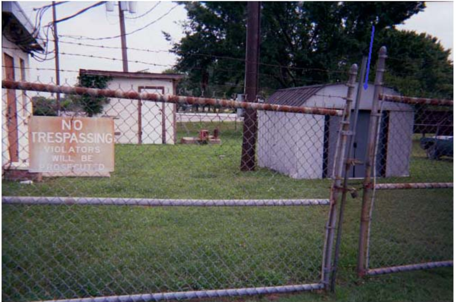
Photo 53: View of Quapaw #2 well location. Well is located inside shed at right (blue arrow).
