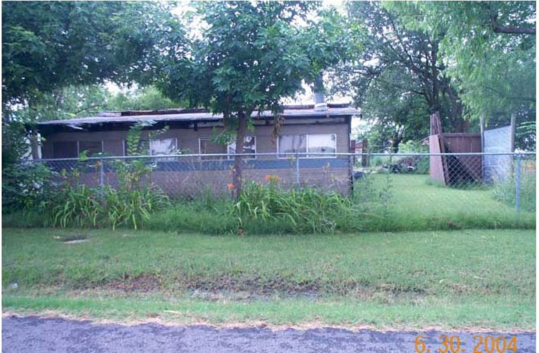
Photo 30: View of remediated property in North Miami, Oklahoma.
