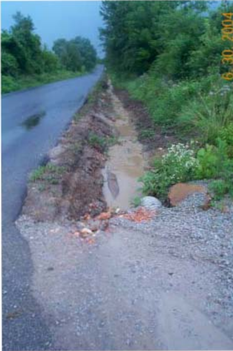
Photo 48: View downstream in the drainage ditch and culvert at entrance to borrow source. Runoff water in the drainage ditch is discolored from silt.
