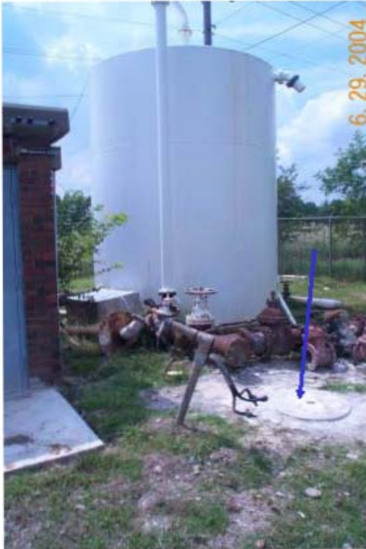
Photo 2: View of the plugged Commerce #3 well (blue arrow). White tank in background receives and stores water from the Commerce #4 well (located to the east of this location). Building at left is where chlorine is added to the water prior to entry into drinking water system.
