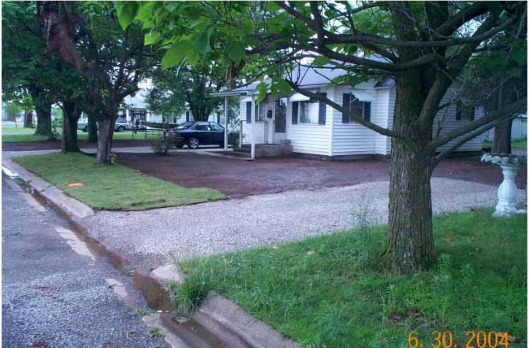
Photo 36: View of property in Commerce, Oklahoma. Construction was not complete at the time of the site inspection. Remediated portion of the yard (bare area in middle of photograph) is awaiting the placement of sod.
