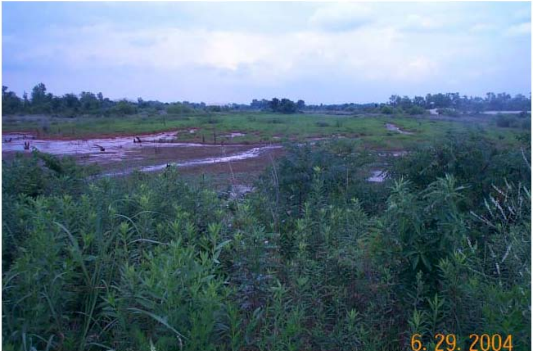
Photo 7: View of diverted Lytle Creek from on top of the dike at the Admiralty Mine site. View is towards the east.
