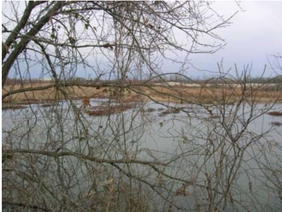
Photo 39: View of water-filled collapse feature on southwest side of Admiralty diversion dike. Water discharges towards the southwest towards Tar Creek. View is to the southwest.
