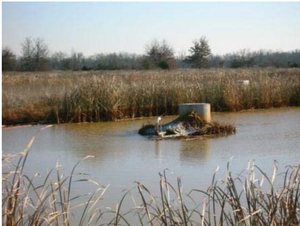
Photo 68: View of iron settling pond at Meyer Ranch. Part of University of Oklahoma constructed wetlands treatment system.
