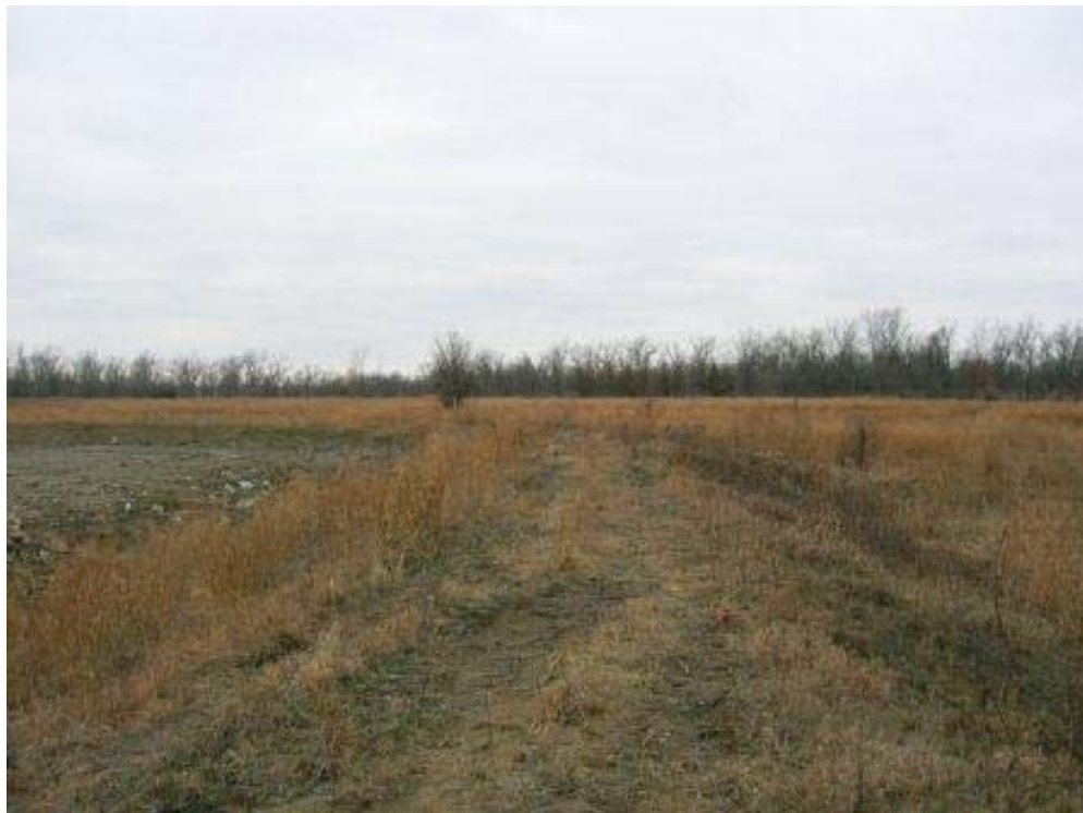
Photo 10: View of the dike at the Muncie site. The subsidence (at left) has been filled in. Diverted Tar Creek channel is in the tree-line in center background. View is facing north.
