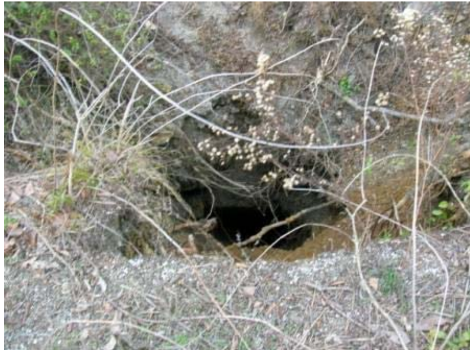
Photo 26: View of mine shaft collapse on the east side of Picher near Picher Well No. 6-MW.
