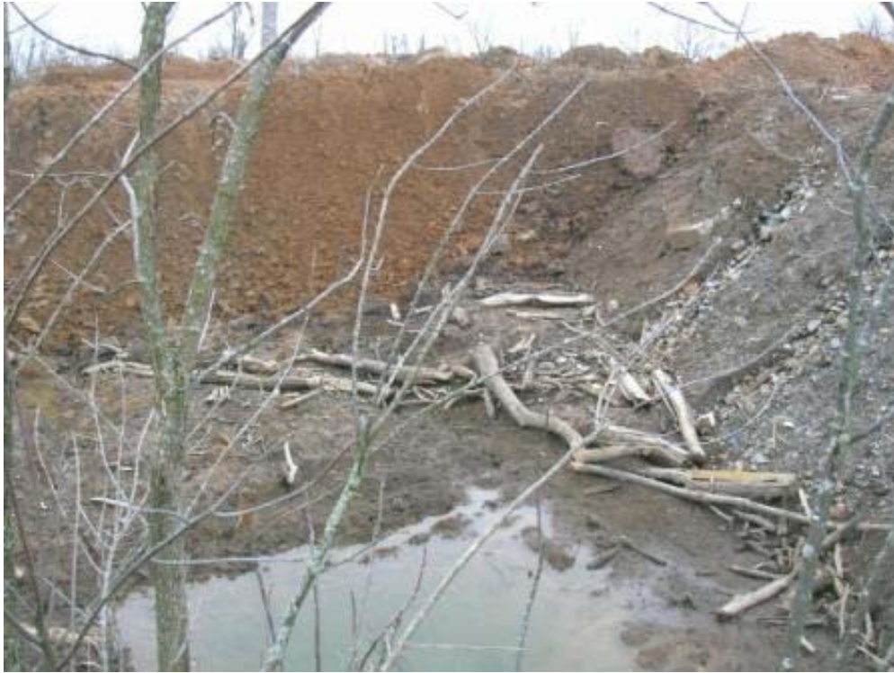
Photo 9: View of the Muncie subsidence being filled in.
