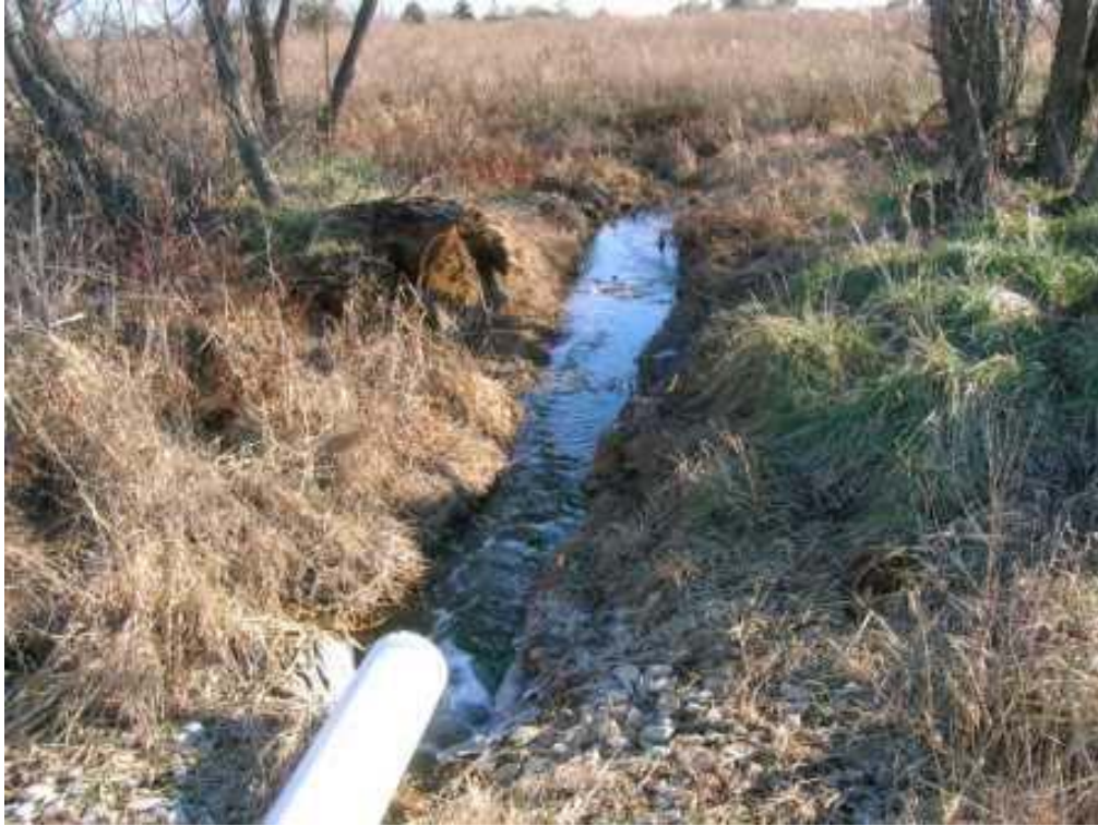
Photo 75: View of discharge water from the constructed wetlands treatment system.
