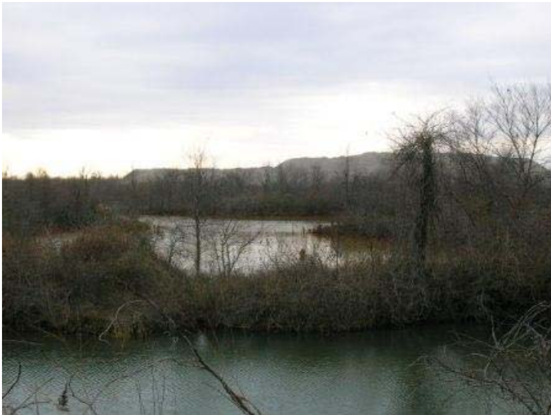
Photo 40: View of water-filled collapse feature on southwest side of Admiralty diversion dike. Water discharges towards the southwest to Tar Creek. View is to the west.
