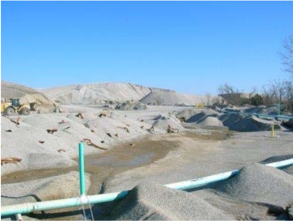
Photo 63: Pipeline used to feed wash-water and washed fine tailings from chat washer to injection well.
