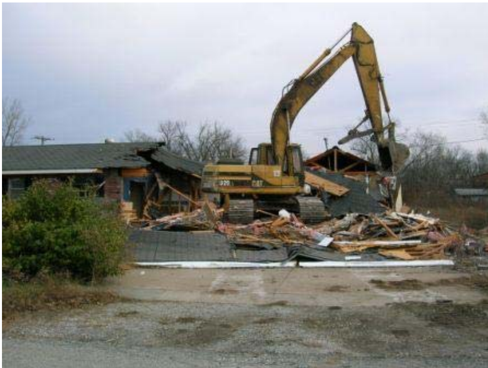
Photo 38: View of home demolition in Picher.
