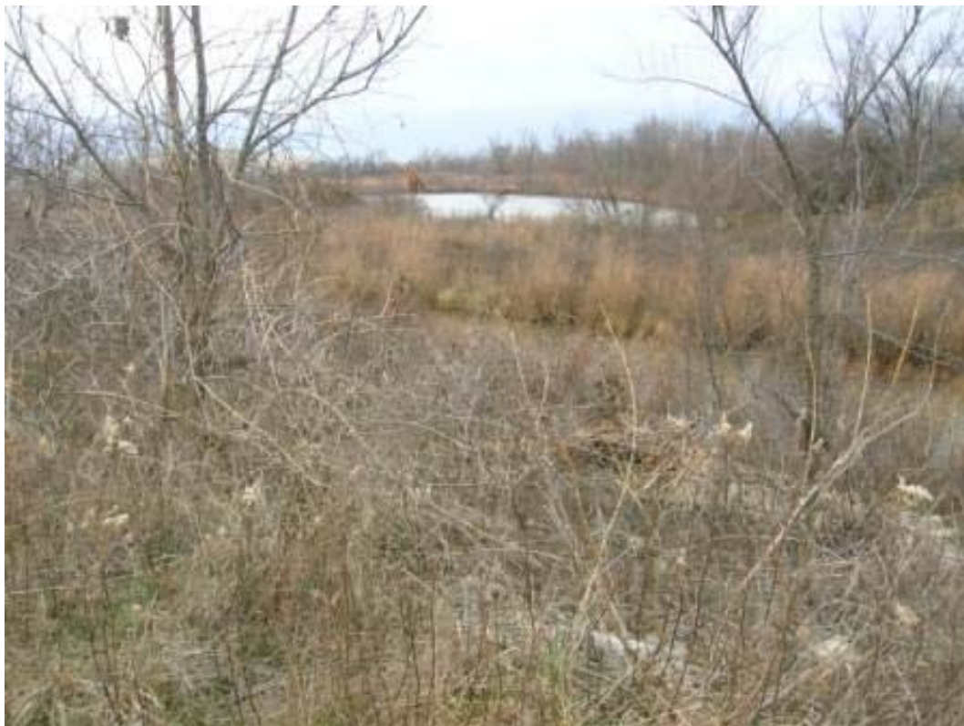
Photo 44: View of diverted Lytle Creek channel from Admiralty diversion dike. View is facing north/northeast.
