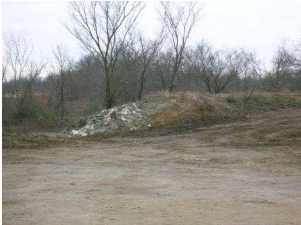
Photo 13: View of breach made in diversion dike at the Muncie site to allow access to fill in the subsidence. View is to the southwest.
