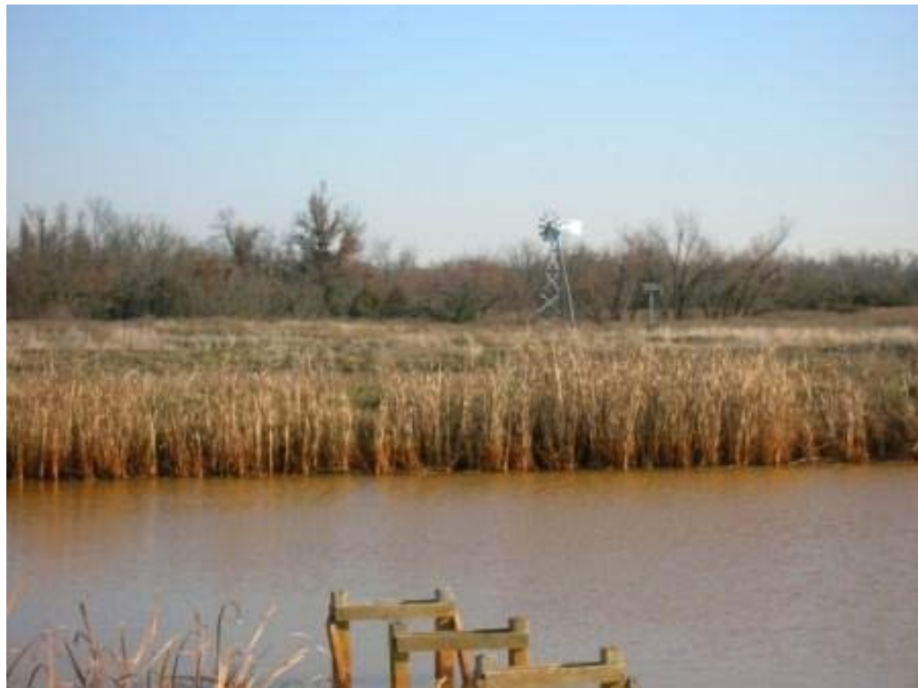
Photo 72: View of iron settling pond and windmill and solar panel at OU's constructed wetlands treatment system at Meyer Ranch. Windmill and solar panel are used to supply electricity. View is facing east.
