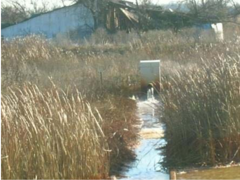
Photo 71: View of mine water flow into the constructed wetlands treatment system at Meyer Ranch.
