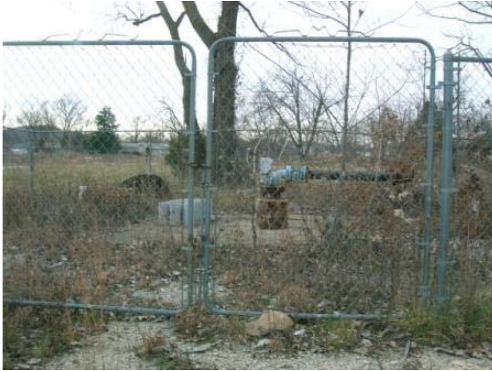
Photo 25: View of Picher Well No. 6-MW. Well is monitored by ODEQ under the Roubidoux Groundwater Monitoring Program.
