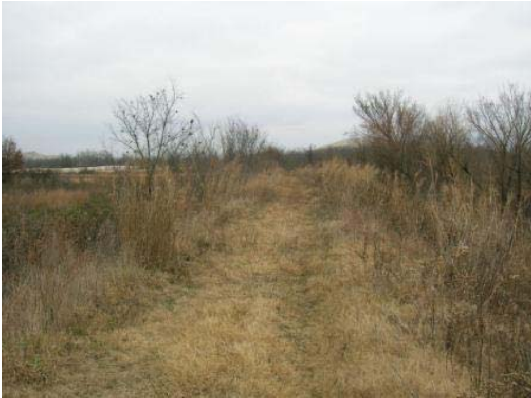
Photo 45: View along top of Admiralty diversion dike. View is facing east.
