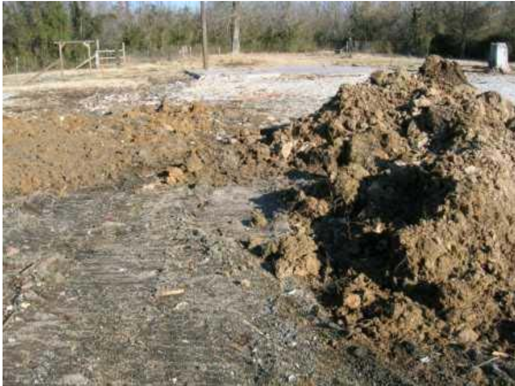
Photo 57: View of chat in building footprint and fill dirt.
