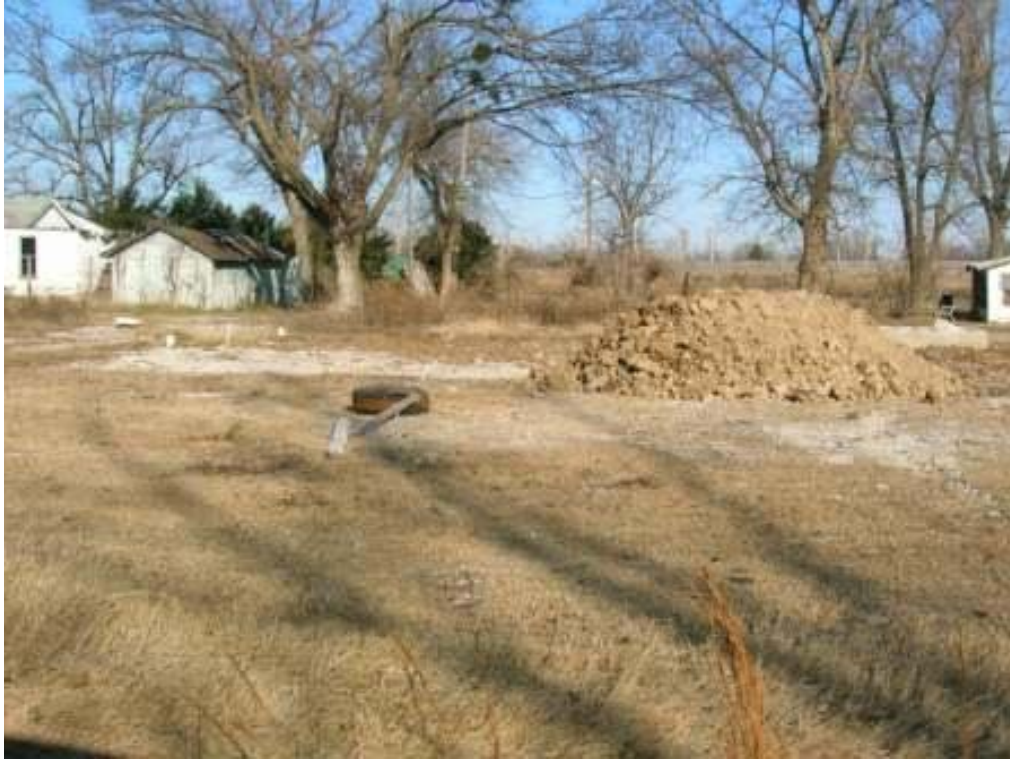
Photo 51: Footprint of home demolished in Picher. Chat is present within the footprint of the home. Fill dirt has been brought in to fill in the depression where the house once sat.
