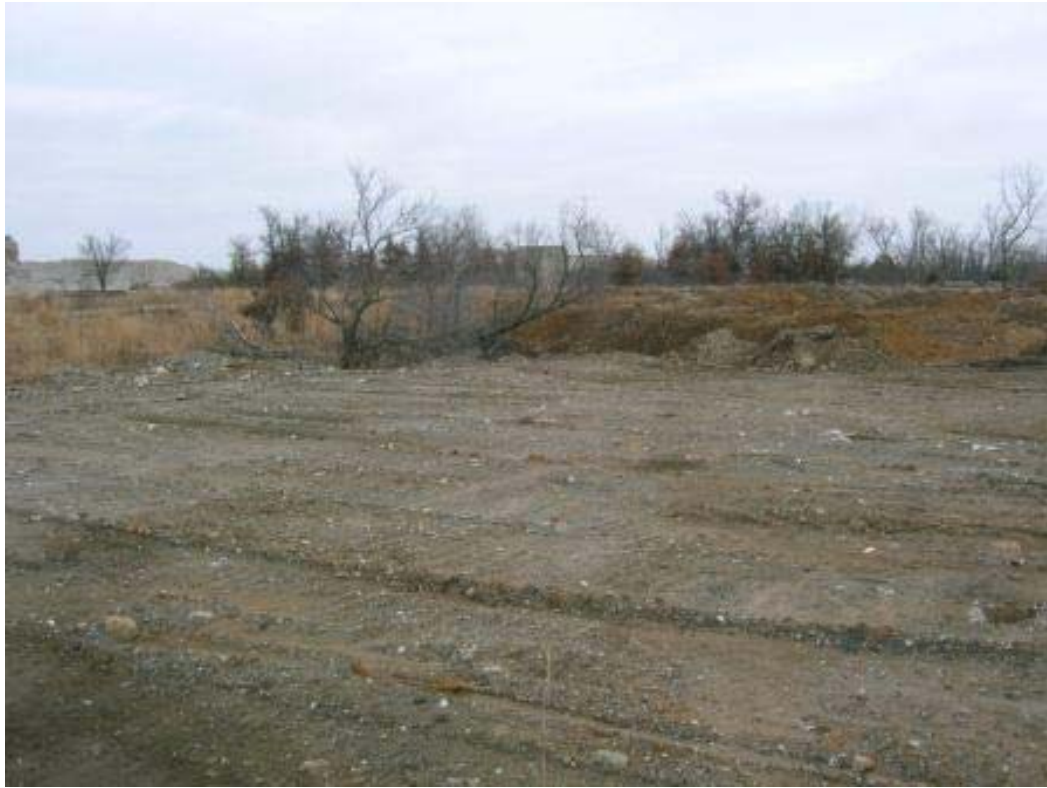
Photo 7: Remediation at the Muncie site in Kansas, being performed for the Treece Subsite of the Cherokee County Superfund Site (EPA Region 7). Depression in the center background is what remains of the Muncie subsidence.
