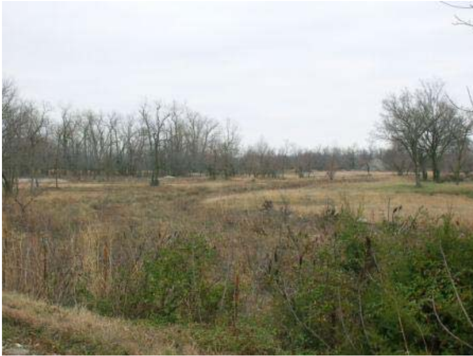
Photo 21: View of channel improvement on Tar Creek tributary west of Tar Creek and northeast of Big John site. Stream channel has been straightened and widened. View is to the southeast.
