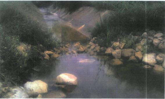
View of rip rap at end of drainage channel showing erosion, view east
