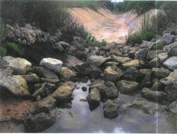
View of rip rap at end of drainage channel showing erosion, view east
