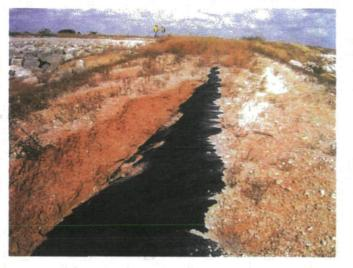
CCND Severe Erosion – Exposed FML
