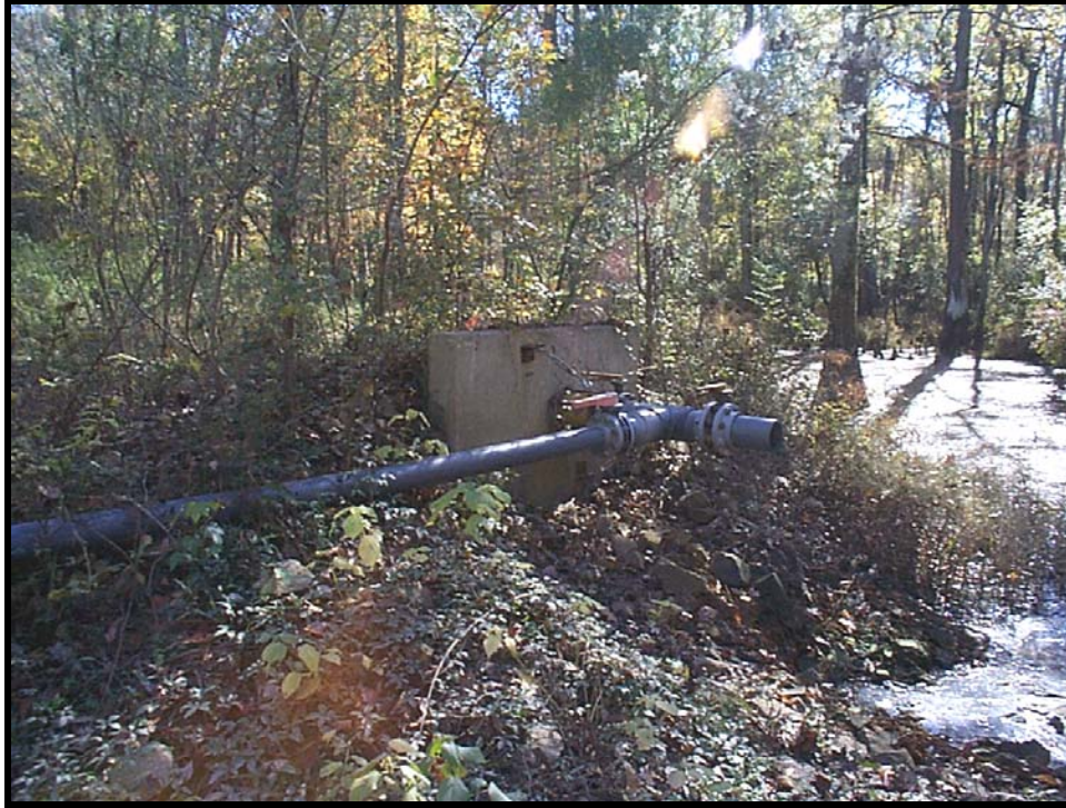
GWTP Outfall at Harrison Bayou
