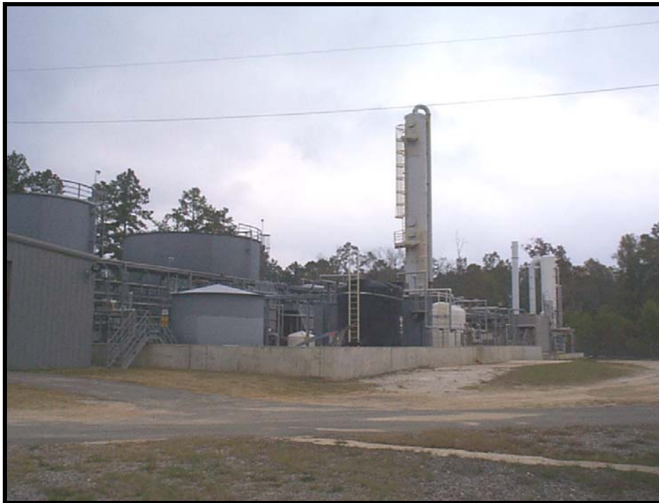
Site 18/24 Groundwater Treatment Plant (From Southwest)
