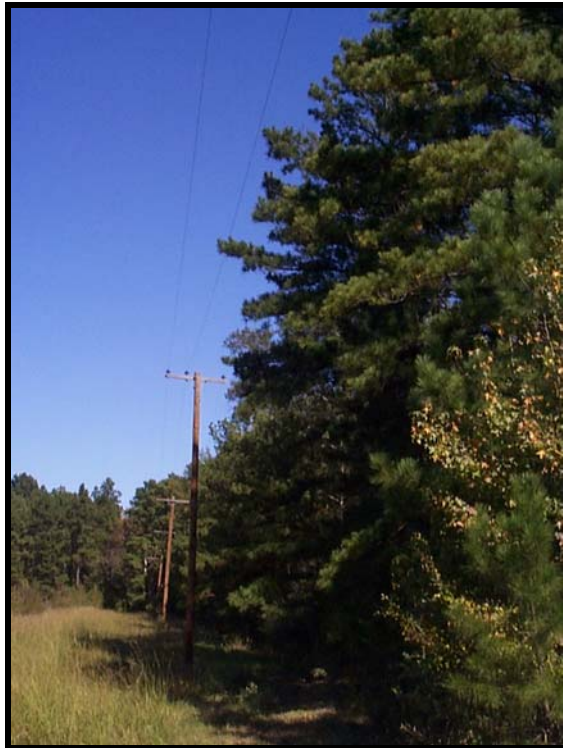
Trees in Electrical ROW at Site 18/24
