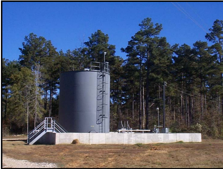
60,000 gallon holding tank at Site 16
