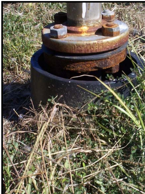
Flange from ICT into Dual Containment Pipe (Some deterioration of carbon steel flange at ground level)
