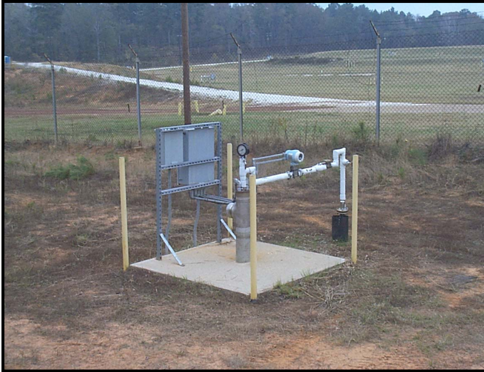
Interceptor Collection Trench Wellhead
