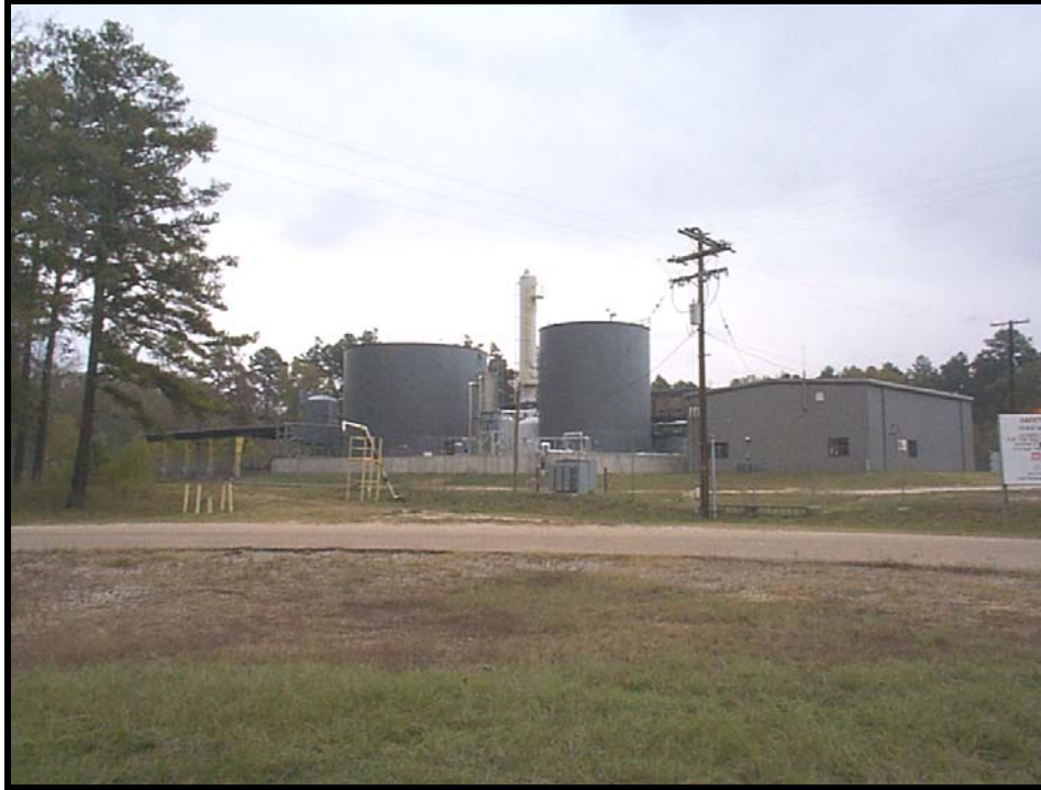
Site 18/24 Groundwater Treatment Plant (From Northwest)
