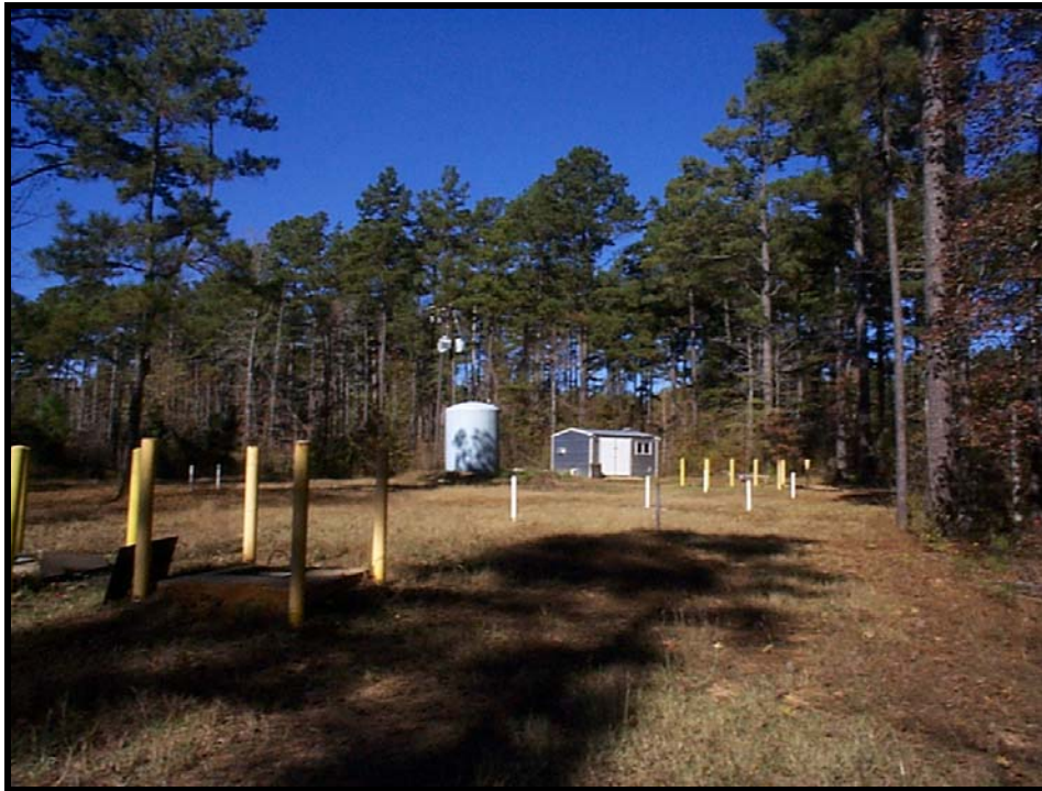
Site 16 Extraction Well System
