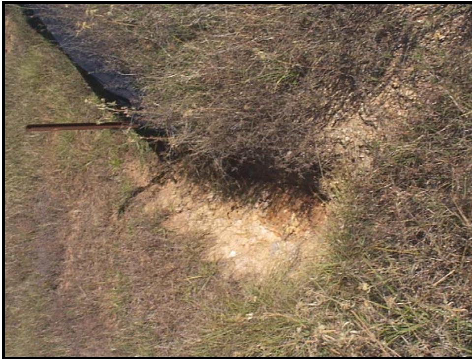
Minor erosion on Site 16 cap
