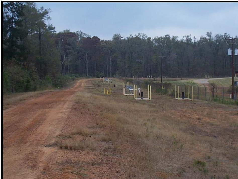
Interceptor Collection Trenches 12-D and 12-E
