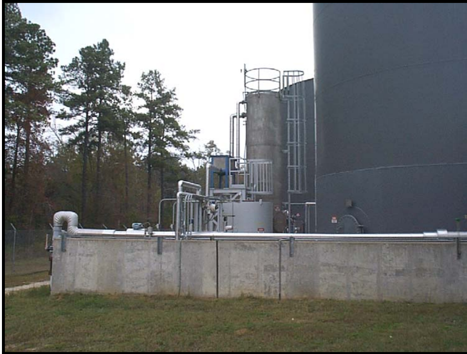
View of Fluidized Bed Reactor at Groundwater Treatment Plant
