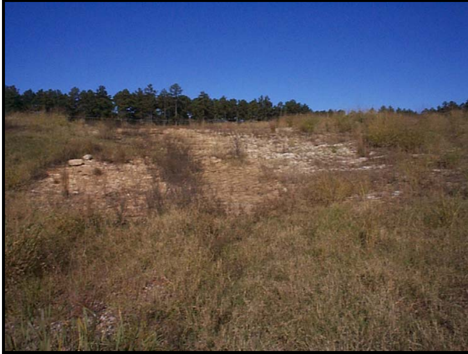
Riprap for erosion control on slope of Site 16
