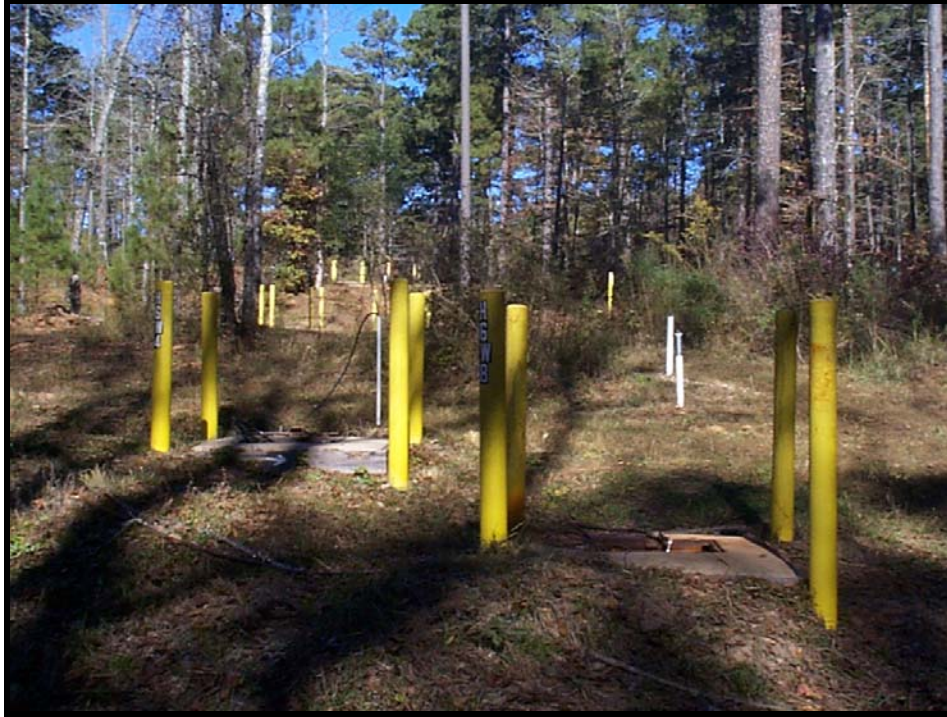
Site 16 Extraction Wells
