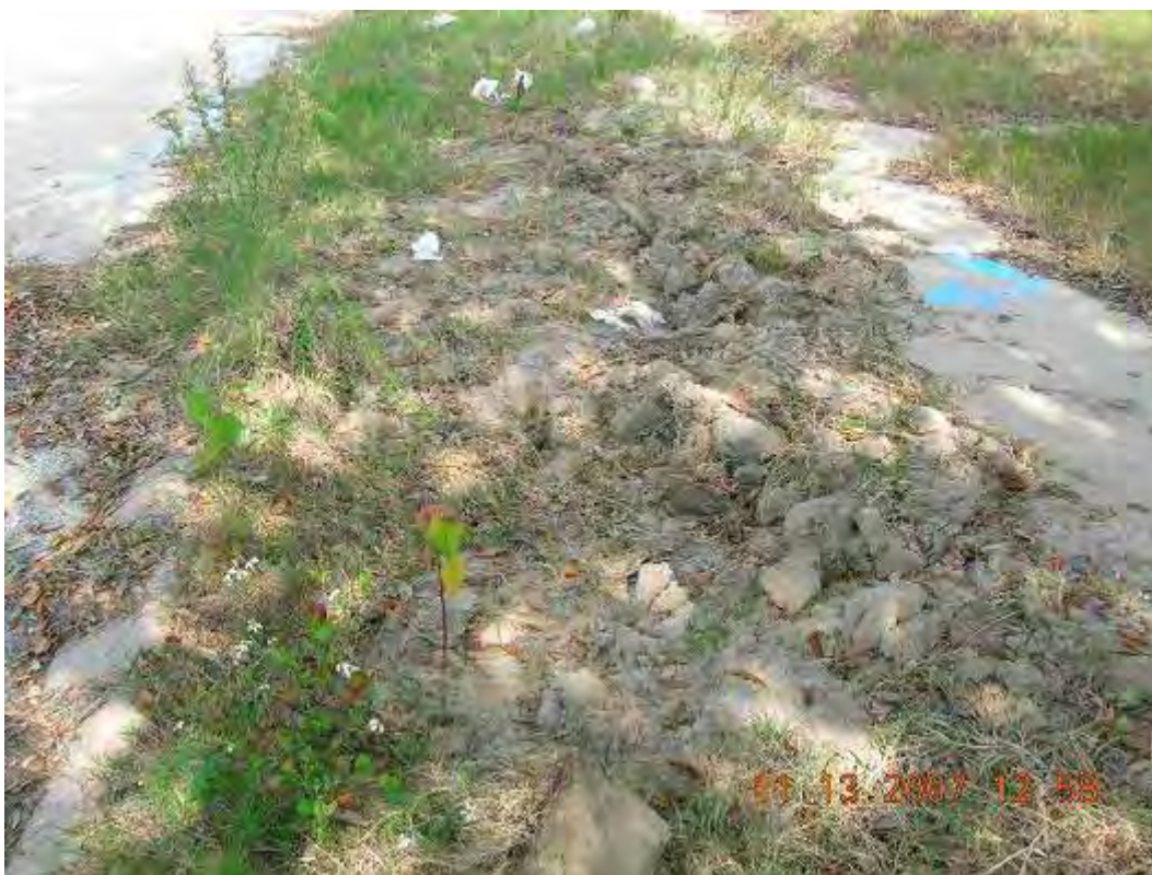
Photo 39: Evidence of digging along the sidewalk at Press Street near the corner of Benefit Street. The geotextile liner was not exposed.
