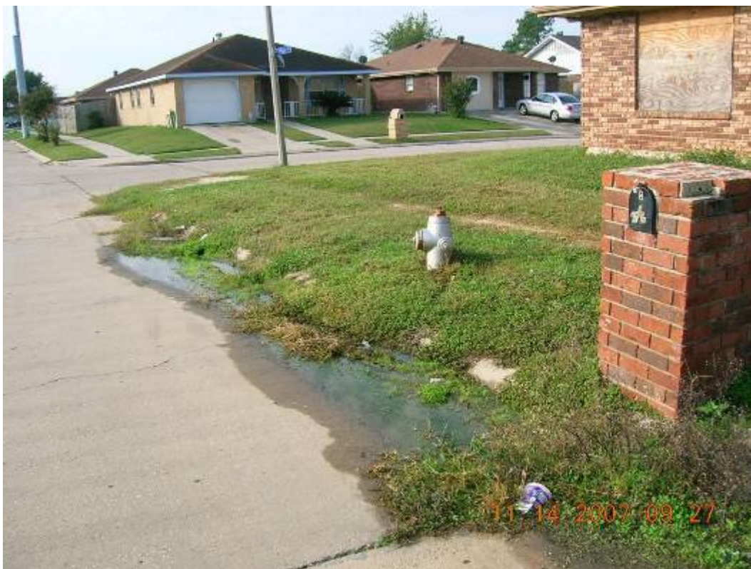
Photo 48: A water leak apparently from a fire hydrant. View is to the south at the corner of Press Street and Benefit Street.
