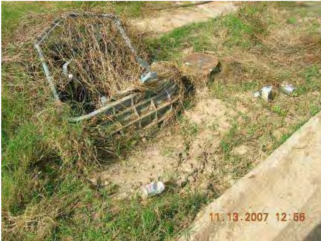
Photo 38: View of an excavated area near a water main line at Press Street. The geotextile liner was not exposed.
