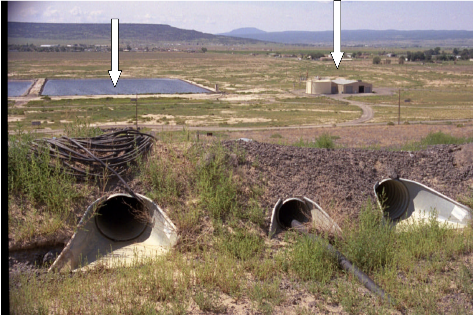
View south at top of southern slope of large tailings pile, showing runoff drainage pipes. Note west collection ponds and reverse osmosis plant (left and right arrows, respectively) Residential community is visible in background.
