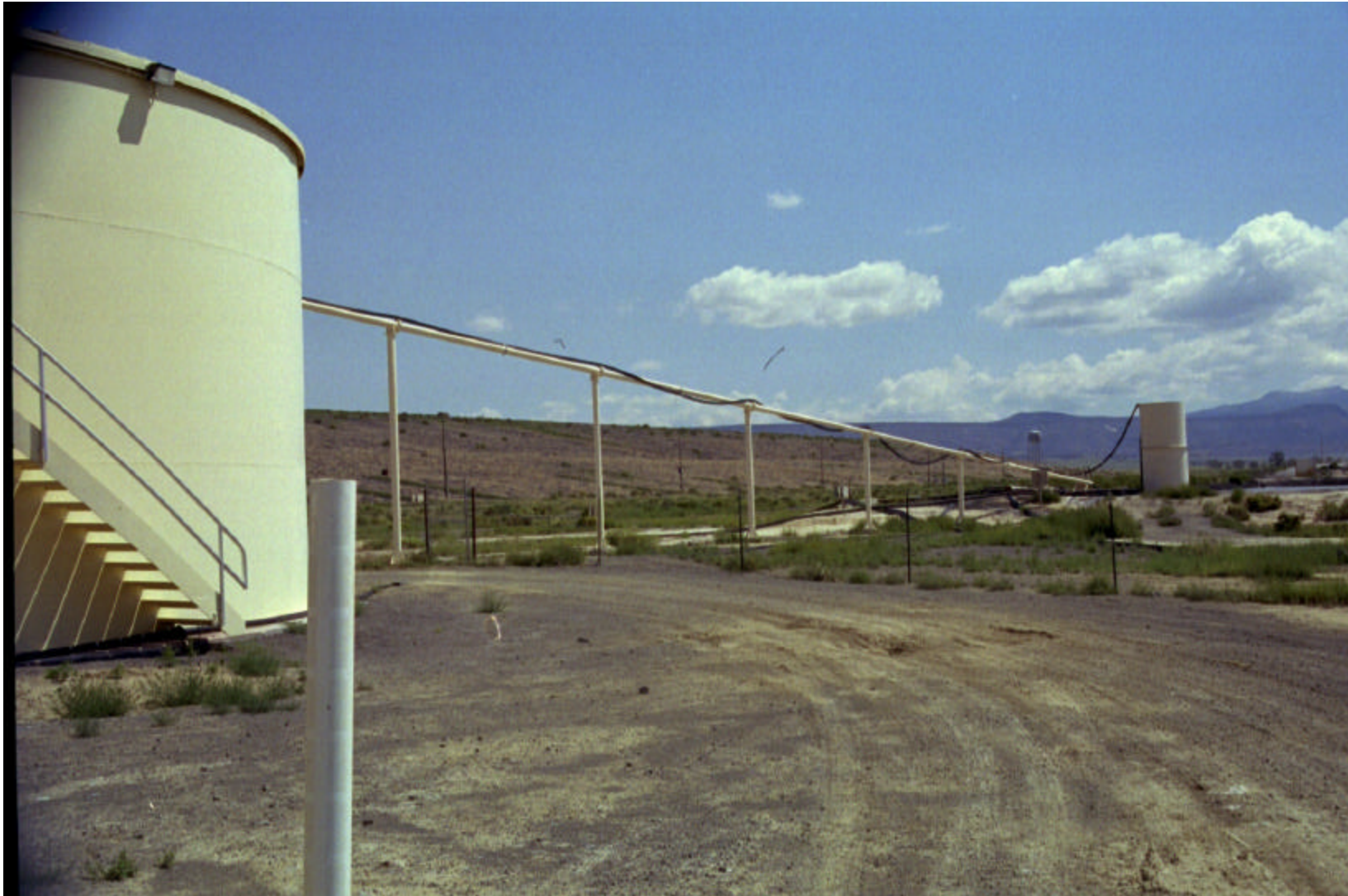
Exterior of reverse osmosis plant, showing conveyance between plant and evaporation ponds to right of view. Facing north-northwest.
