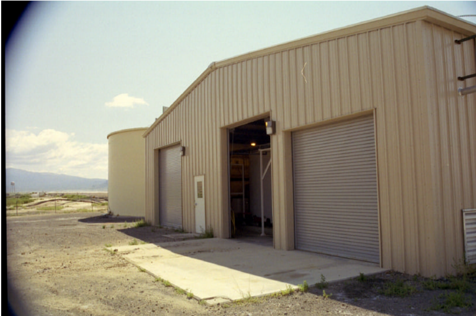
Exterior of reverse osmosis plant, facing east-southeast.
