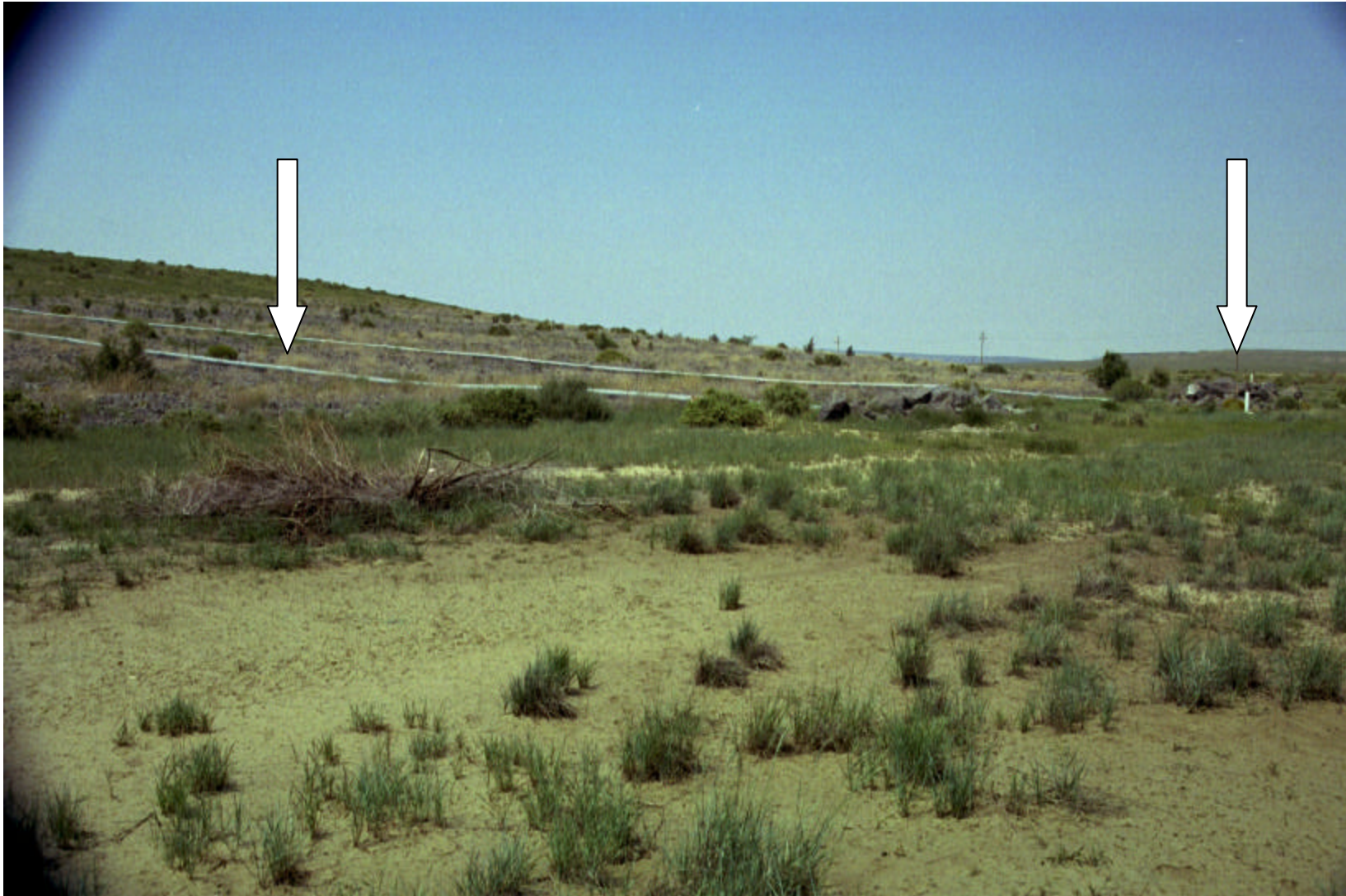
To right of previous view. Asbestos disposal area is left of view; runoff conveyance from top of large tailings pile is visible at left white arrow. Right white arrow shows runoff discharge point, which uses boulders to break flow.
