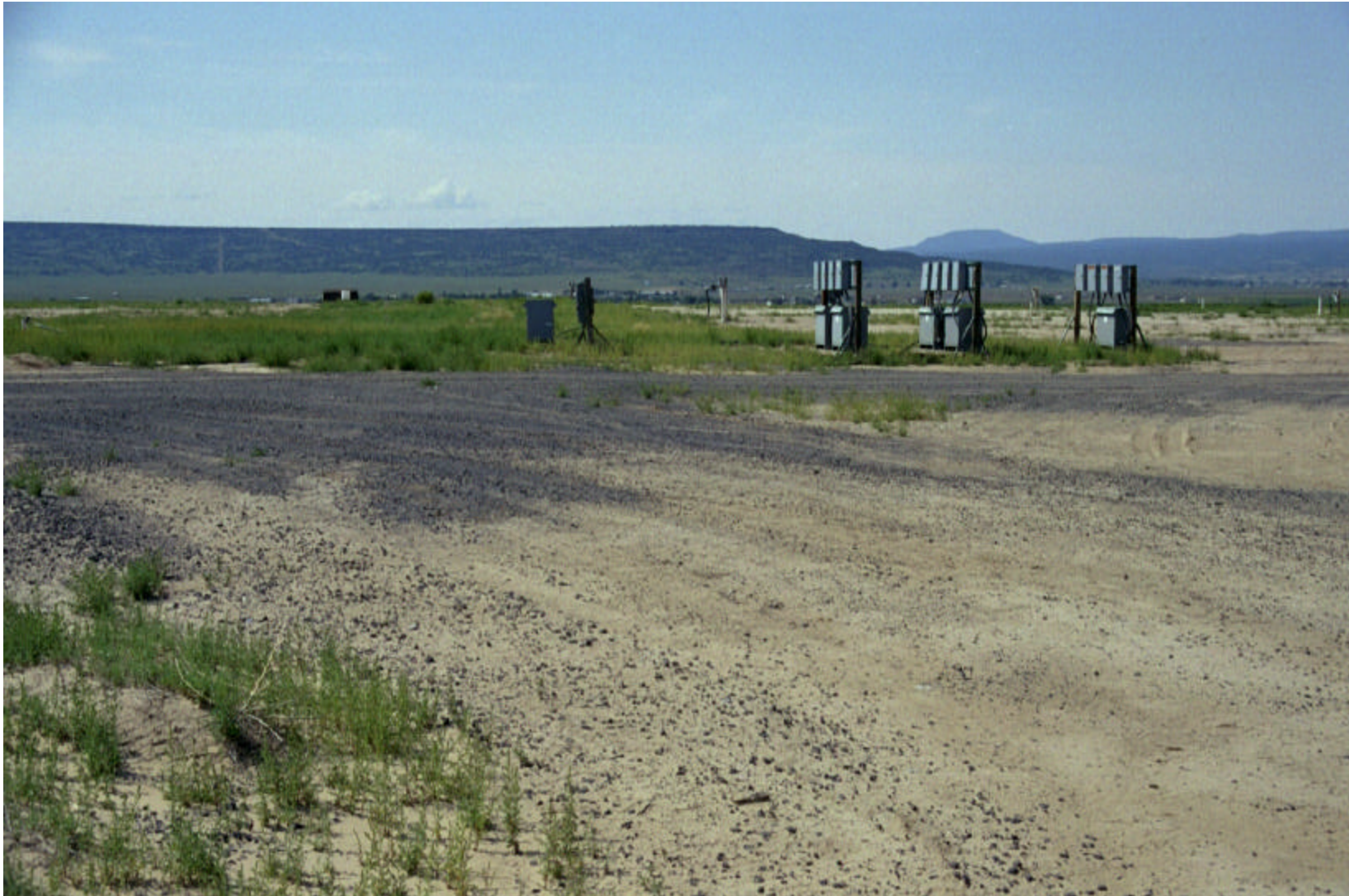
Facing south across large tailings pile temporary cover. Structures visible are the electrical boxes for the tailings pile dewatering well system.
