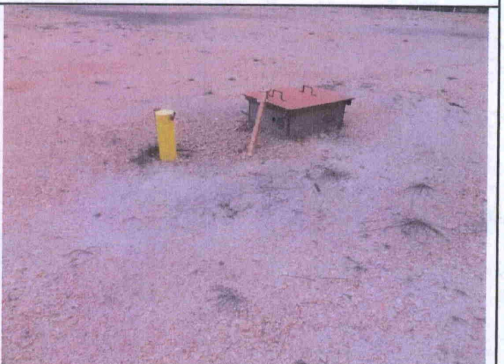
10 – Cap, Not in service extraction well
