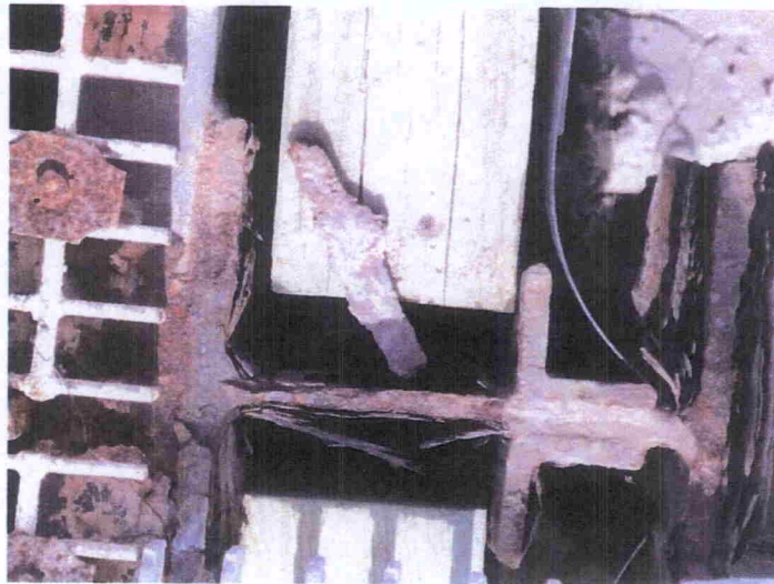
North Decant Structure Corrosion
