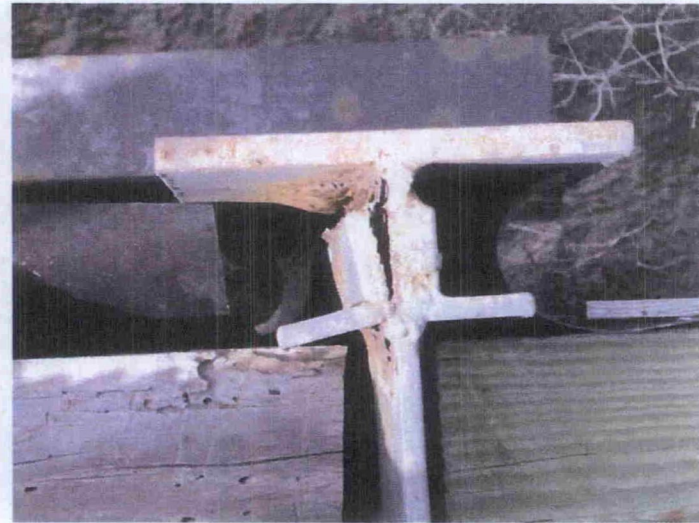
South Decant Structure Corrosion
