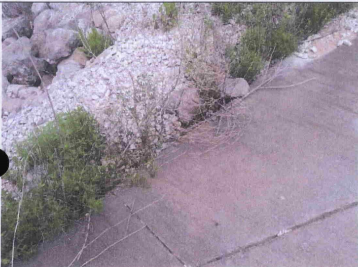
27 – Emergency Spillway, viewing minor washout
