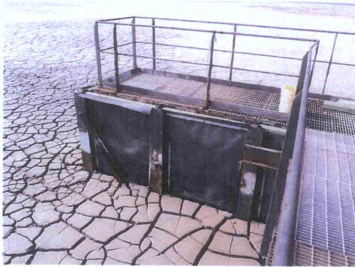
North Decant Structure Corrosion
