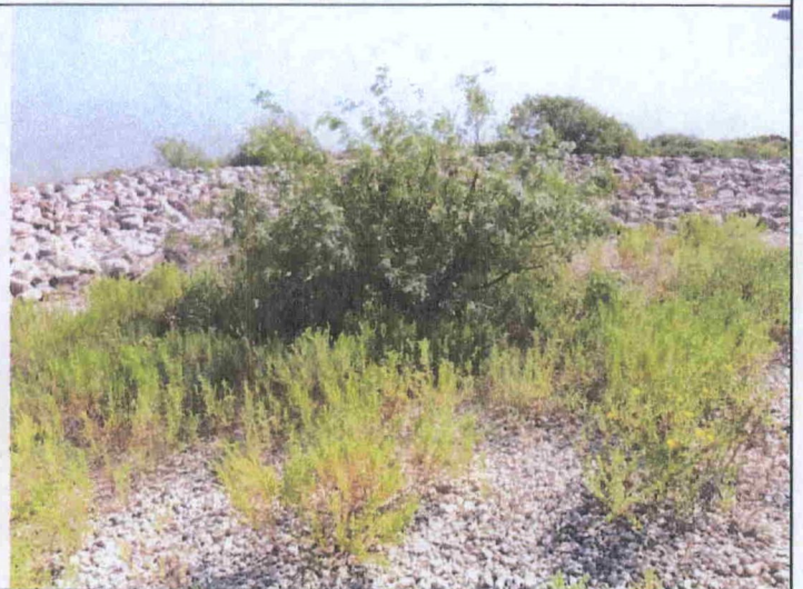
12 –Intrusive trees and vegetation in exterior gravel protection
