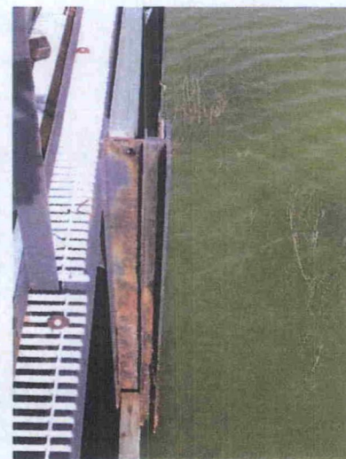
South Decant Structure Corrosion
