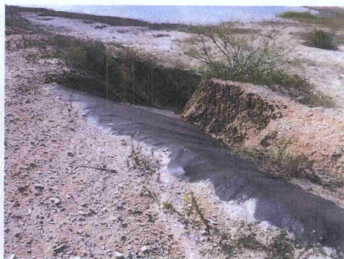
CCND Water Stop FML Exposed, Erosion (previously noted)
