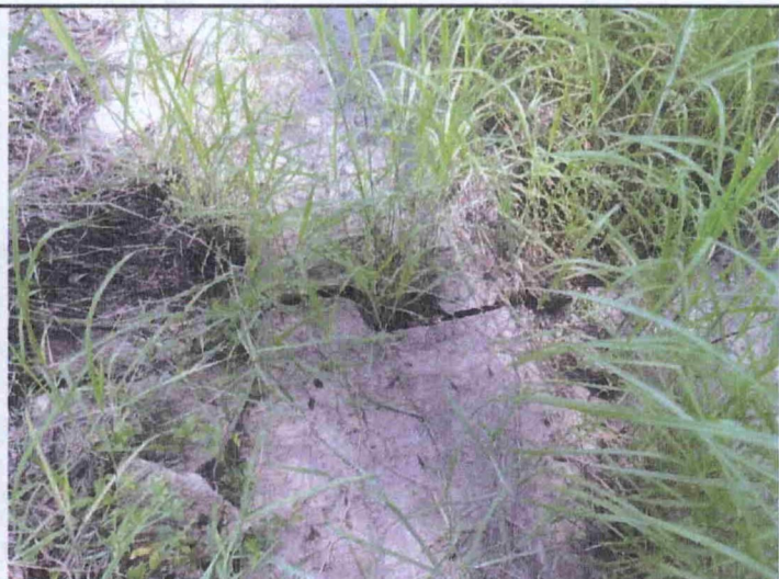
16 - View of vegetation growing through old portions of the drainage channel
