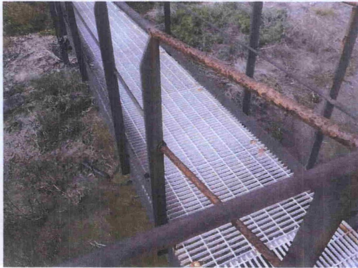
South Decant Structure Corrosion
