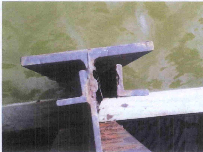
South Decant Structure Corrosion
