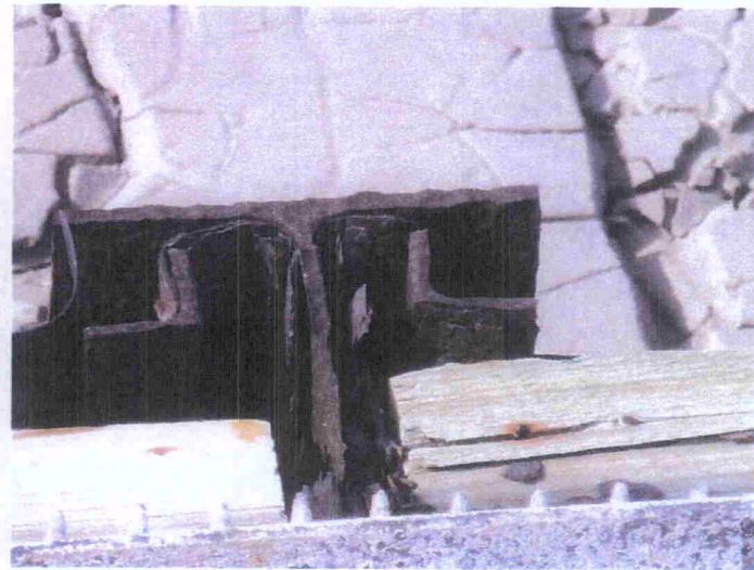
North Decant Structure Corrosion
