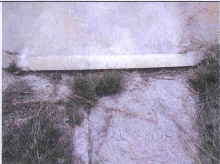
14 - View of erosion at lip of drainage channel
