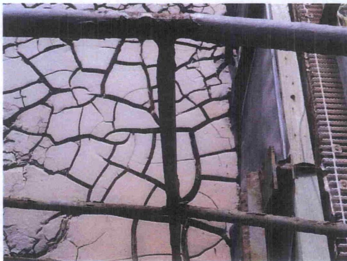
North Decant Structure Corrosion
