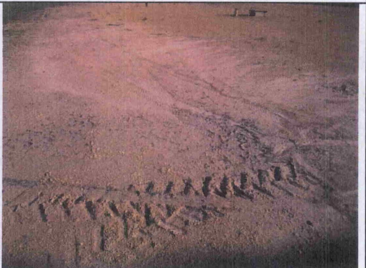
12 – Cap, Ruts from mowing of ditches
