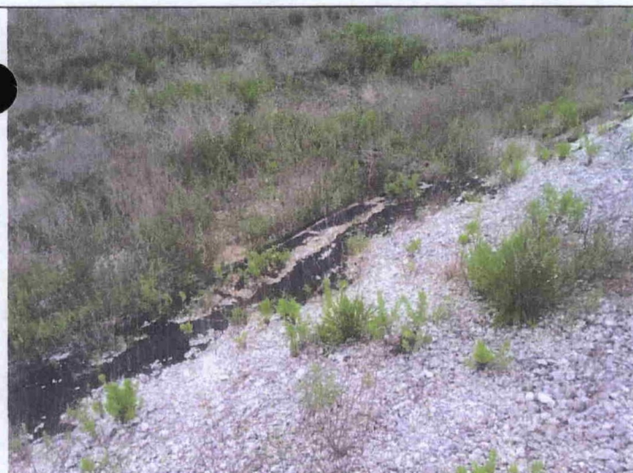
19 – South Dike, viewing exposed geomembrane
