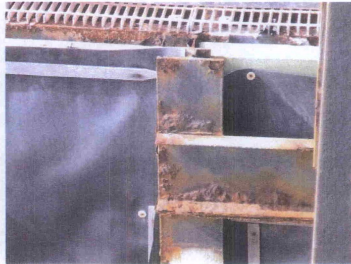
North Decant Structure Corrosion
