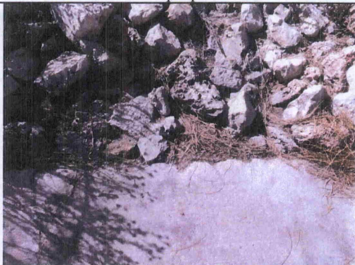
16 - View of minor movement of rip rap at the end of the drainage channel
