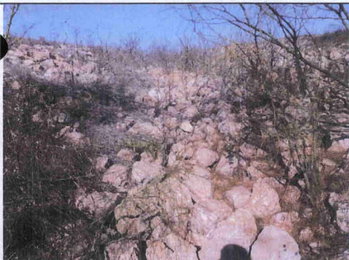
13 - View of vegetation in drainage rip rap from drainage channel
