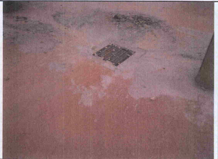
2 - Cap, storm sewer drain at R-301
