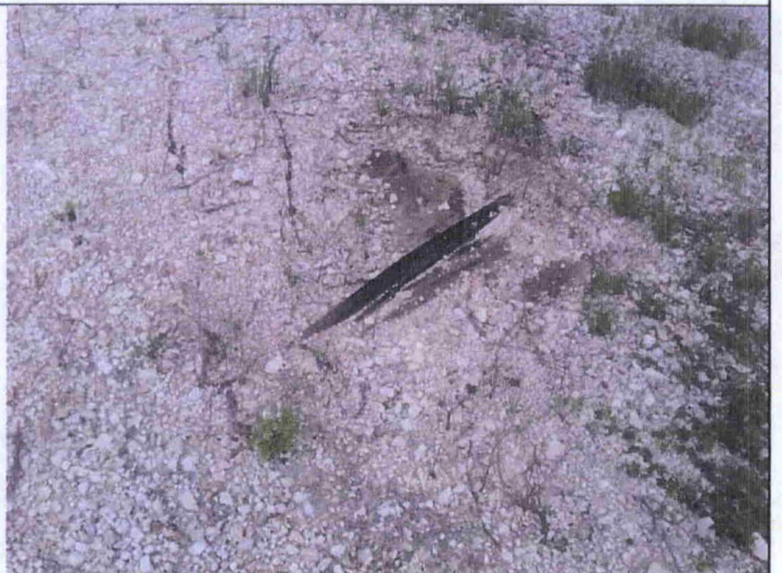
37 – Viewing tear of the geomembrane in the road
