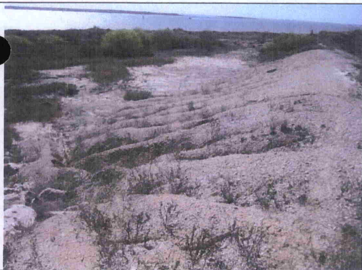
31 – East CPA Outer Dike, viewing erosion rills
