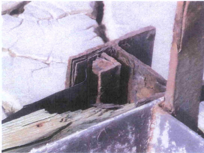
North Decant Structure Corrosion
