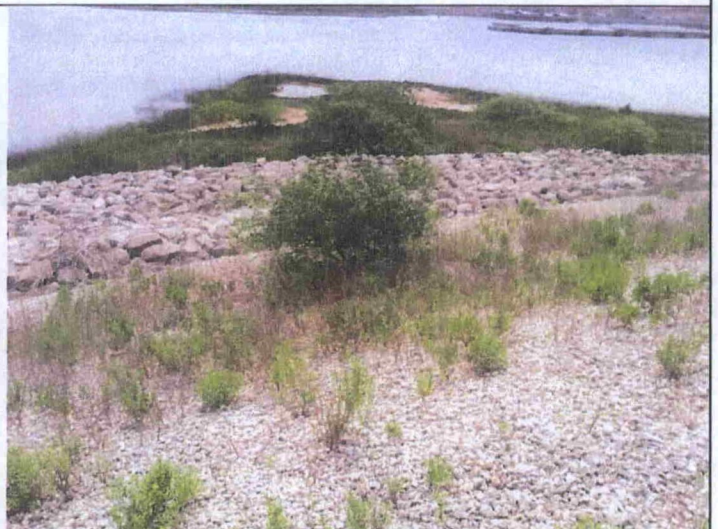
12 – Intrusive trees and vegetation in exterior gravel
