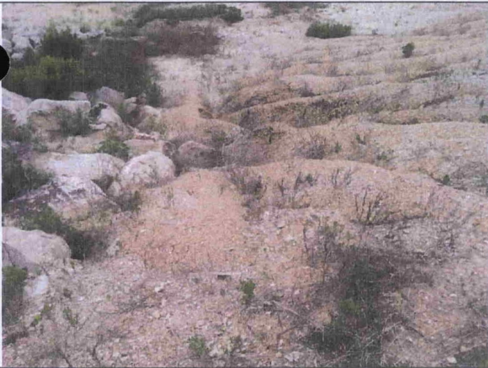
31 – East CPA Outer Dike, viewing erosion rills
