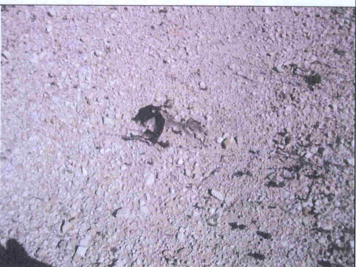
37 – Viewing tear of the geofabric in the road
