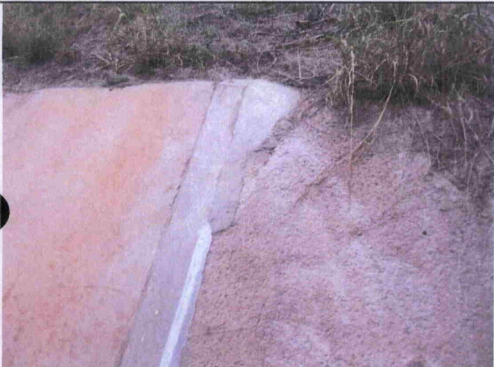
15 - View of repaired sidewall of drainage channel
