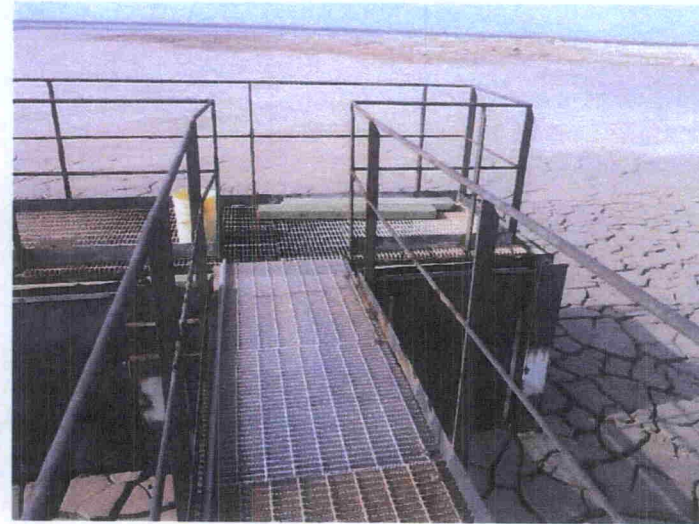
North Decant Structure Corrosion
