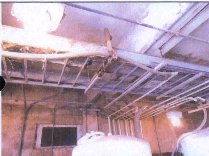
15 – Building, viewing rusted support structure
