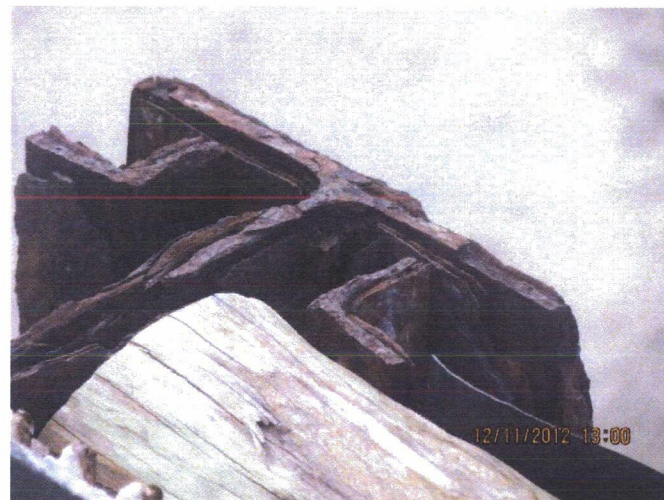
North Decant Structure Corrosion
