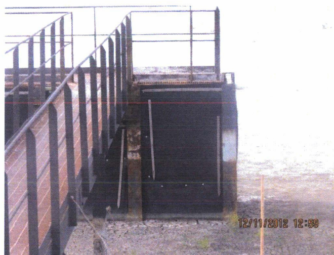
North Decant Structure Corrosion
