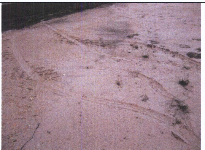
12 – Cap, Ruts from mowing of ditches
