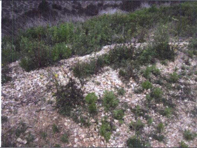
13 – Intrusive vegetation in Gravel Protection
