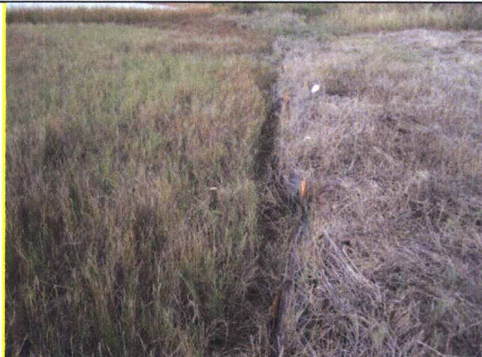
7 – Silt fence between the tank farm slope and drainage channel
