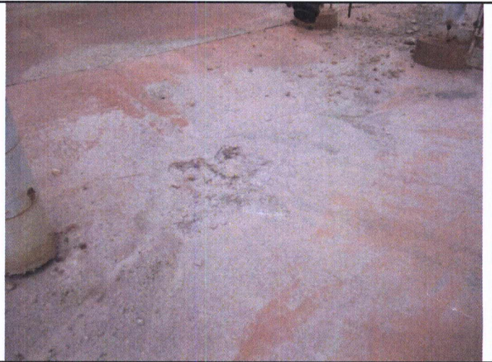
2 - Cap, storm sewer drain at R-301
