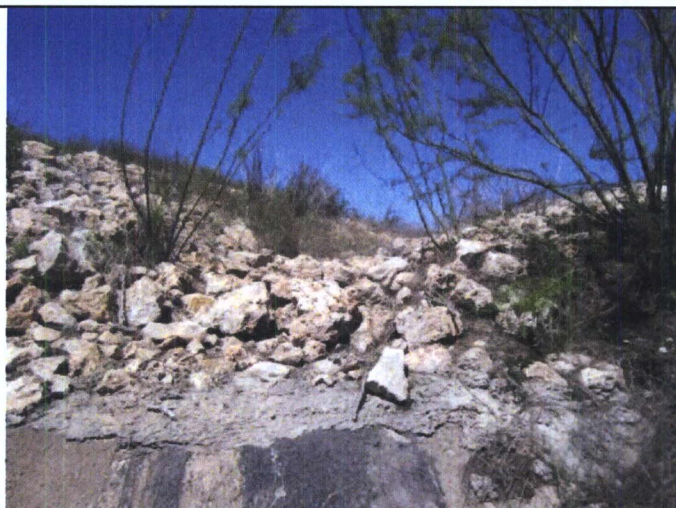
13 - View of rip rap at drainage from drainage channel
