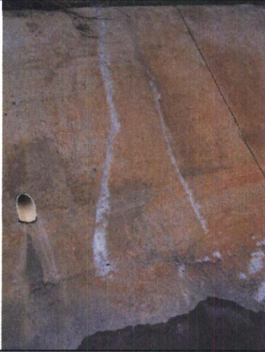
7 – Deterioration (marks) on the concrete within the drainage channel
