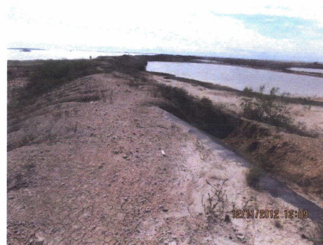
CCND Severe Erosion – Exposed FML
