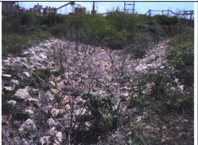
12 - View of rip rap at drainage from tank farm cap
