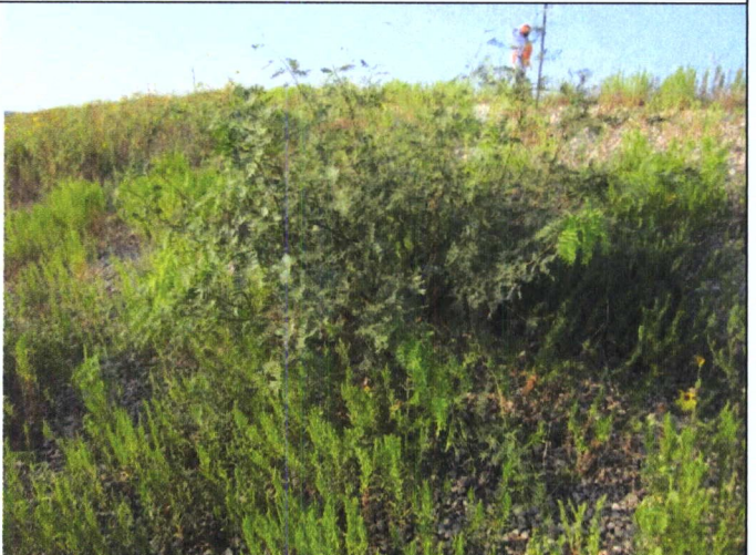
12 –Intrusive Trees and Vegetation in Gravel Protection
