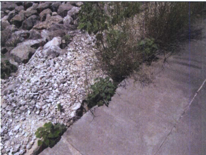
27 – Emergency Spillway, viewing minor washout
