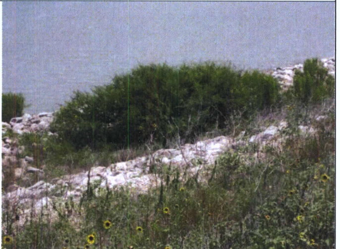
12 –Intrusive Trees in Storm Protection
