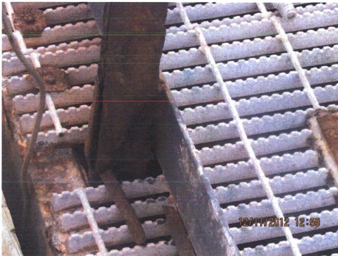
North Decant Structure Corrosion
