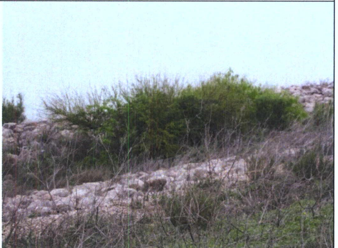
12 –Intrusive Trees in Storm Protection
