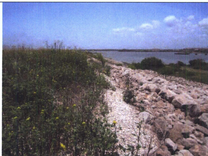
13 – Intrusive vegetation in Gravel Protection
