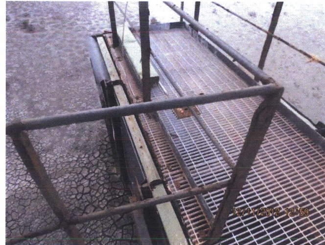
North Decant Structure Corrosion
