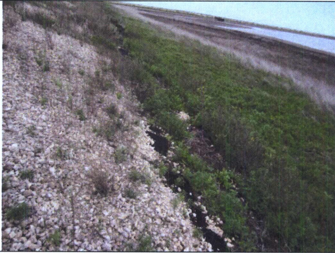
19 – South Dike, viewing exposed geofabric
