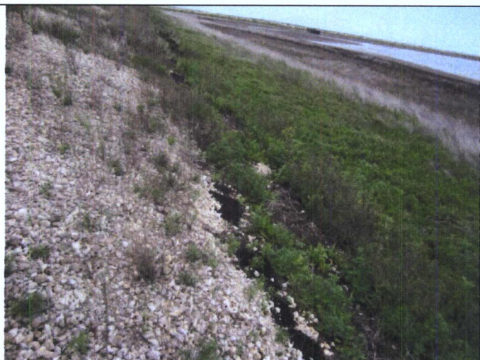
19 – South Dike, viewing exposed geofabric
