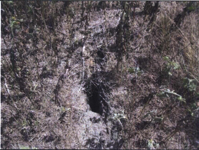
15 - View of large cracking in the slope
