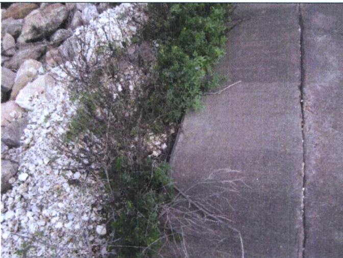
27 – Emergency Spillway, viewing minor washout
