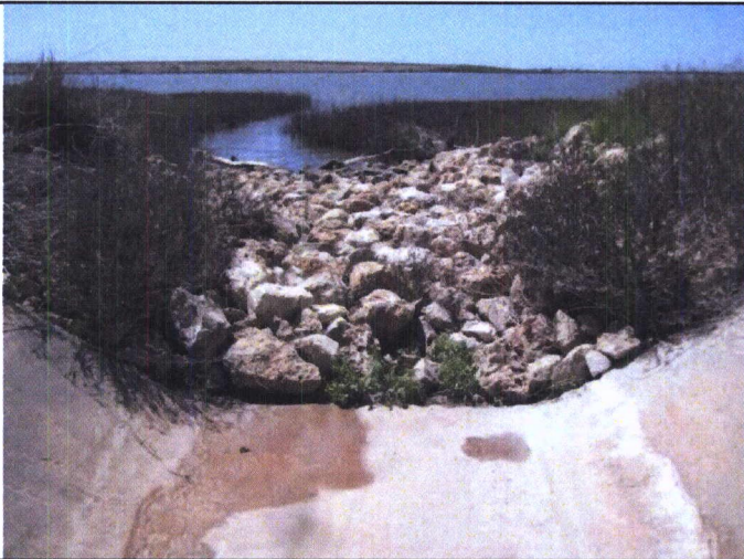
9 - View of rip rap damage at the end of the drainage channel
