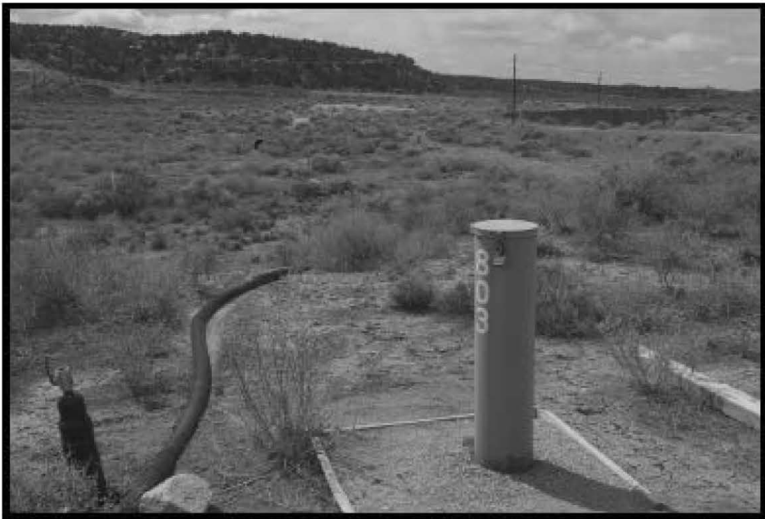
Photograph 10. View of Southwest Alluvium extraction-monitoring well No. 803 at south end of UNC Mill Site evaporative tailings pond disposal area. Well has not been used for extraction since 1999.
