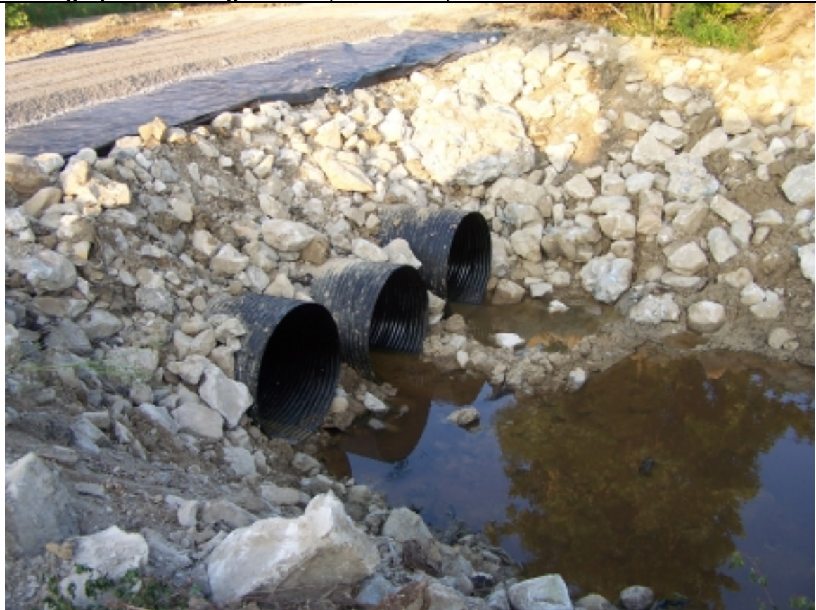
Photograph 28 – Bridge Construction, Scenic OU, Southwest 6/1/10
