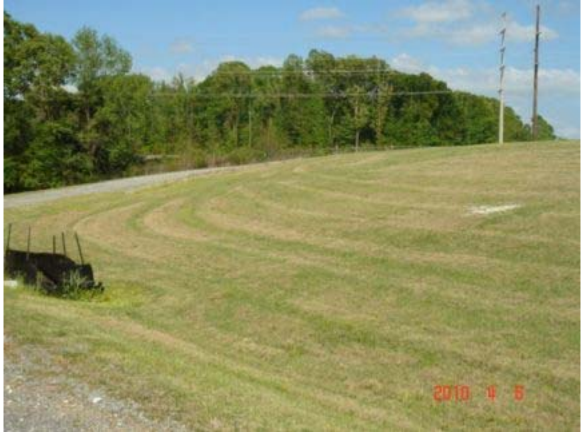
Photograph 22 – Covered Disposal Area, Scenic OU, Northeast 4/6/10
