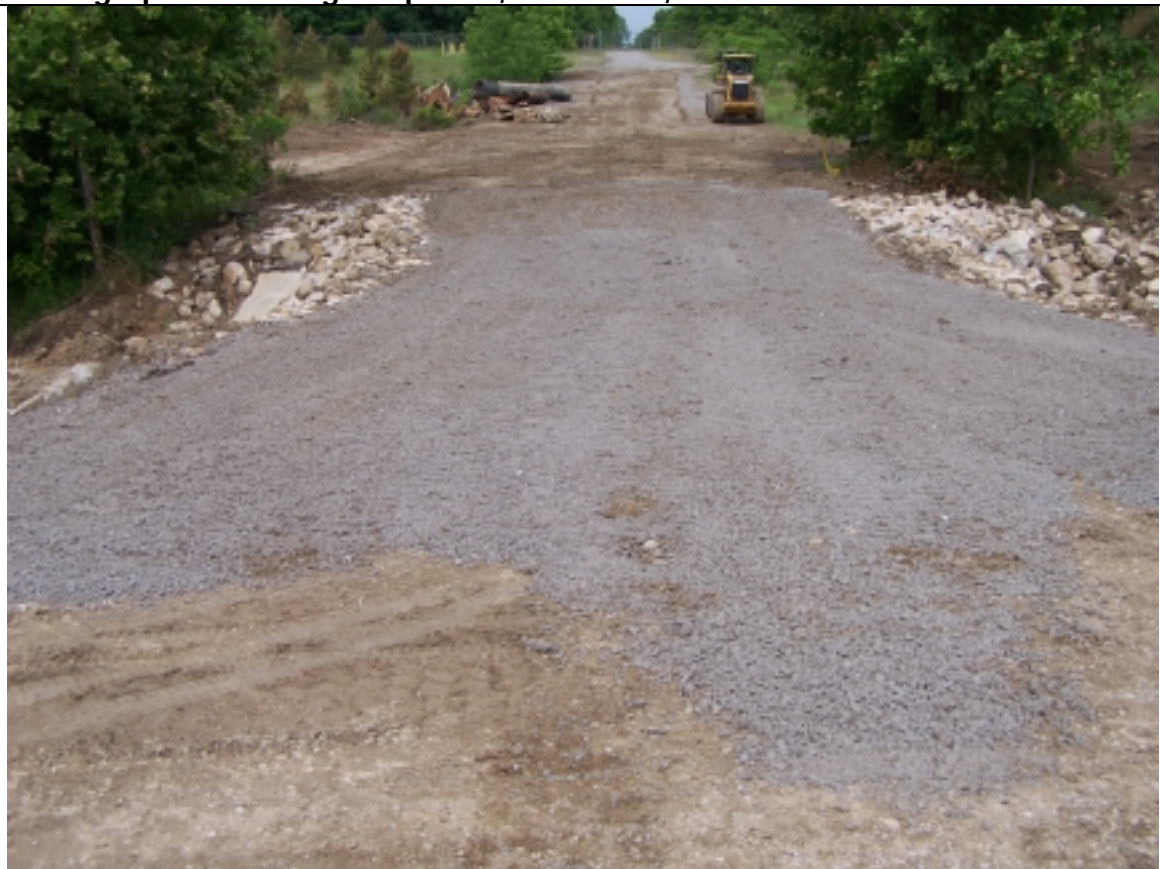
Photograph 30 – Bridge Repaired, Scenic OU, West 6/3/10
