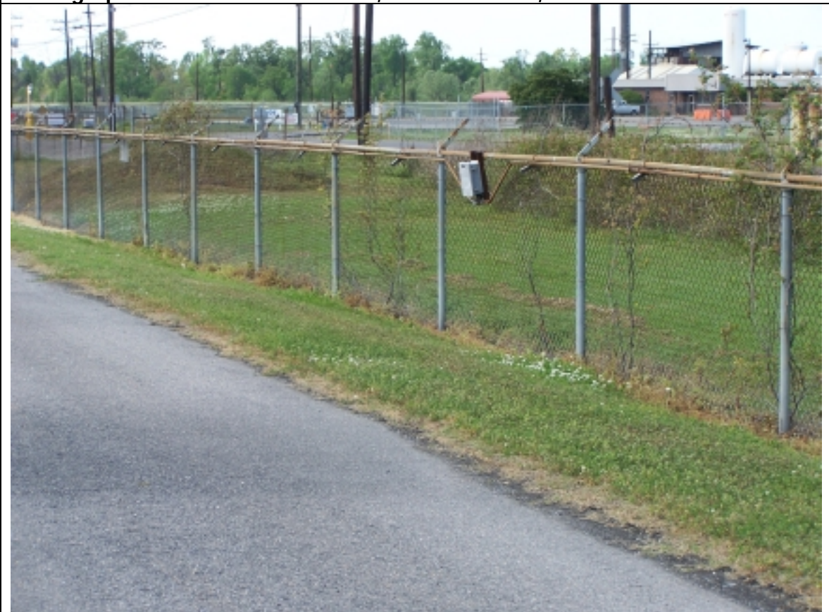
Photograph 12 – North Perimeter Fence, Brooklawn OU, Northwest 4/6/10
