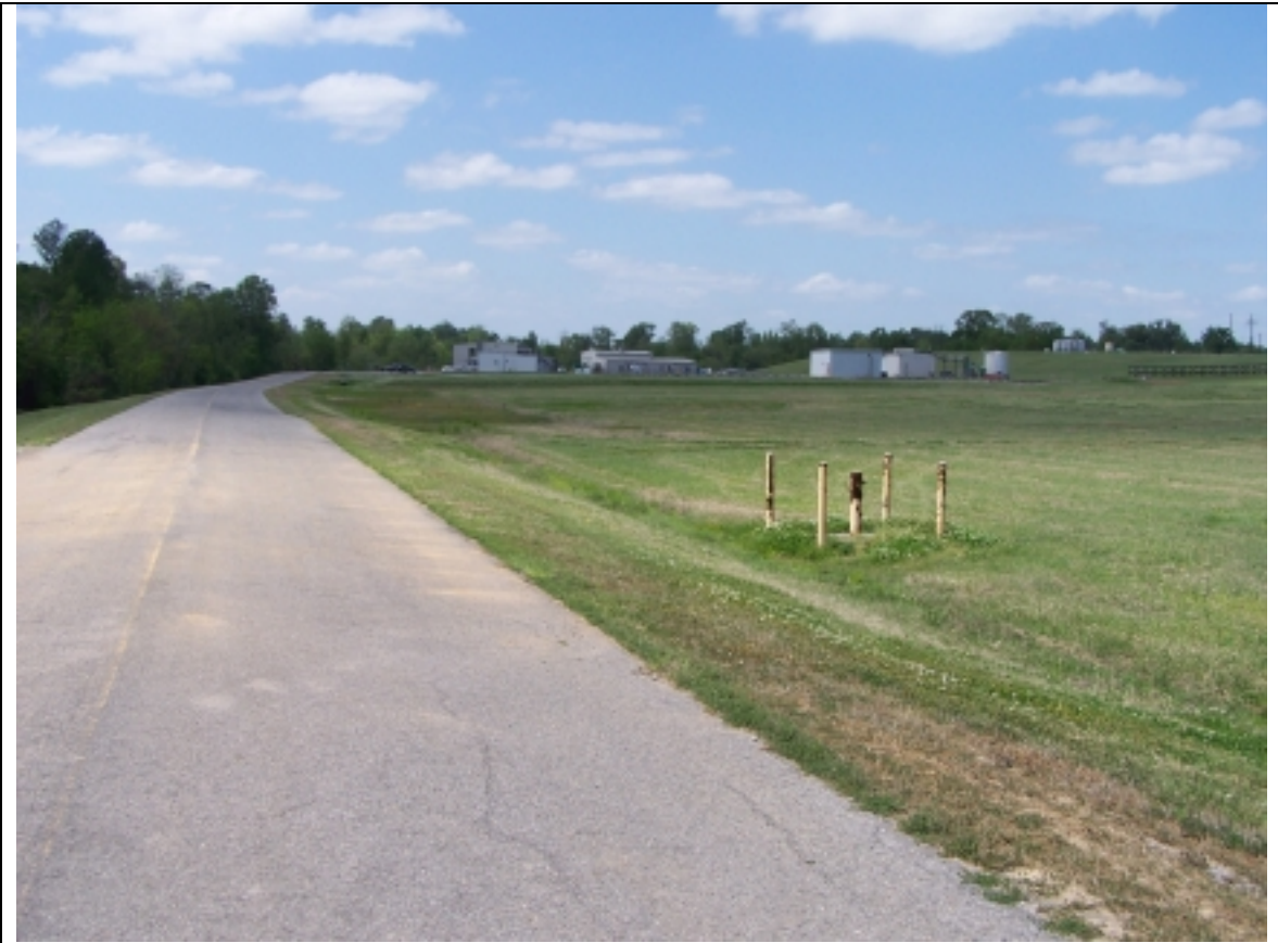
Photograph 11 – South Levee Road, Brooklawn OU, West 4/6/10
