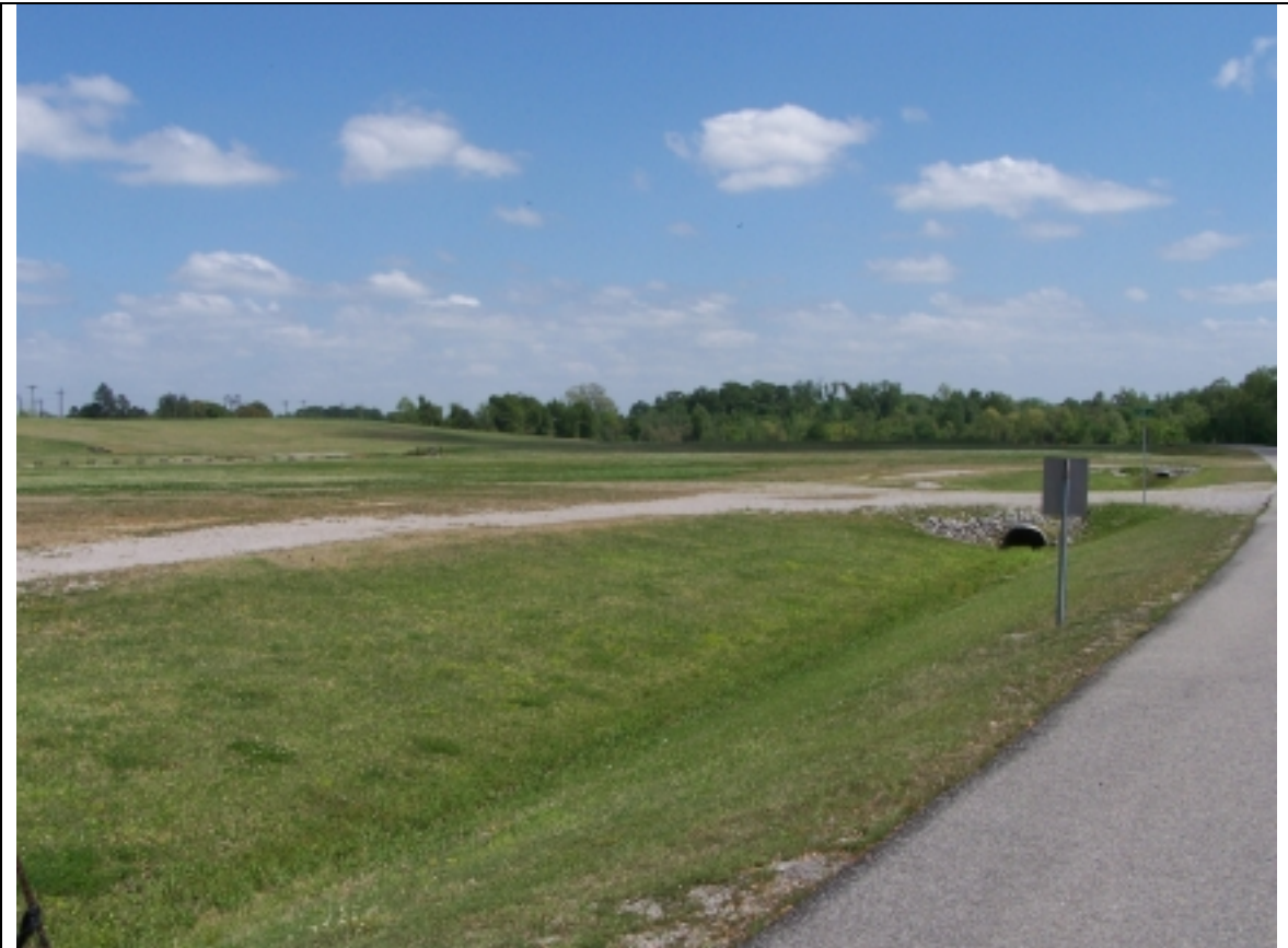
Photograph 9 – South Levee Road, Brooklawn OU, East 4/6/10
