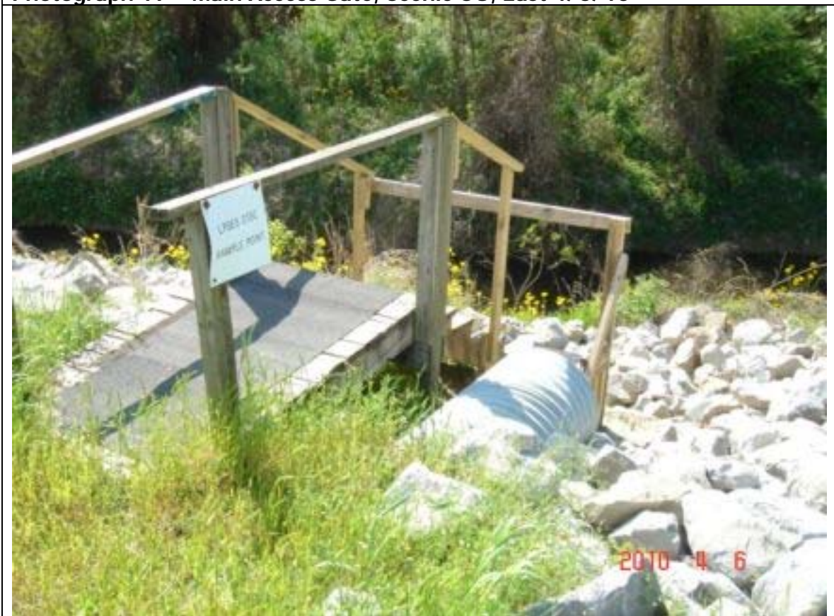
Photograph 20 – LPDES Outfall 013C, Scenic OU, East 4/6/10
