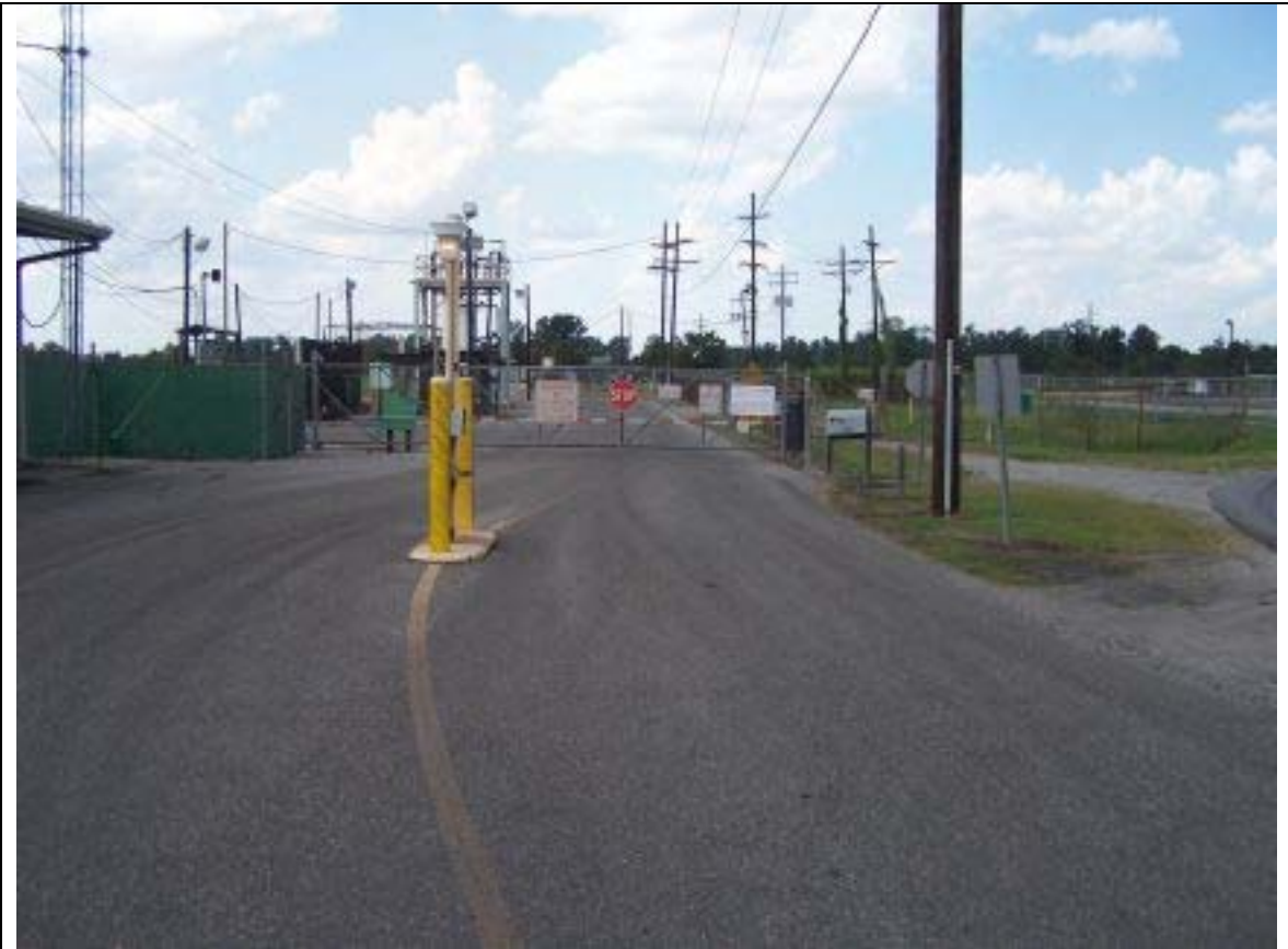
Photograph 1 – Main Access Gate, Brooklawn OU. West, 9/22/10
