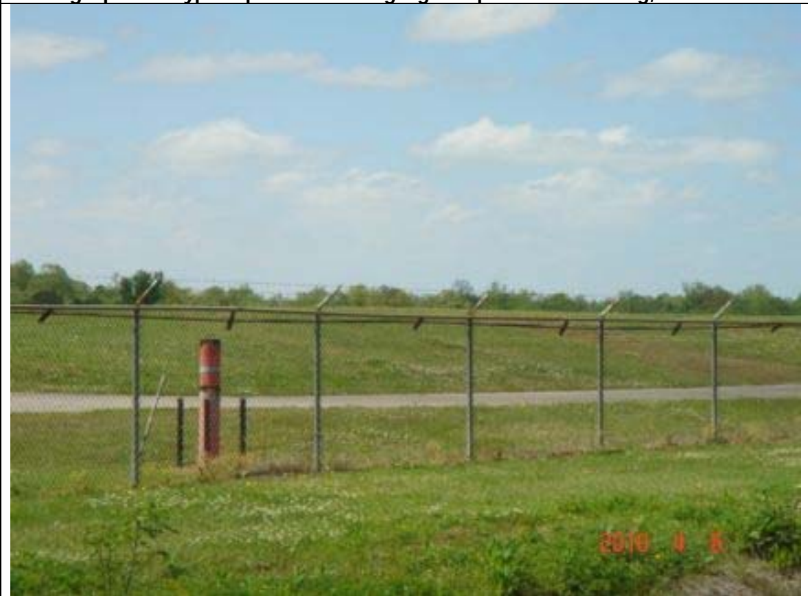
Photograph 4 – North Perimeter Fence, Brooklawn OU, South 4/6/10
