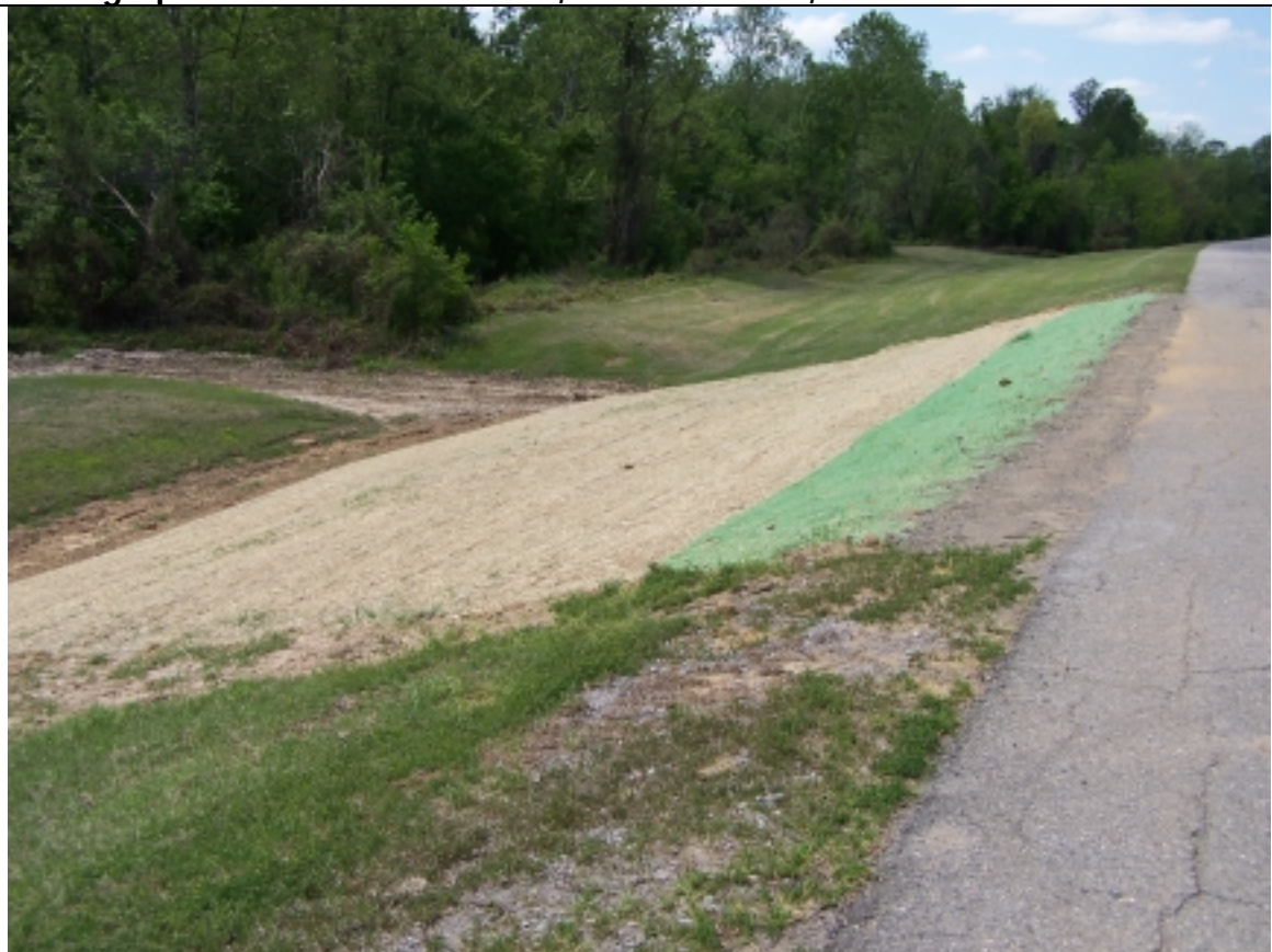
Photograph 10 – Repair on South Levee Road, Brooklawn OU, West 4/6/10
