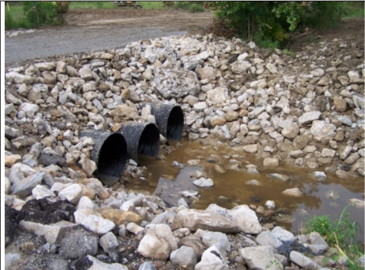
Photograph 29 – Bridge Repaired, Scenic OU, Southwest 6/3/10
