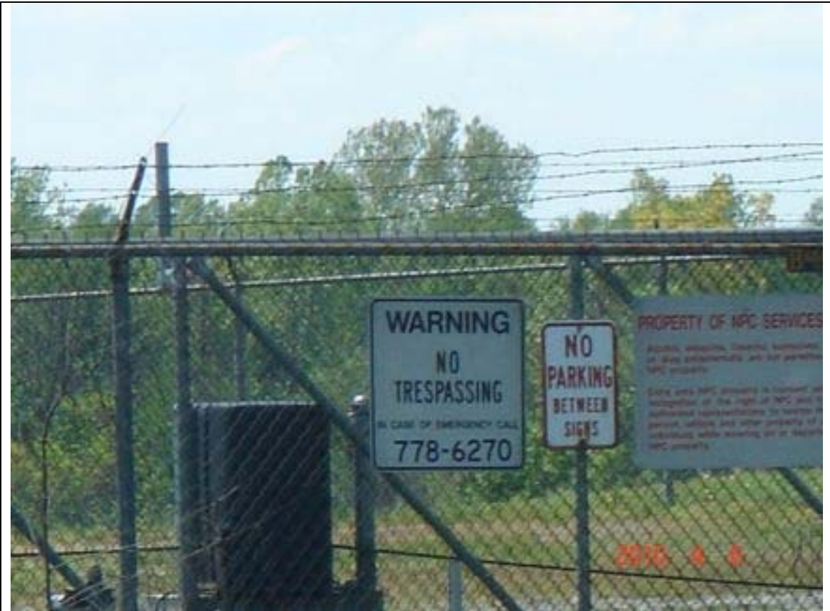
Photograph 3 – Typical posted warning sign on perimeter fencing, South 4/6/10
