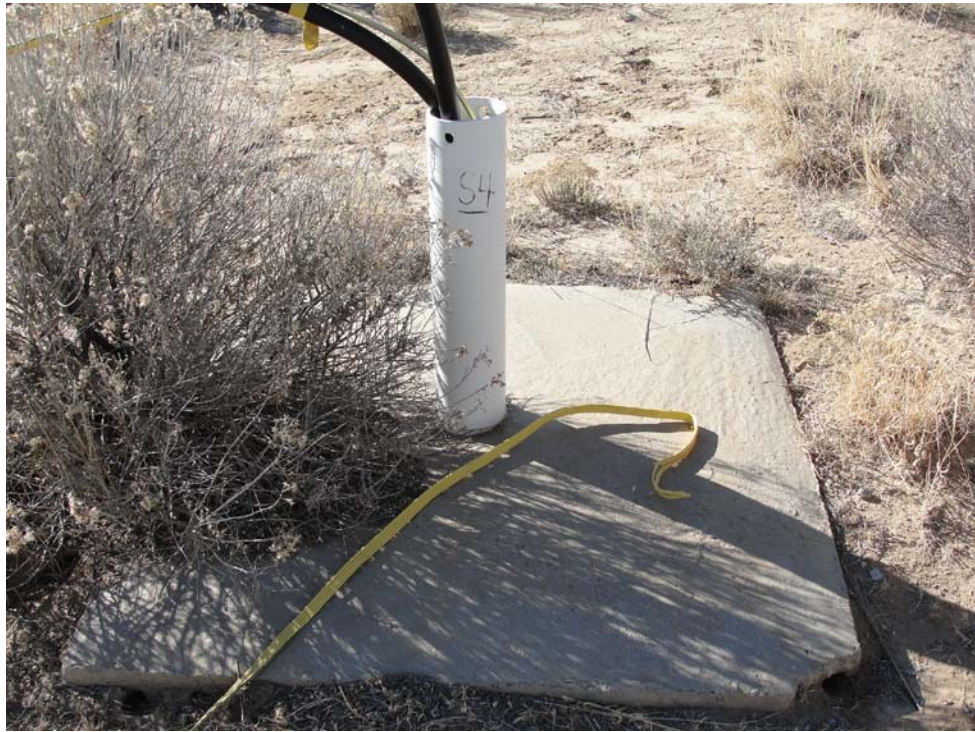
Photo 17: POC Well S4 on the west side of the large tailings pile.
