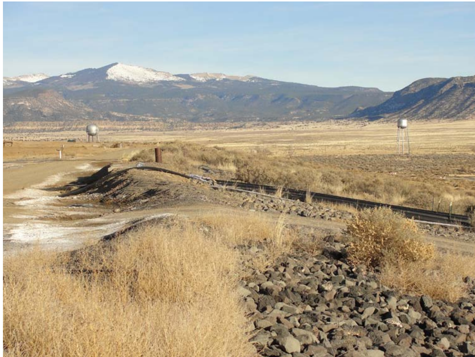
Photo 5: Roads leading up to (foreground) and on top of the large tailings pile. Piping on the opposite side of the road is used to convey collected groundwater to the RO treatment plant or to one of the evaporation ponds for disposal. Note the water towers marking the locations of the two former mill sites. View looking east.
