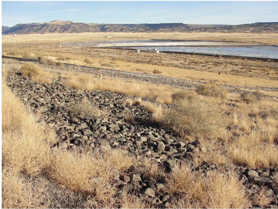
Photo 1: View of Evaporation Pond 1 (far left) and Evaporation Pond 2 from on top of the large tailings pile. Note the cobbles in the foreground used as a part of the erosion-protection cover on the large tailings pile. View looking southeast.
