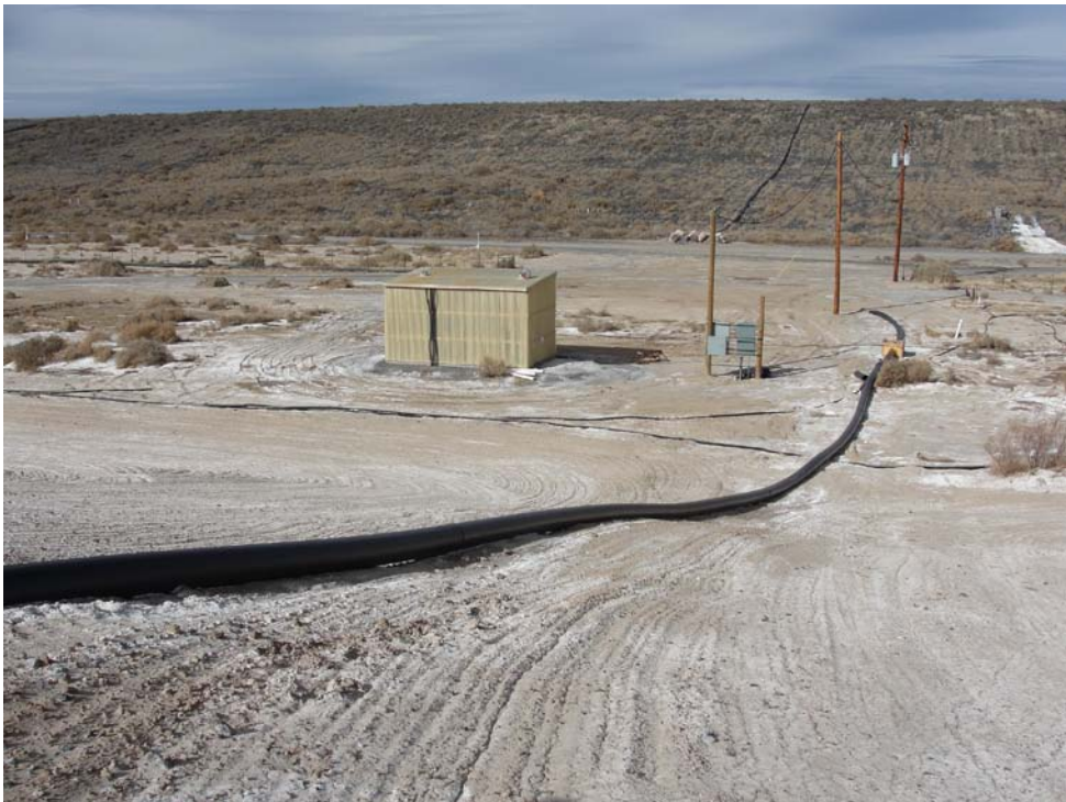
Photo 12: South side of the large tailings pile viewed from the south berm of Evaporation Pond 1. Extracted groundwater is pumped from the large tailings pile to the evaporation ponds using the piping in the center of the pictured. View looking north.
