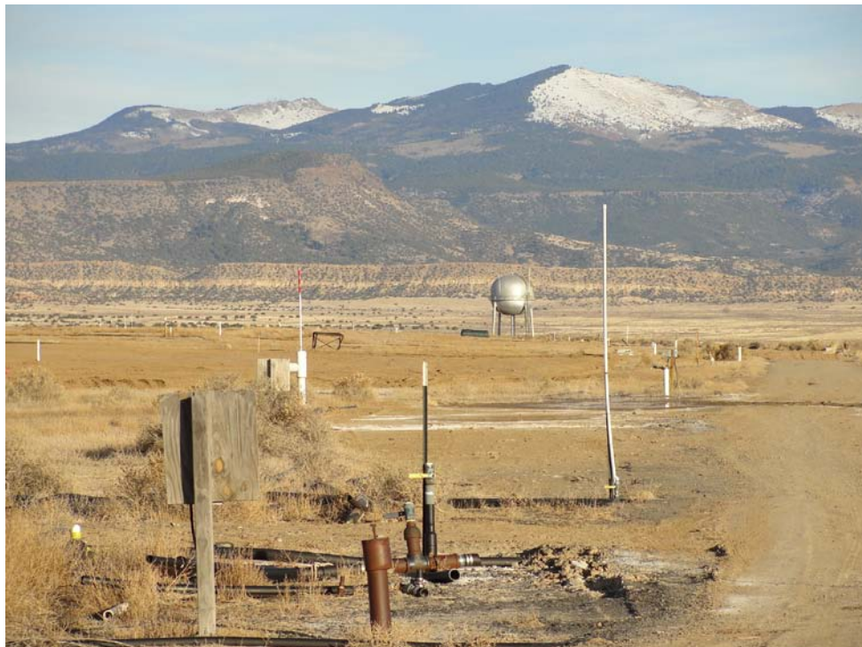
Photo 6: Extraction wells and piping on top of the large tailings pile. View looking east.
