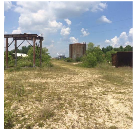
Above ground storage tank and remnants of former creosote site operations
