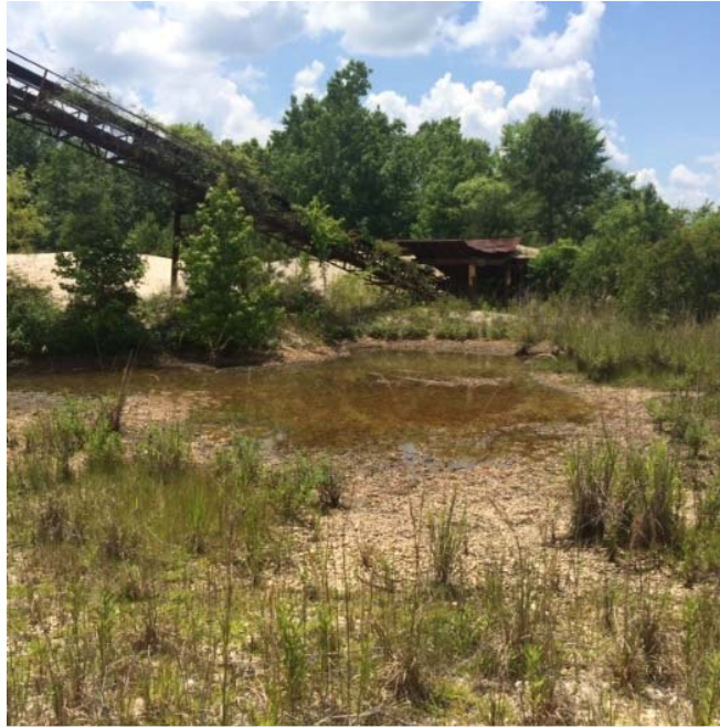
Remnants from former creosote site operations
