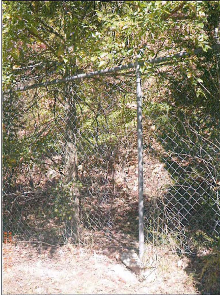
Photo 11: Breach in Perimeter Fencing On North Side
