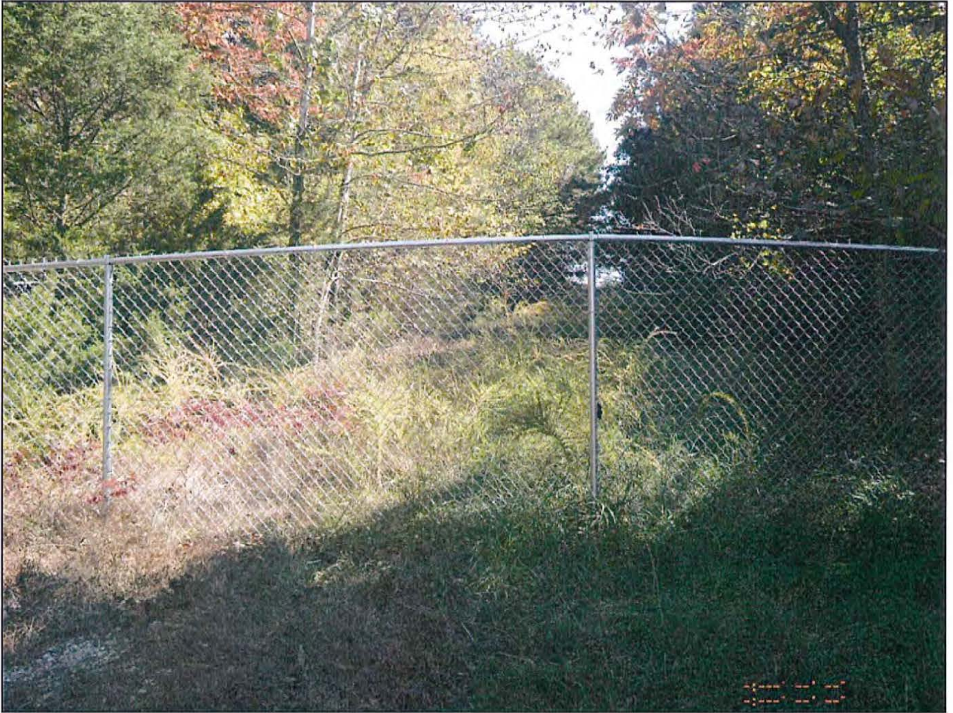
Photo 8: New Perimeter Fencing At East End
