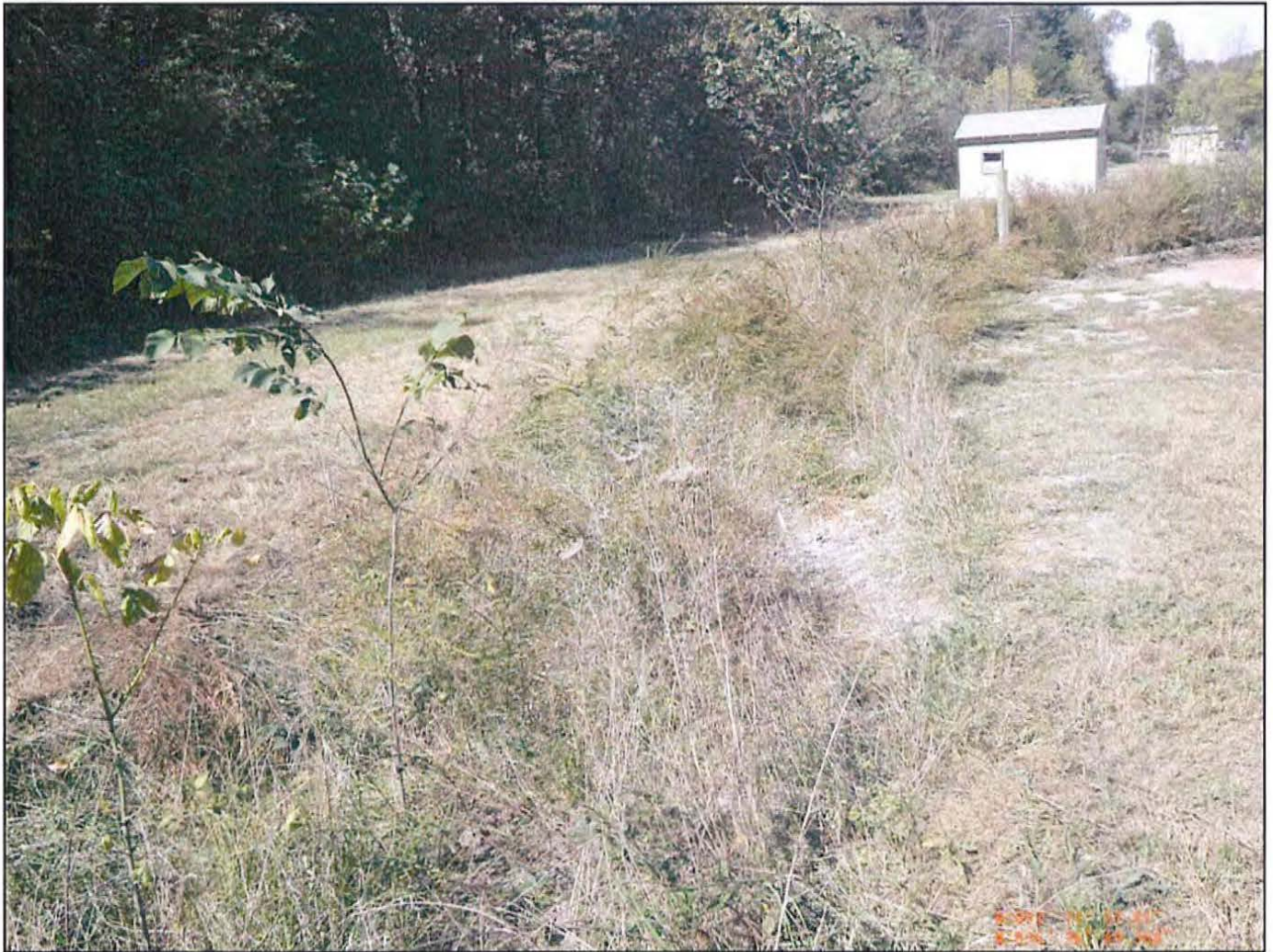
Photo 4: Site Stormwater Ditch - South
