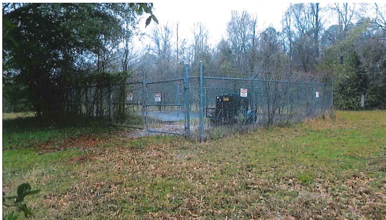
Staging area for DNAPL collection operations
