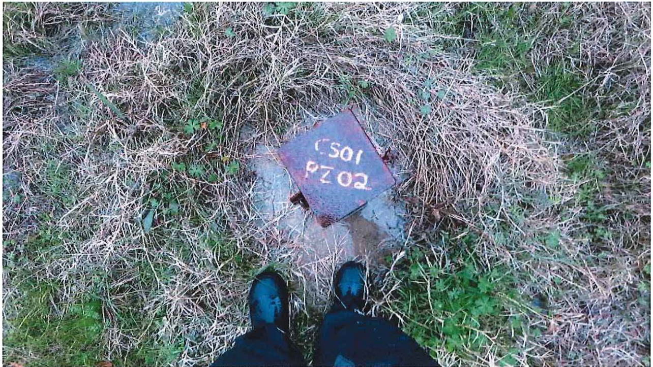
DNAPL recovery system piezometer
