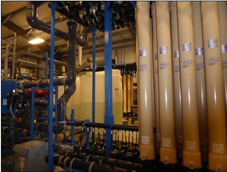
New microfiltration units within the RO treatment system facility
