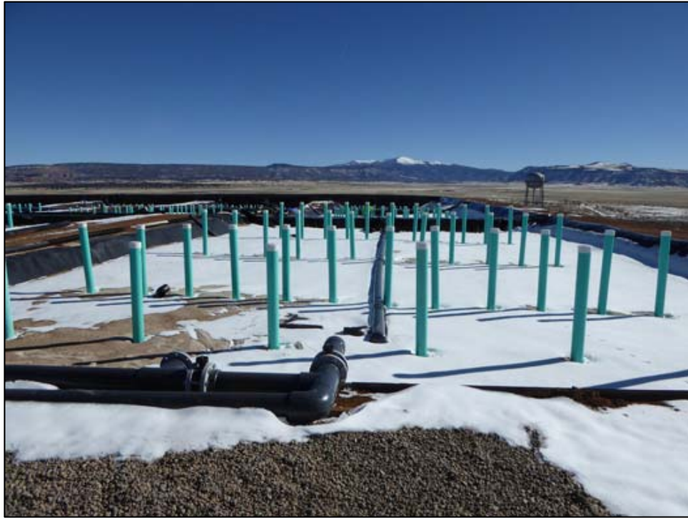
Full-scale zeolite treatment system vents
