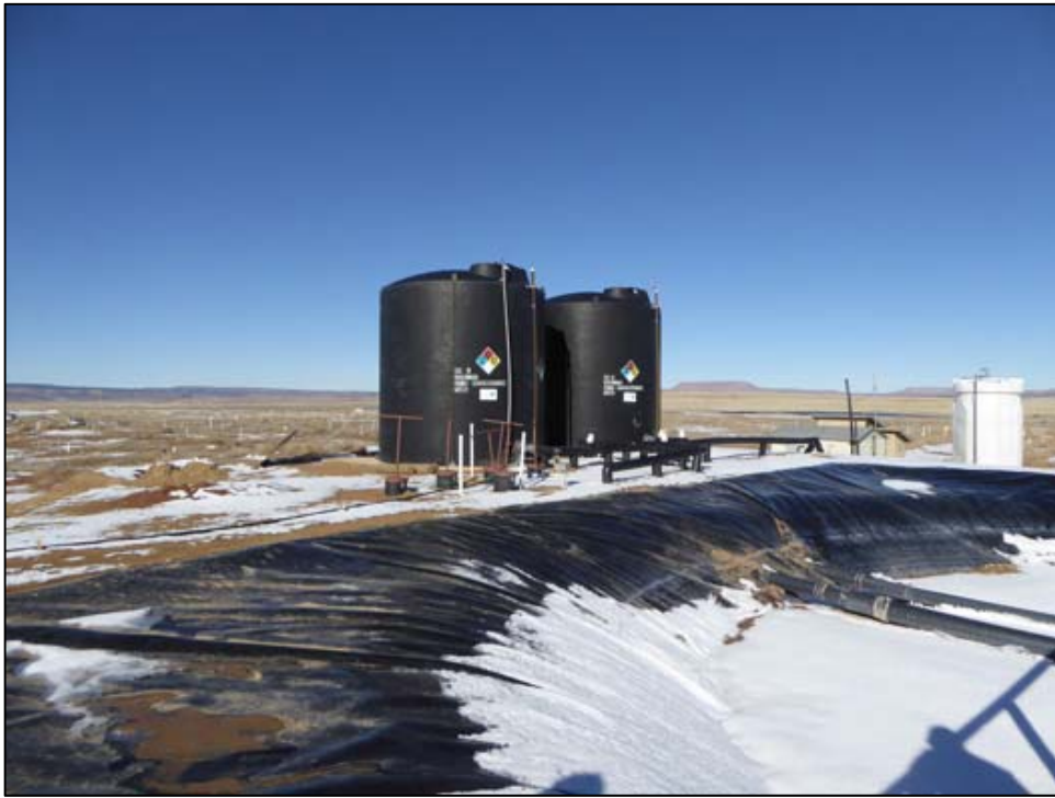
Pilot zeolite treatment system tanks
