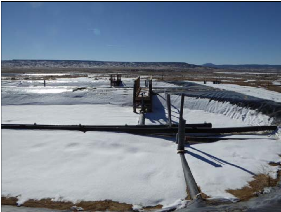
Pits and piping for the pilot zeolite treatment system
