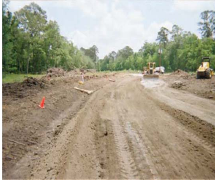
Cutting of subgrade and ditch along CR126 (2009)
