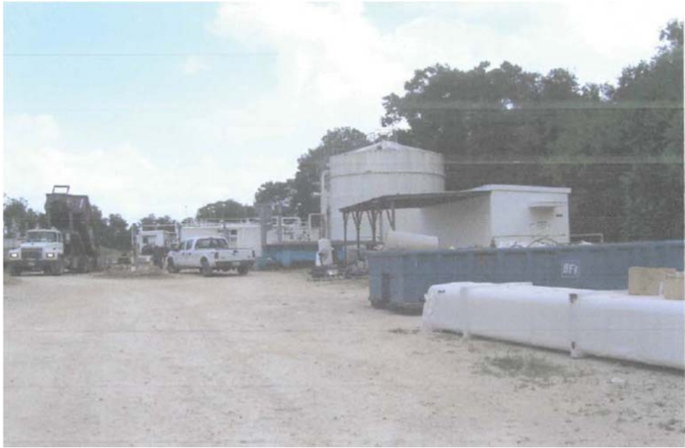
Wastewater treatment plant at the MWA (2005)
