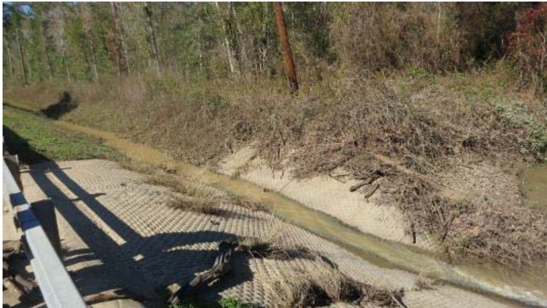
Culvert running parallel to CR126 discharging to Turtle Bayou (far right)
