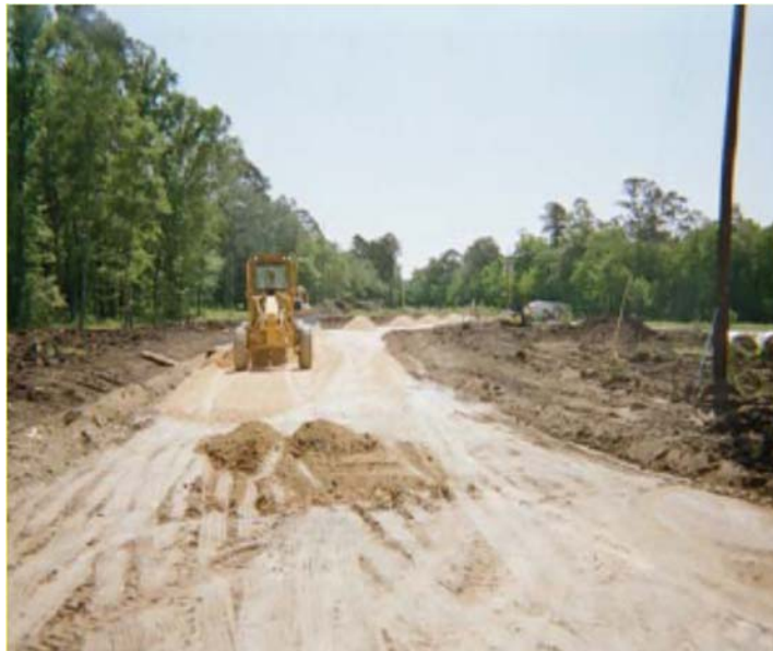
Adding aggregate to subgrade along CR126 (2009)
