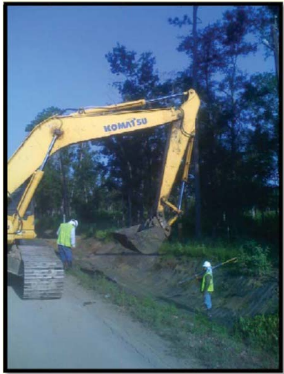
Construction of new ditches along CR126 (2010)
