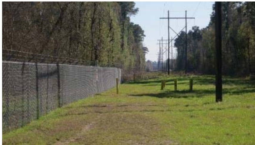
Secured entrance into the utility easement areas (the EA)
