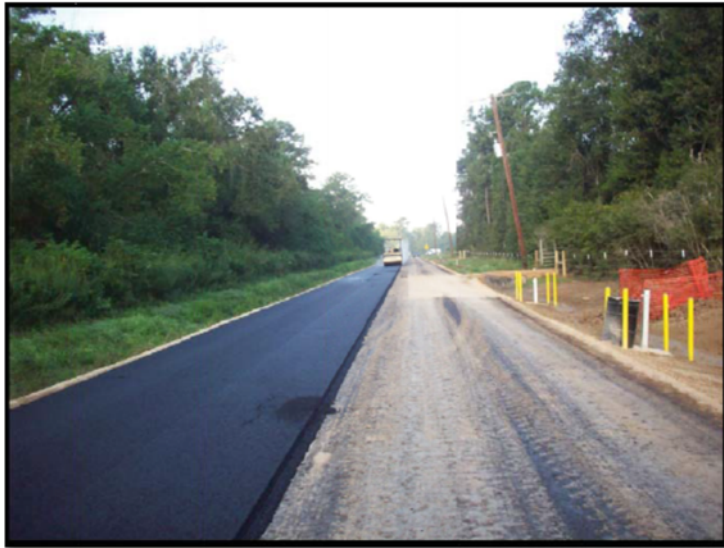
Asphalt paving of CR126 (2010)
