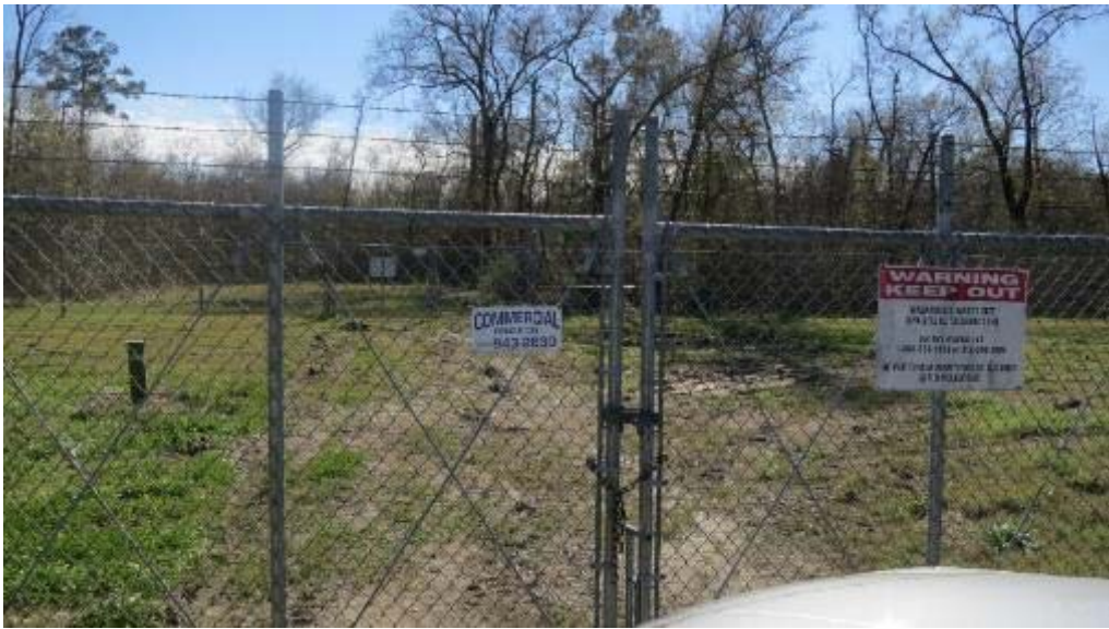
Gated and locked entrance to the WRA, looking south
