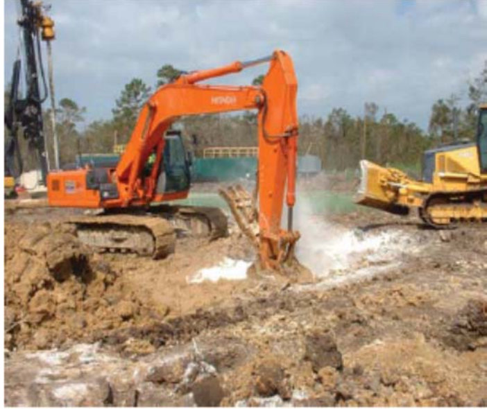
Mixing of treated soil with lime (2009)
