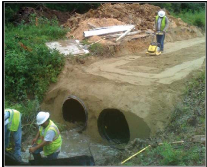
Installation of new ditch culverts (2010)
