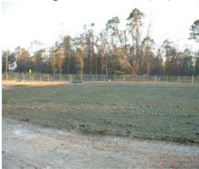
FWRA soil treatment area graded and hydroseeded (2009)
