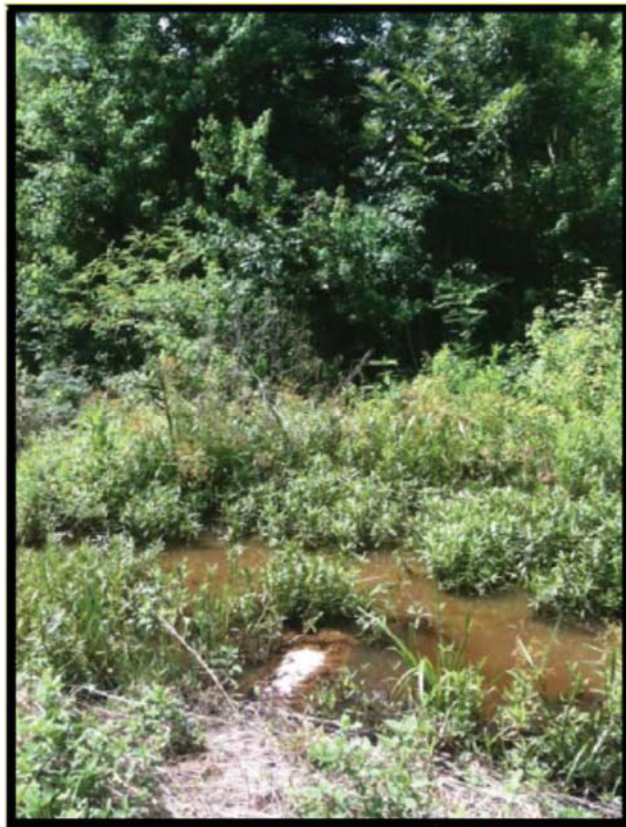
CR126 Ditch prior to improvements (2010)
